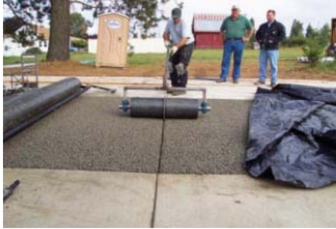
Figure 2.15: Use of a Rolling Joint Tool
