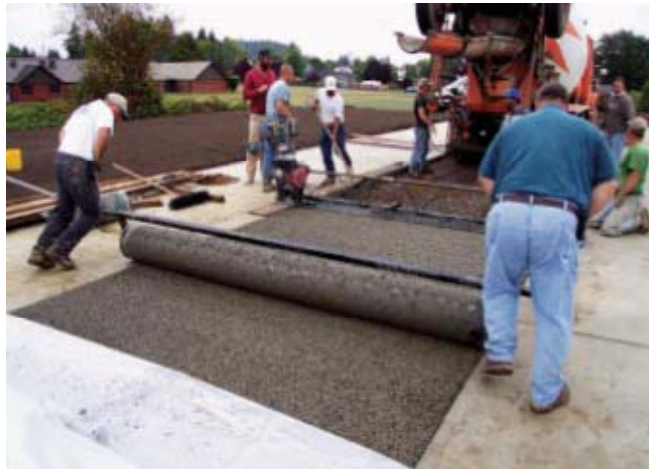
Figure 2.14: Use of a Steel Roller
