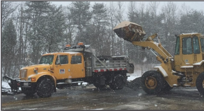
Clearing snow-covered roadways
