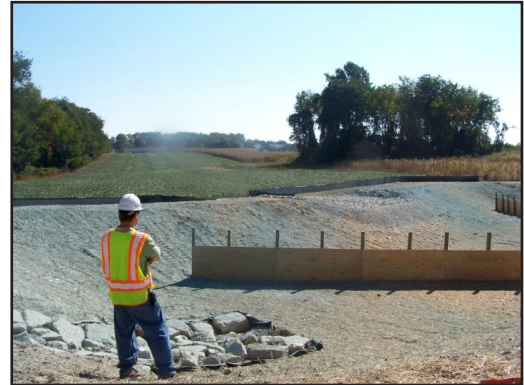
Inspection of sediment basin during construction
