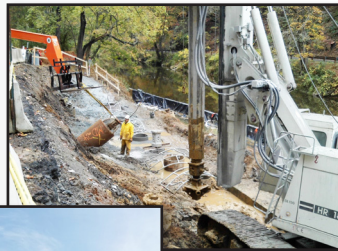
MD 24 road/slope repair
