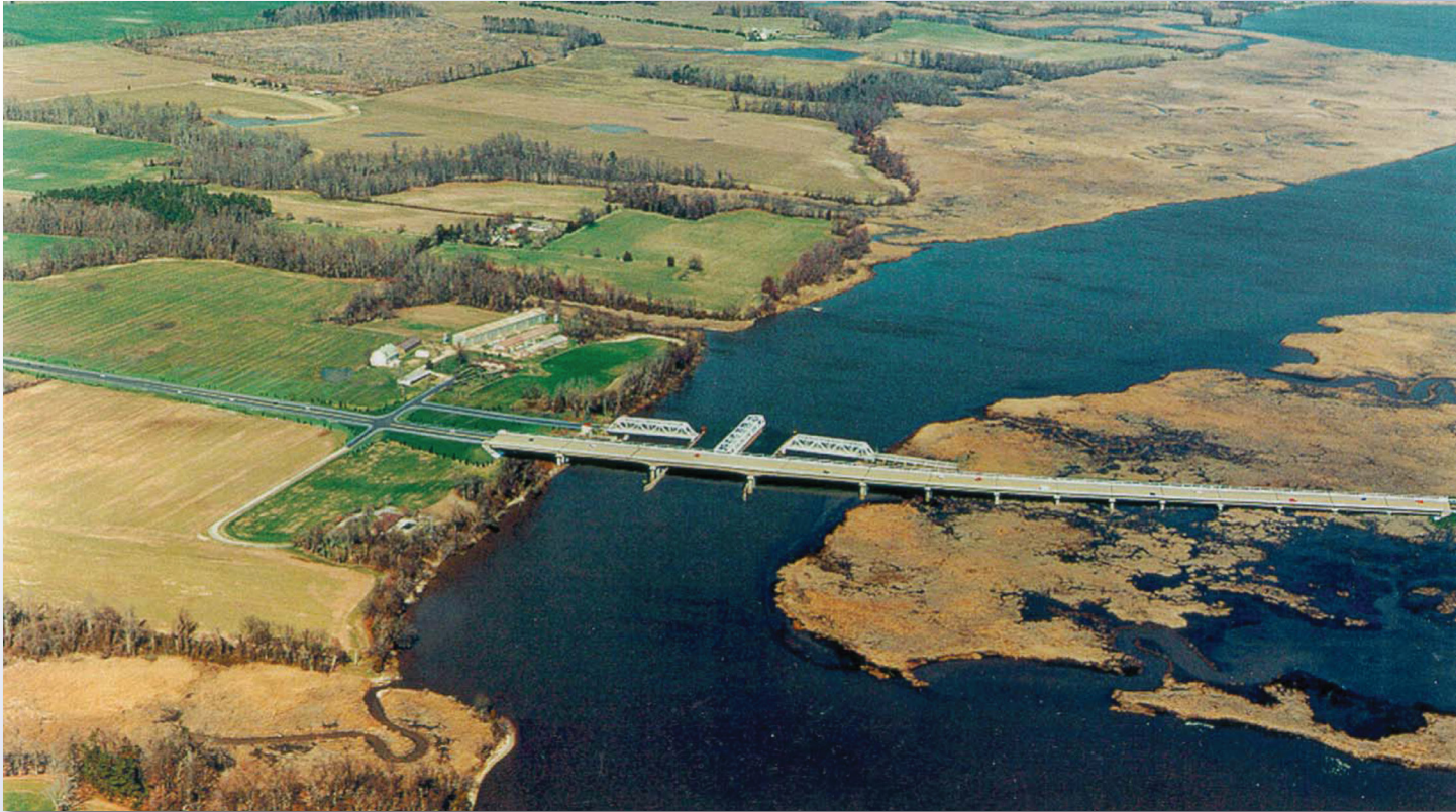
New Bridge with Old Bridge in Open Position
