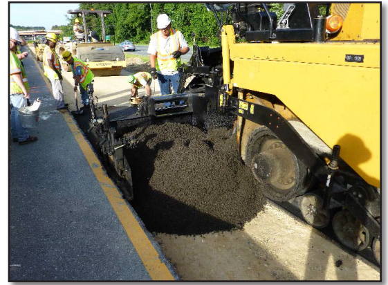
Workers applying a test strip of recycled base material to northbound US 29
