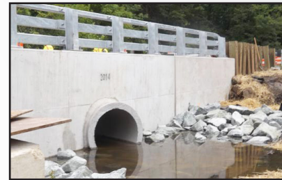
MD 648 bridge over Cattail Creek work in progress
