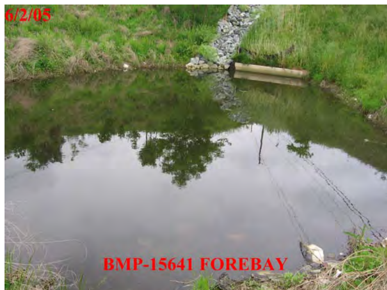
Example of BMP Inspection Digital Photo
