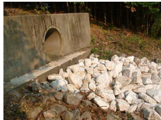
Figure 3-3 SWM Pond Outfall Stabilization at BMP 13347
