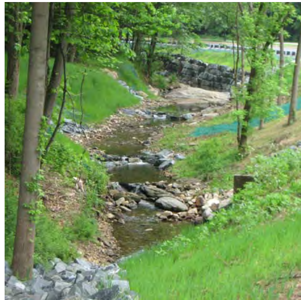
Construction on Towson Run Stream Stabilization was Completed in 2007
