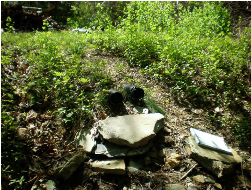
Laundry wastewater connection to natural stream channel.
