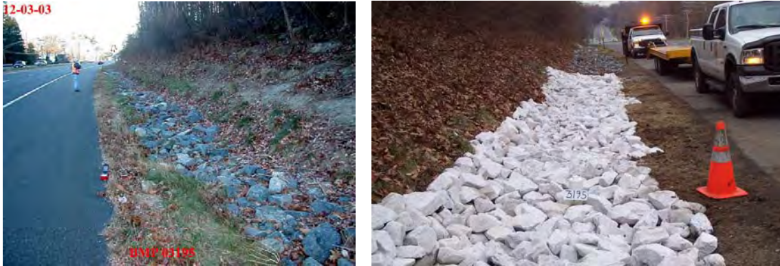
Figure 3-4 Installation of Infiltration Trench Monitoring Well and Media Replacement for BMP 3195 in Baltimore County
