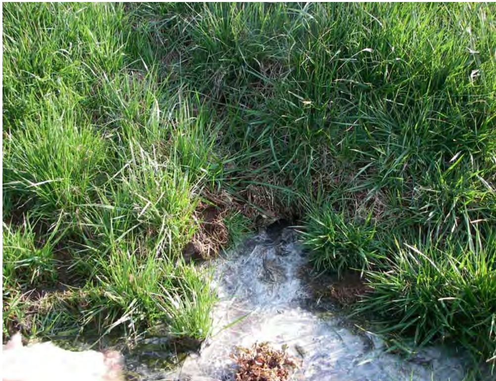
Wastewater discharge in front of 12751 Creagerstown Road.
