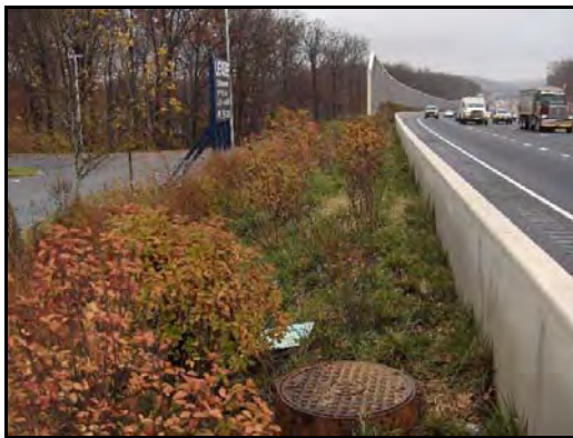
Instrumentation at I-83 Underground Storage Facility Sites
