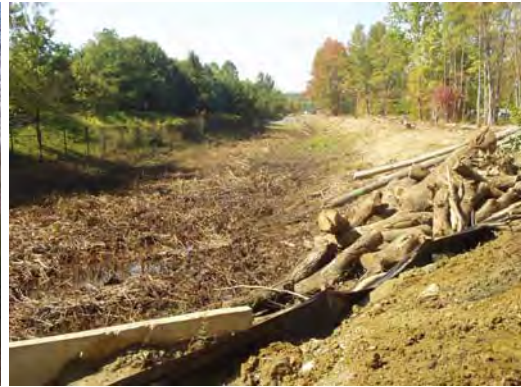
During the construction
