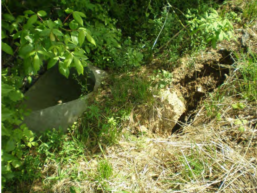
Additional view of end separation from pipe.
