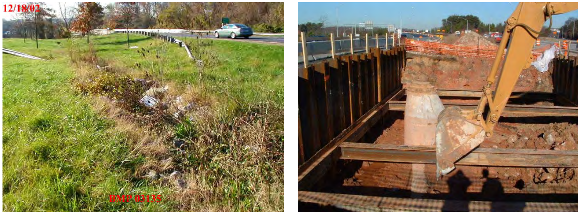
Figure 3-4 Installation of Infiltration Trench Monitoring Well and Media Replacement for BMP 3195 in Baltimore County
