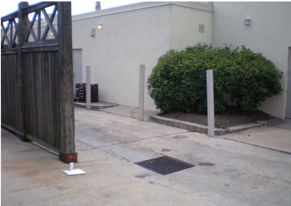
View of inlet where illicit flow was found.
