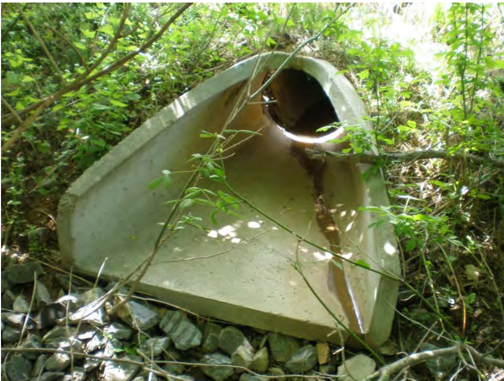
Downstream SHA end section is separated from 24" pipe.
