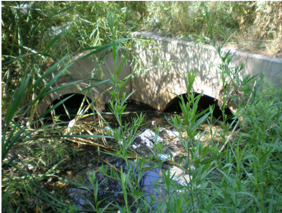
View of outfall #1304315.001.
