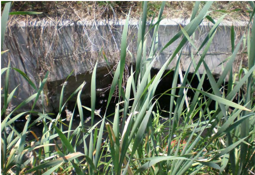
View of outfall #1300102.001.
