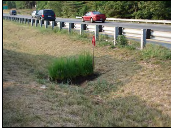
Native Grass Check Dam at SHA Swale
