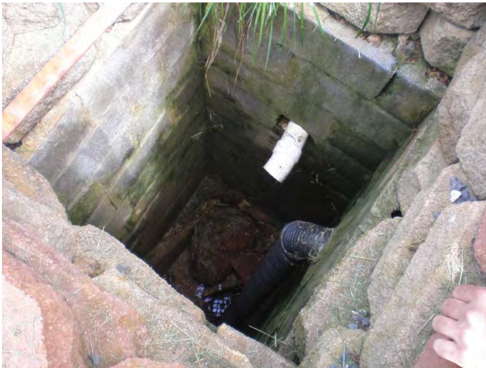
Illicit connections within SHA inlet.
