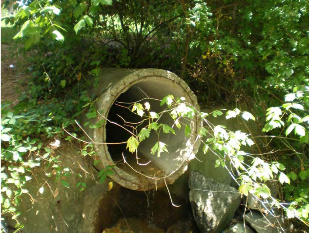
View of outfall #1500716.001
