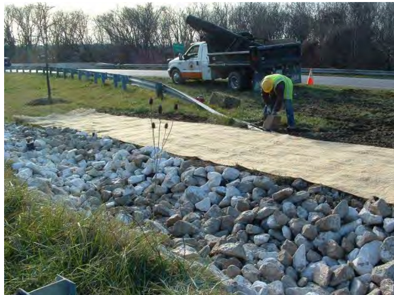
Figure 3-5 Installation of Infiltration Trench Monitoring Well and Media Replacement before, during and after for BMP 3135 in Baltimore County
