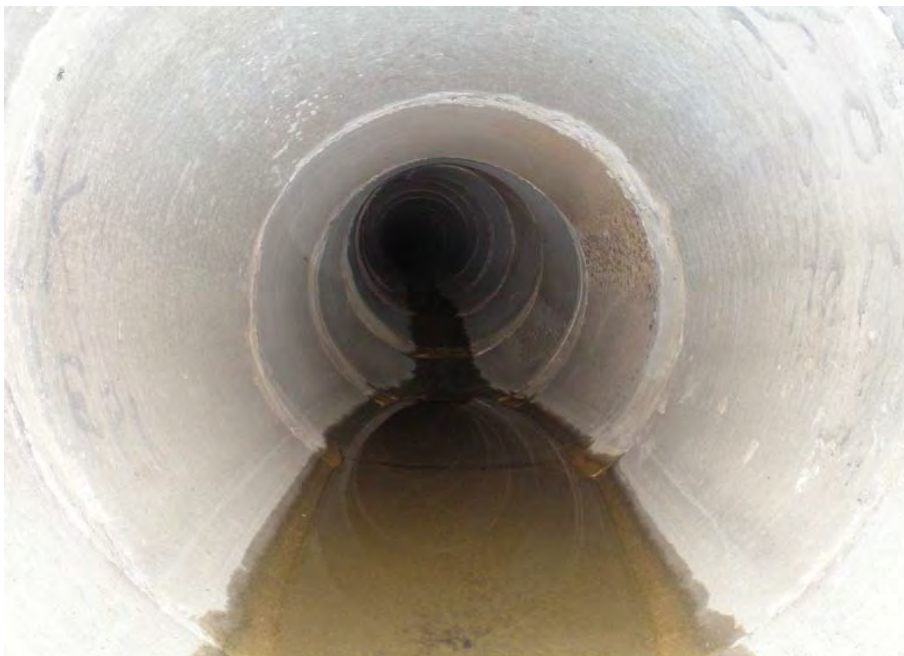
View of pipe
