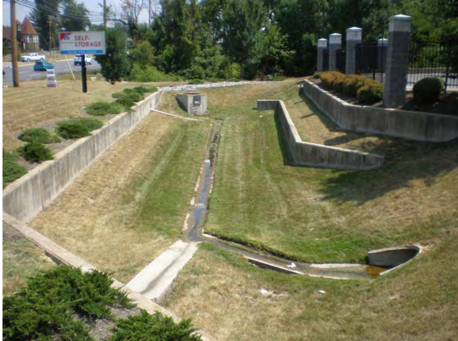
SWM facility in front of Self Storage facility on Kit Kat Road. showing seepage
