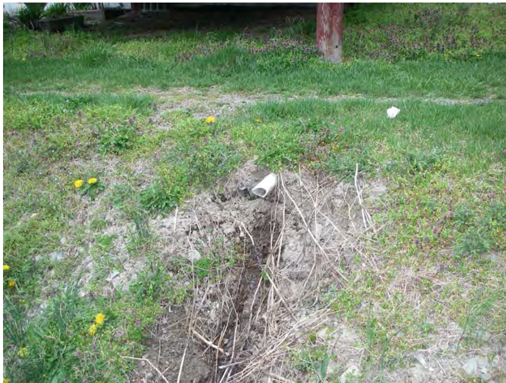
Illicit connection at 12758 New Windsor Road.
