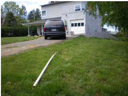
An Illicit Connection at MD 79 in Frederick County
