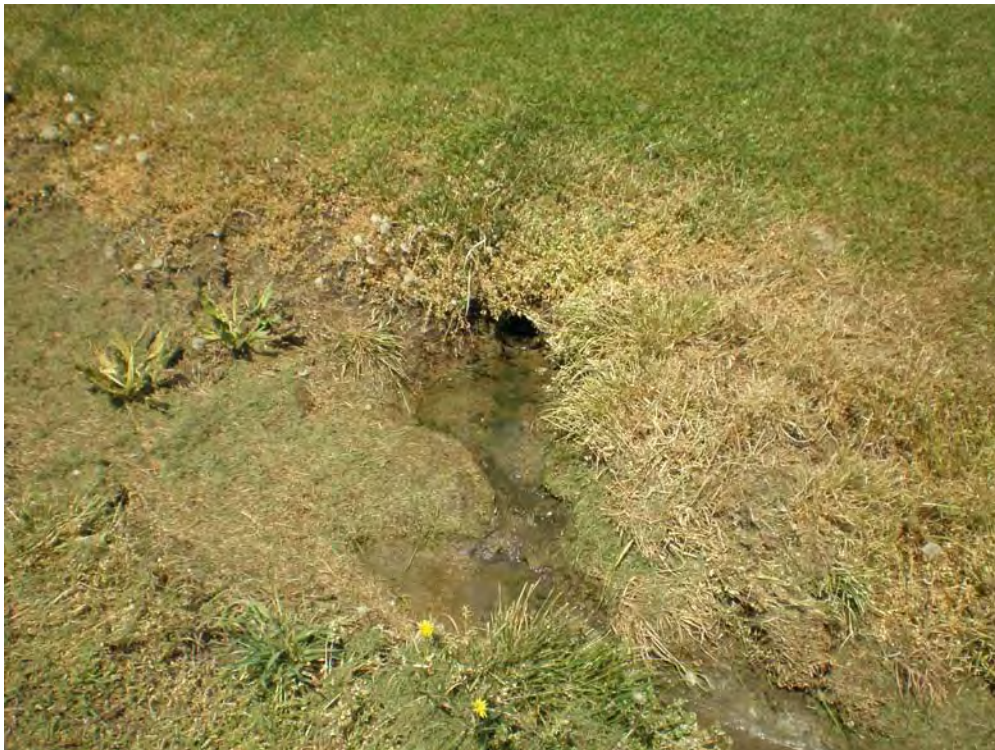
Wastewater discharge at 3302 Burgee Drive.
