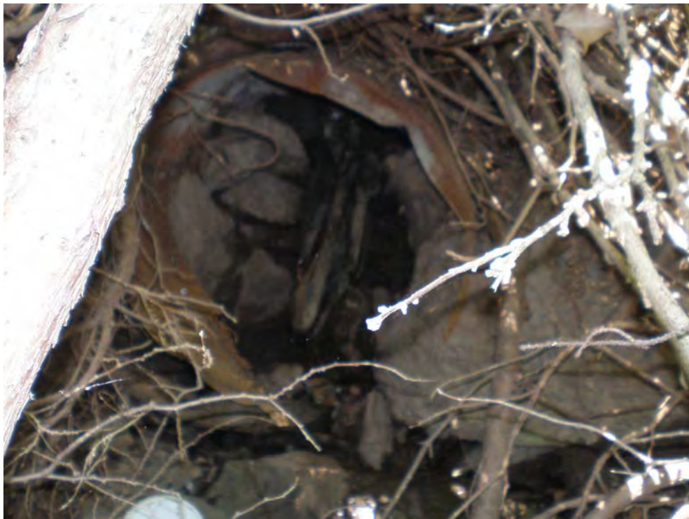
Downstream SHA outfall structure.
