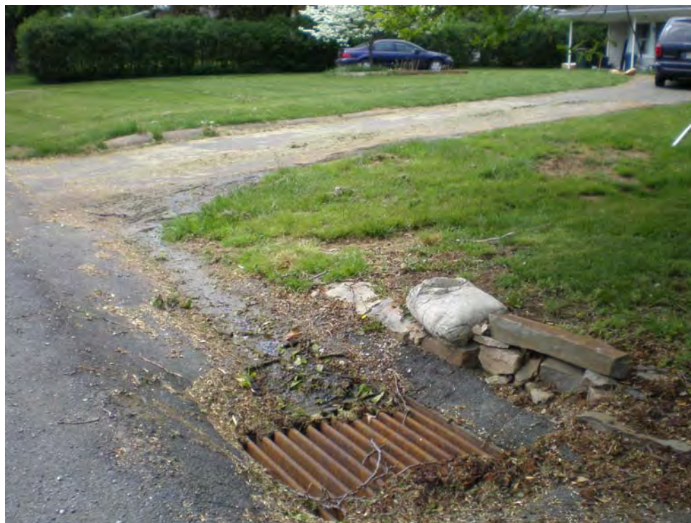
Indication of illicit flow at 3608 Petersville Road.
