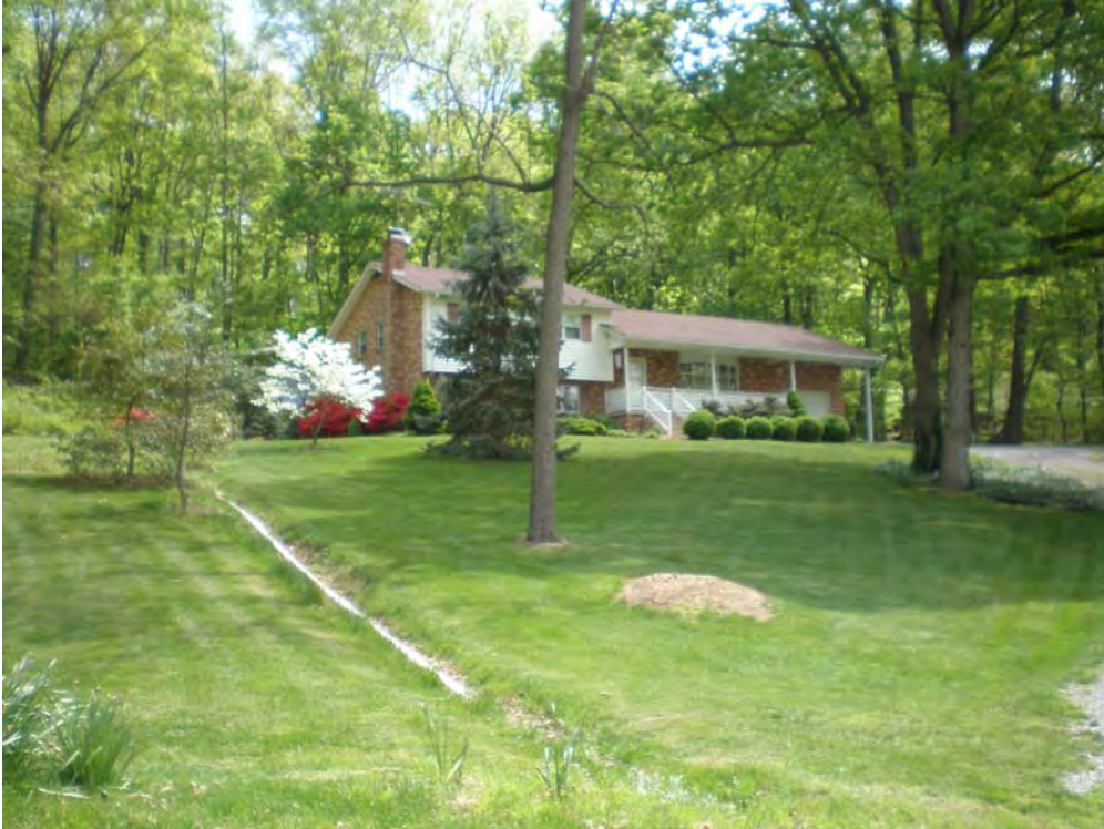
3884 Point of Rocks Road. PVC continues encircling house in backyard.
