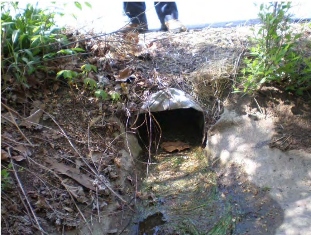
Downstream SHA outfall structure #1020311.001.
