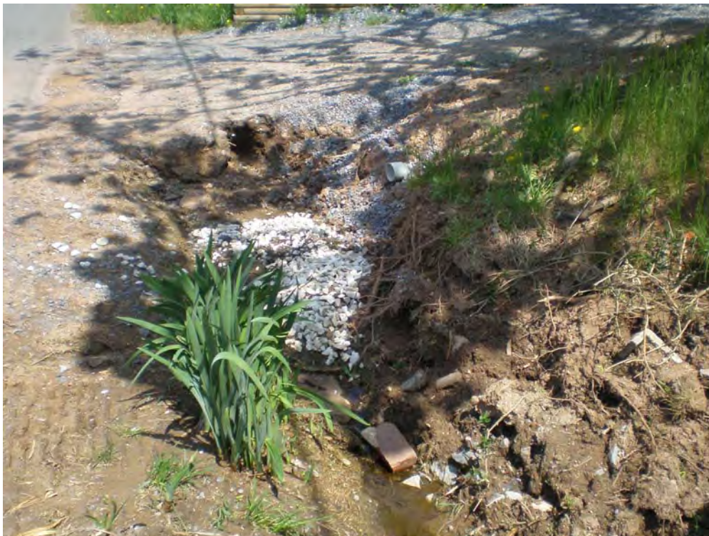
Sewage discharge at 6101 Jefferson Pike. Terra cotta pipe has been replaced with perforated PVC by the homeowner.
