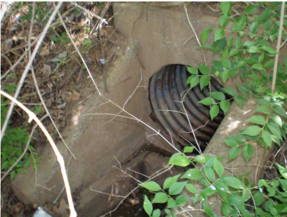
Downstream SHA outfall structure.
