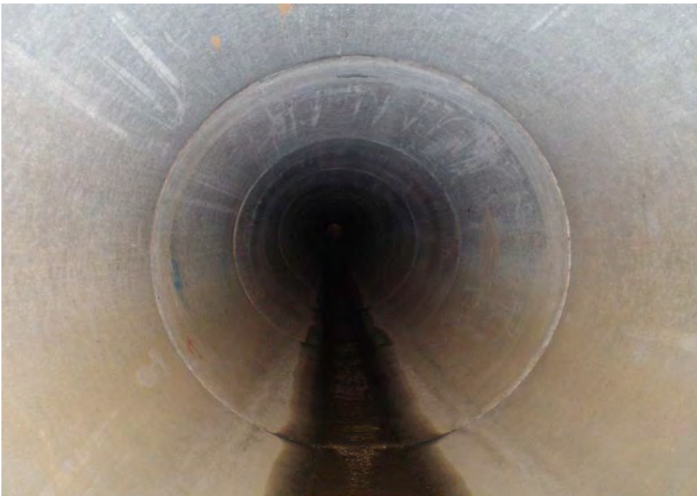
View inside pipe.
