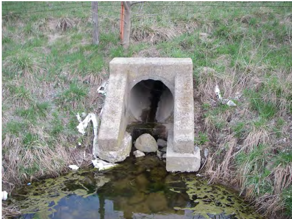
Downstream SHA outfall structure.
