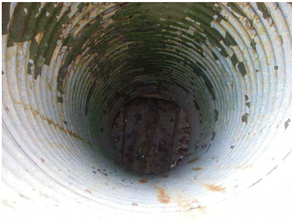
View inside inlet leads to 9001 Hollow Road.
