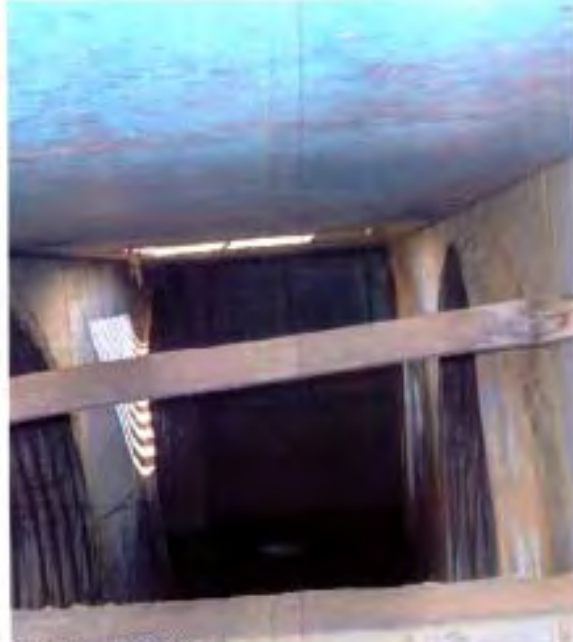
Figure 4. View of centre inlet and storage pipes from control structure of BMP16133
