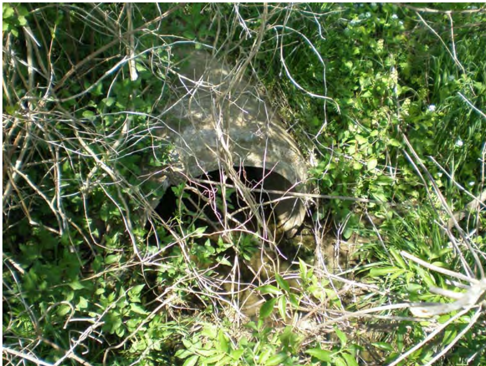
Downstream SHA outfall structure #1001748.001.
