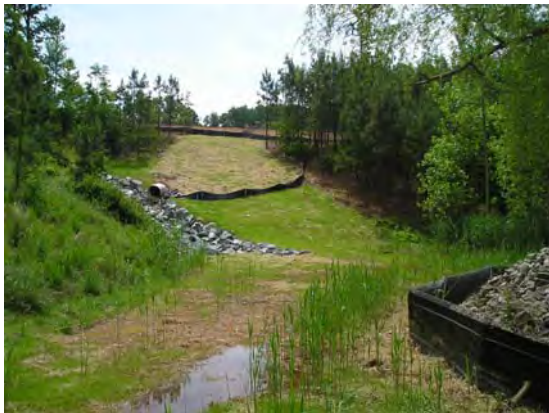
Figure 3-2 SWM Pond Major Maintenance
