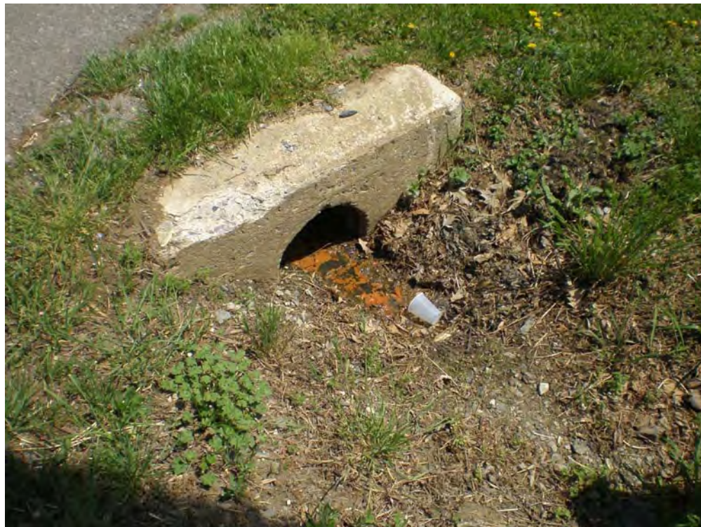
Wastewater discharge at SHA culvert inflow point.
