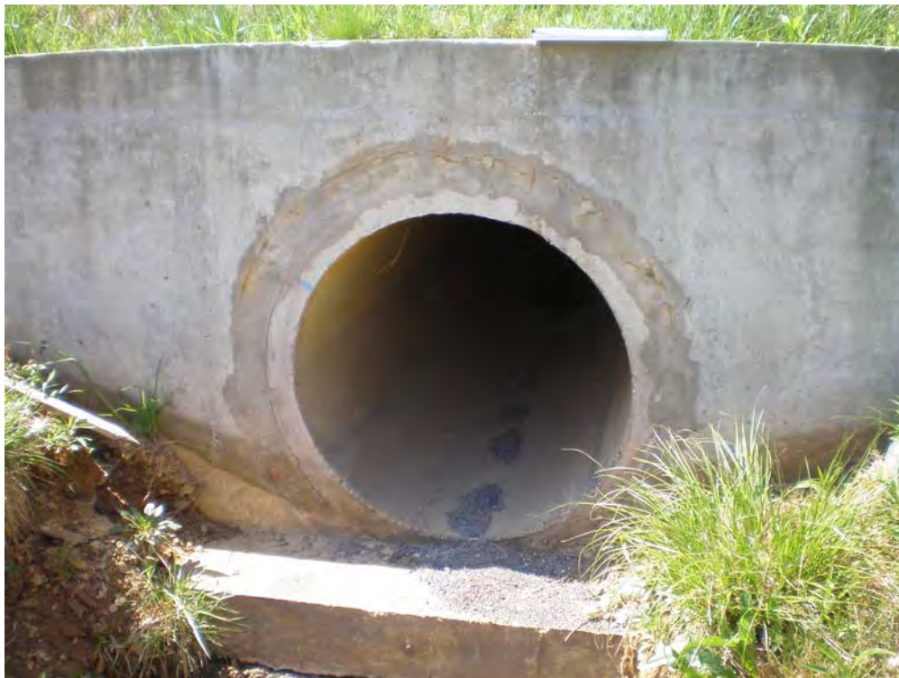
Downstream outfall structure #1020340.035 at SWM pond.
