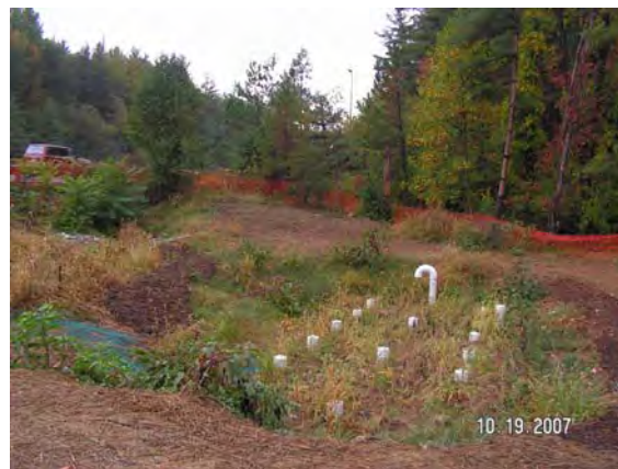
Sand Filter after construction
