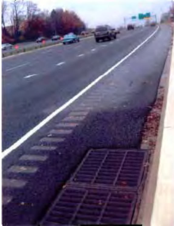
Figure 6. Inlet along I-83 NB
