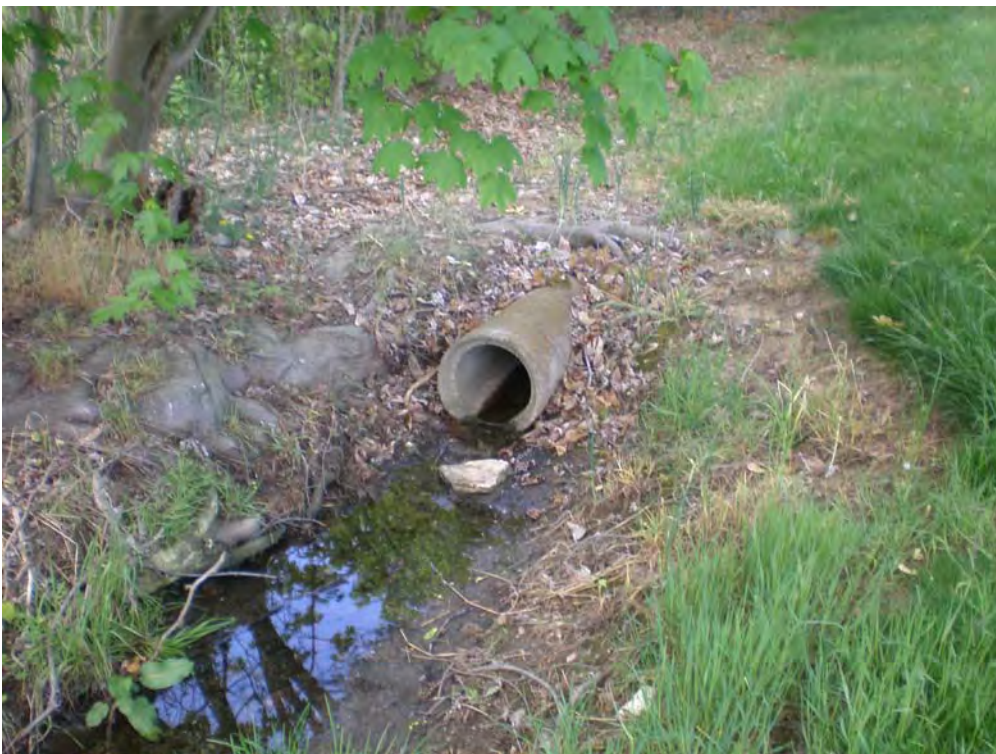
Downstream SHA outfall structure.
