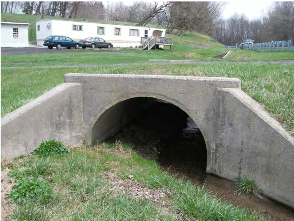
Downstream SHA outfall structure.
