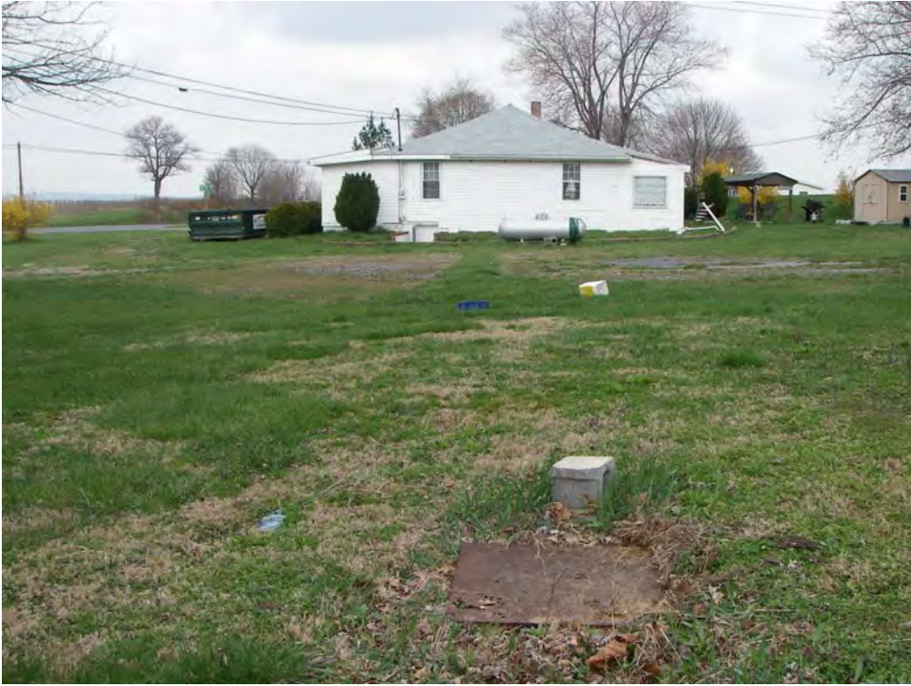
Septic field area and residence at 9001 Hollow Road.
