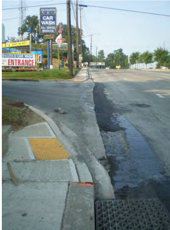
Irrigation from Touch Less II trickles into a SHA inlet - not washwater.
