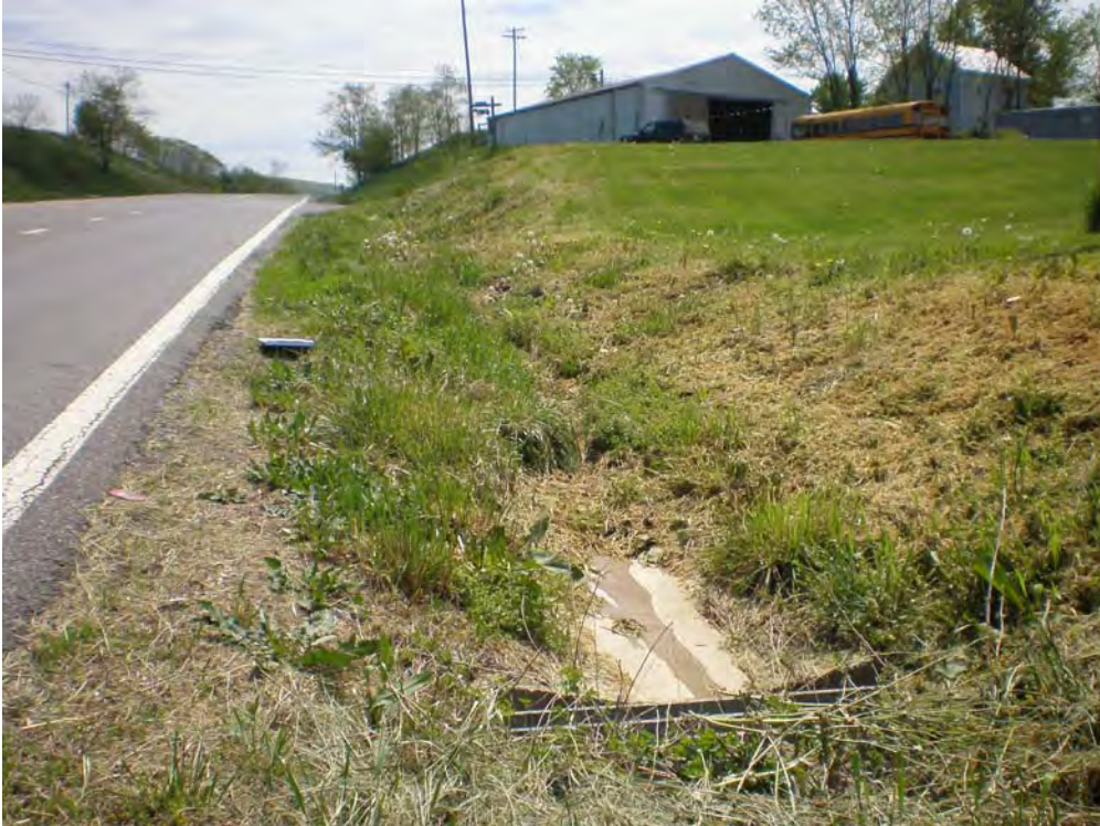
Indications of recent flow at 3253 Point of Rocks Road.
