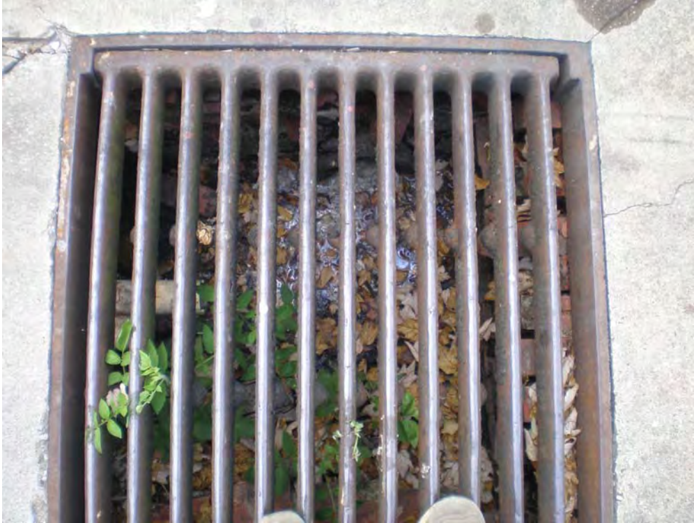
View of foamy discharge inside inlet in rear of Holiday Inn.
