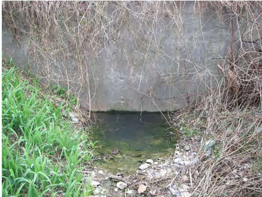
Downstream SHA outfall structure, submerged.
