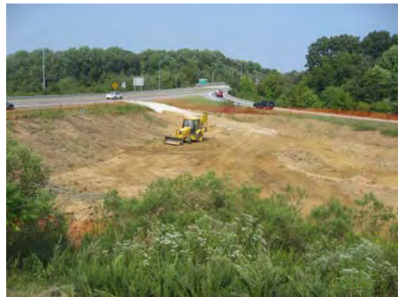
During construction of Micropool Extended Detention Pond
