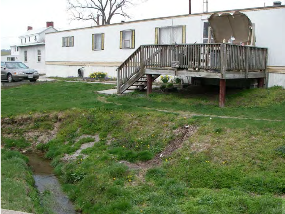
12758 New Windsor Road. PVC pipe connects directly to natural stream channel.
