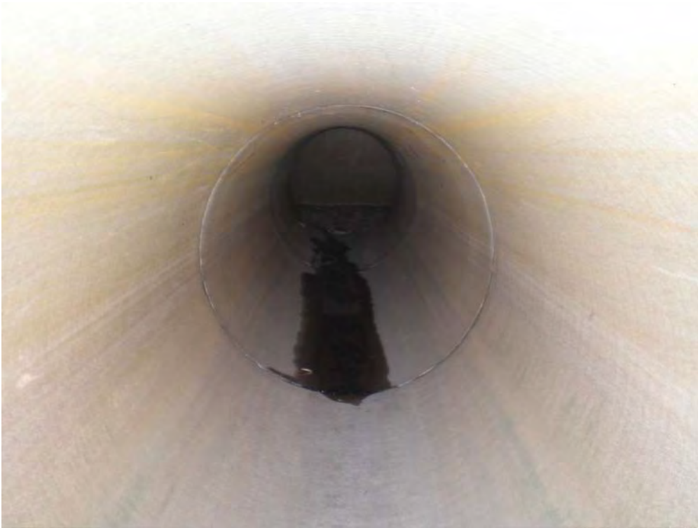
Illicit flow falls through pipe joints before discharging into SWM pond.
