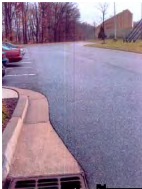
Figure 7. Access point from Timonium Business Park, Timonium two
