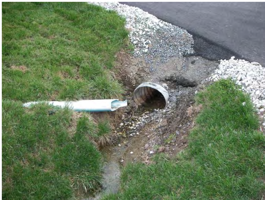
Illicit connection at driveway culvert (outfall point shown). 9303 Woodsboro Road.
