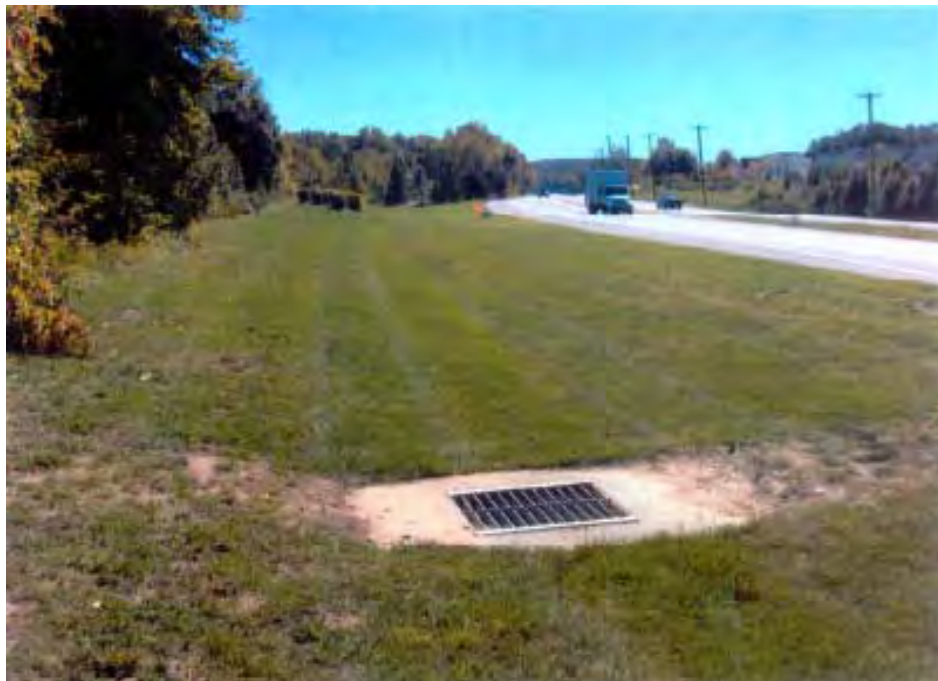
Figure 3. Inlet at centre of BMP16133
