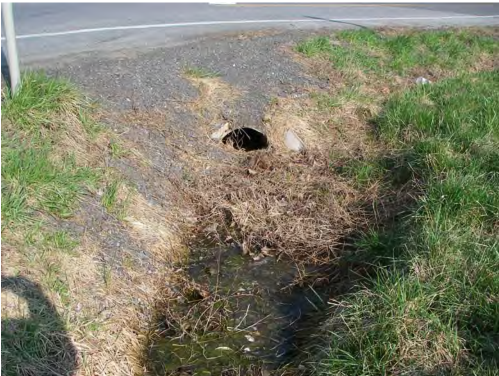
SHA outfall structure downstream of illicit connection.
