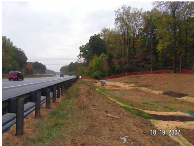
Construction of pocket wetland
