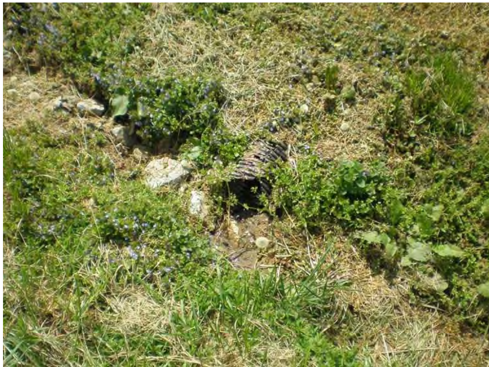
Illicit connection in front of farm property at 3253 Point of Rocks Road.
