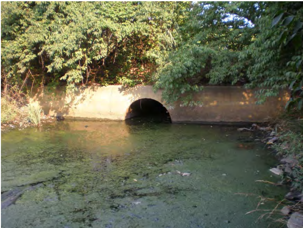
Rancid smelling plunge pool at downstream outfall.
