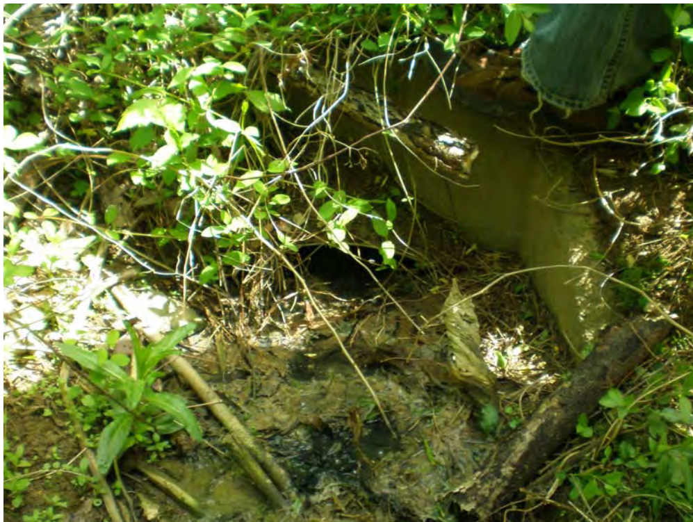
Downstream SHA outfall structure nearly submerged.
