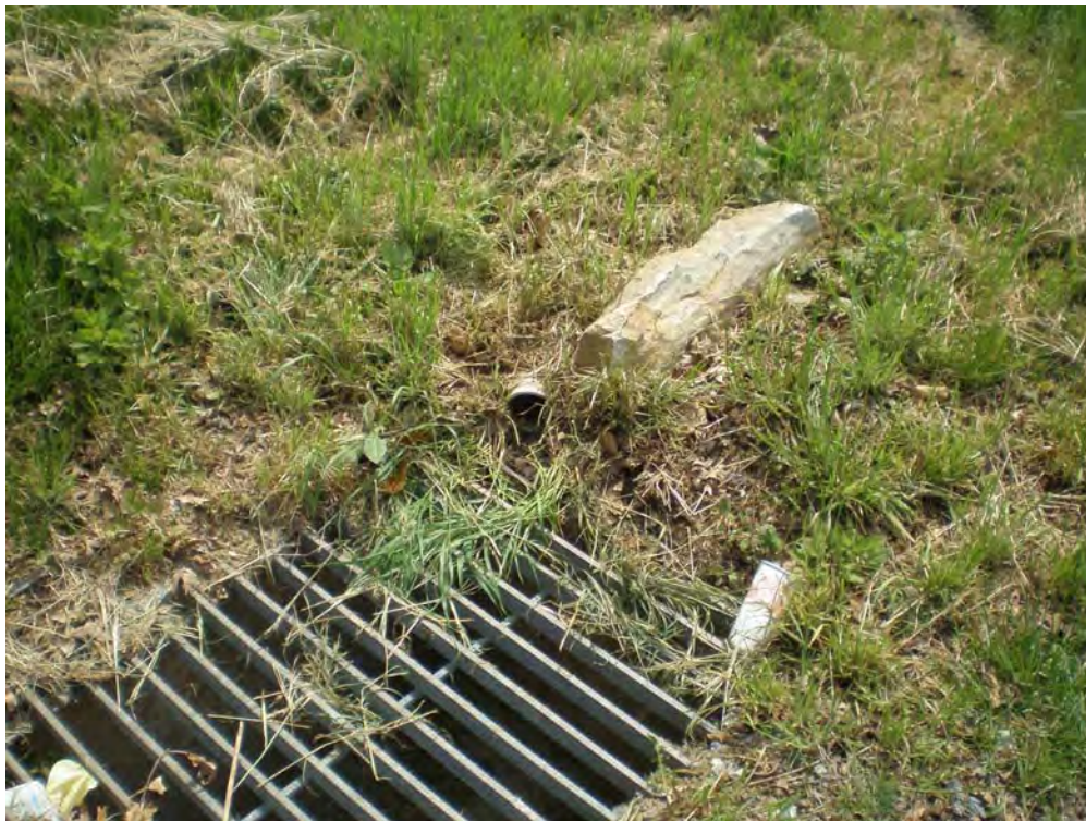
Connection from 3884 Point of Rocks Road.
