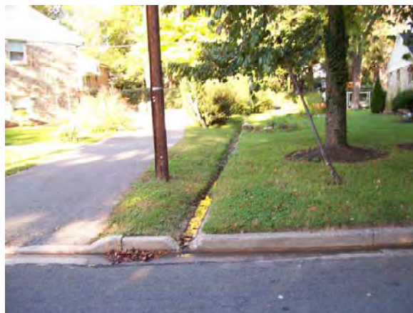
Illicit Discharge with Presence of Detergents and Ammonia discovered in Baltimore County
