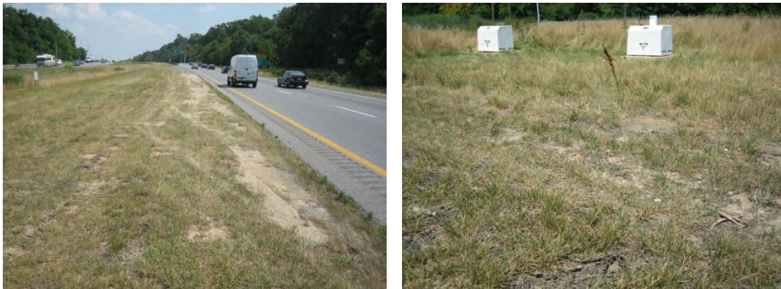
Figure 2. Bare spots on pretreatment area of MDE swale.
