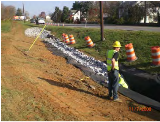
Figure 3-6 Infiltration Trench 020193 In-Kind Replacement
