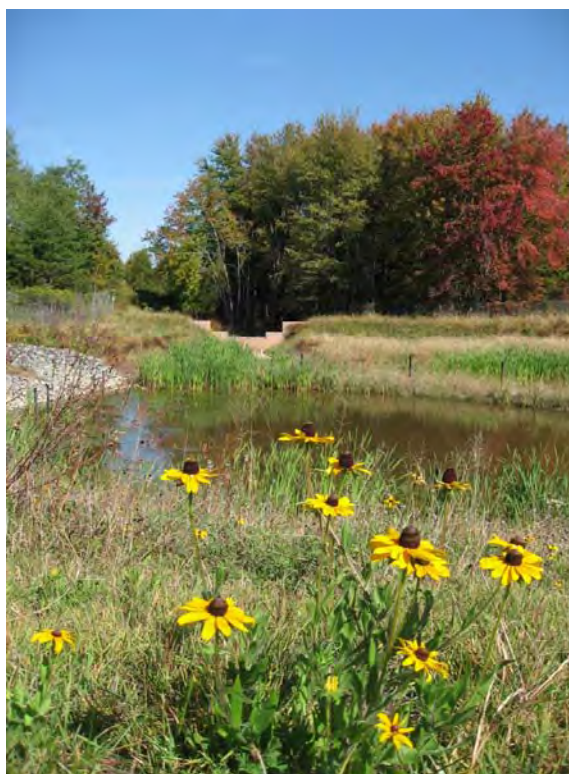
Figure 3-12 Reconstruction of Failed Infiltration Basin at MD 100 into Micro-pool Extended Detention Pond (BMP 020111)
