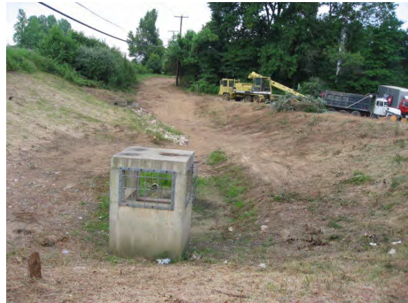
Figure 3-3 Inflow Channel Stabilization (BMP130292) - during construction
