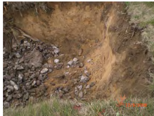
Figure 3-5 Excavation of Infiltration Trench 020191
