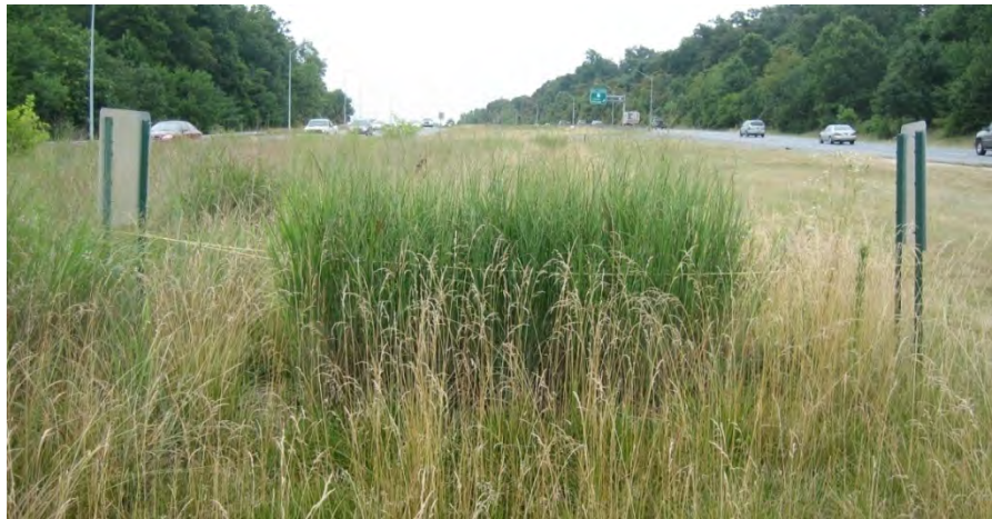
Figure 1-6 Native Grass Check Dams at Study Swale
