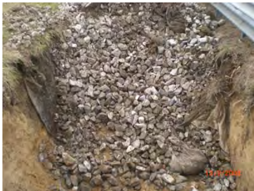
Figure 3-5 Excavation of Infiltration Trench 020191
