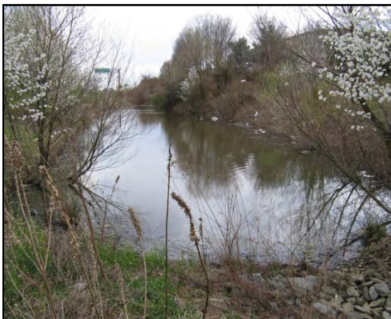
View of BMP 130348 at Outflow Point – Failed Infiltration Basin Currently Monitored
