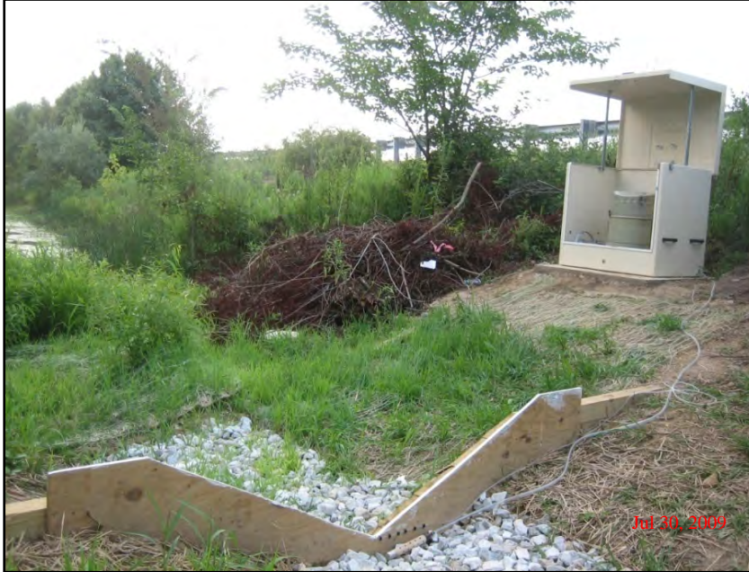
Figure 6. Photo showing sampler and weir installed at the study site.
