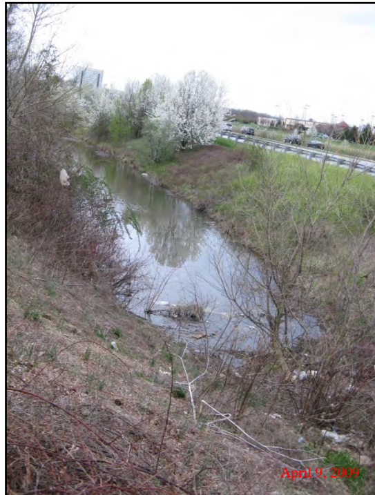
Figure 5. BMP 13348 located along MD-175 east. Photo, looking west, shows single concentrated inflow point to the BMP. Some additional flow will occur from sides of the BMP.
