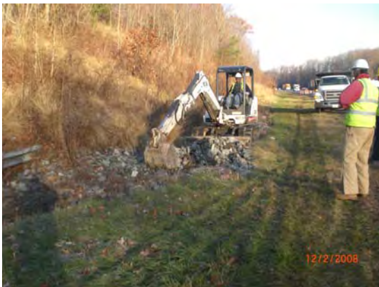
Figure 3-2 BMP 020186 – Removal of Sediment from Infiltration Trench
