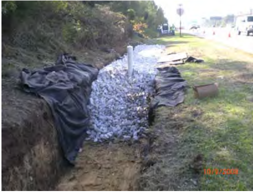
Figure 3-6 Infiltration Trench 020193 In-Kind Replacement
