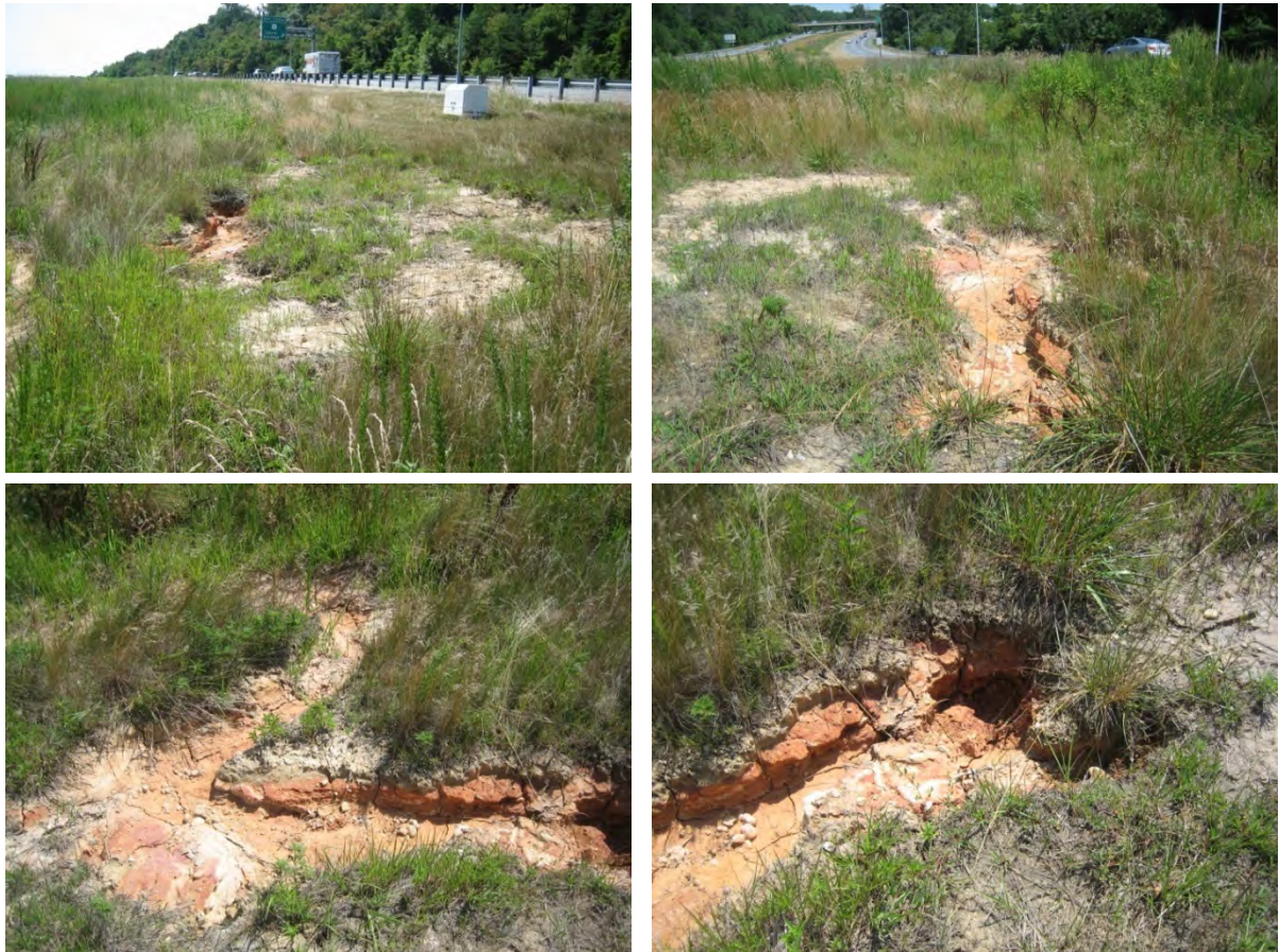
Figure 10. Pits caused by erosion near direct channel
