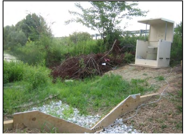
Instrumentation at Failed Infiltration Basin No. 130348
