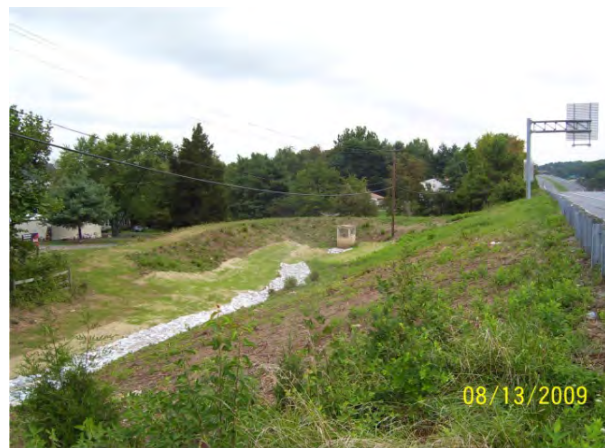
Figure 3-4 Inflow Channel Stabilization (BMP13007) – After Construction
