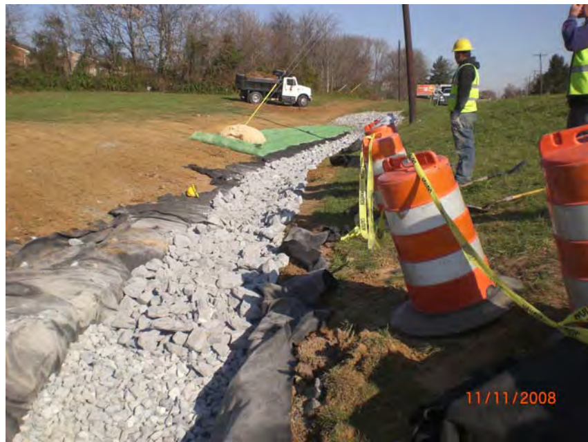
Figure 3-7 Infiltration Trench 210013 In-Kind Replacement
