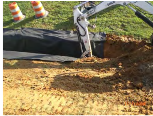
Figure 3-6 Infiltration Trench 020193 In-Kind Replacement
