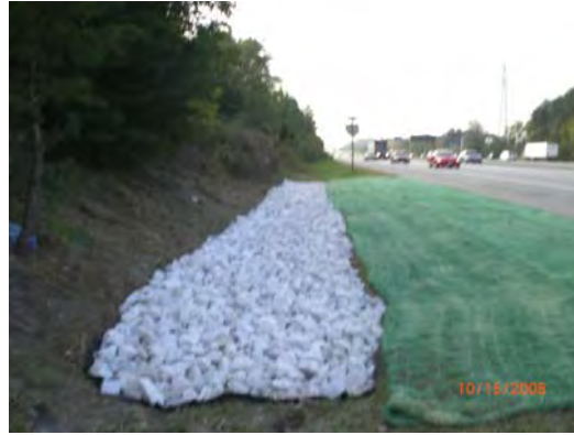
Figure 3-6 Infiltration Trench 020193 In-Kind Replacement
