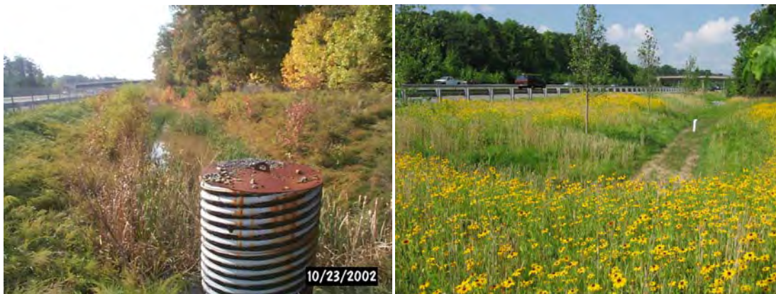
Before the construction (11/2002)
