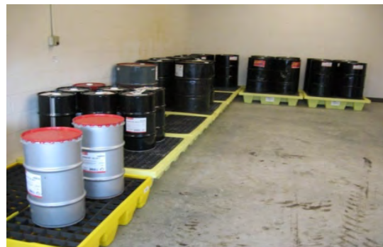
Spill Pallets Used at SHA Maintenance Shops
