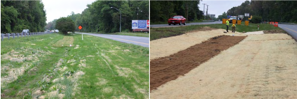
Figure 1-37 Bioswale Construction at US 301 in Charles County
