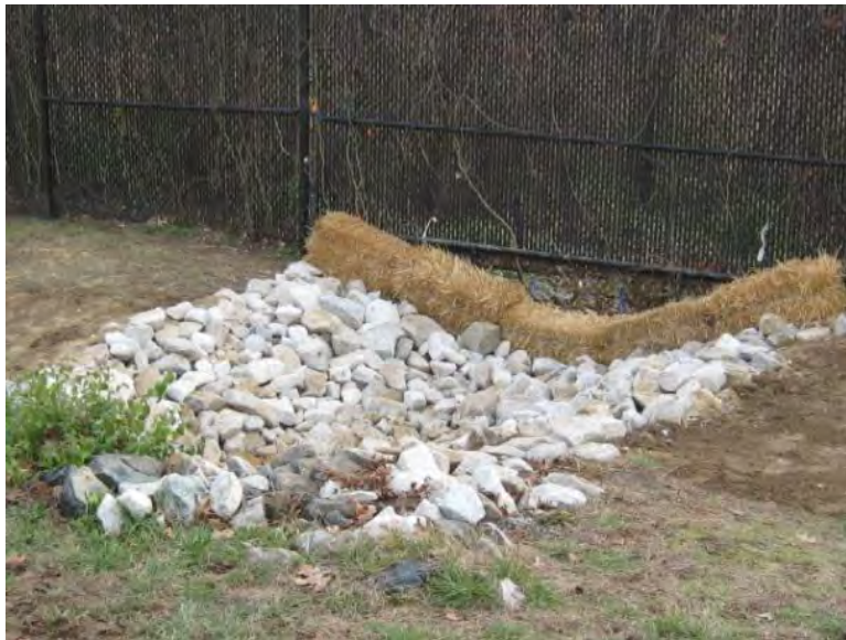
Figure 1-11 Stormwater Outfall Improvements at SHA Maintenance Shop
