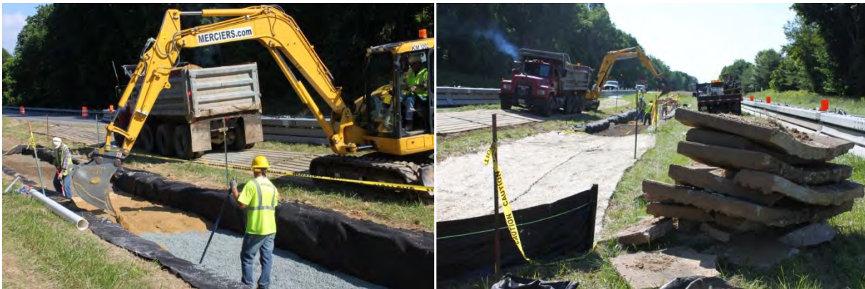
Figure 1-36 Bioswale Construction along US 40 in Howard County
