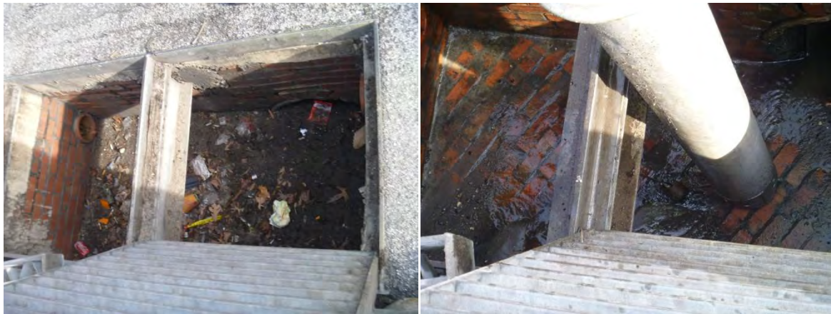
Figure 1-9 Inlet Before (Left) and After (Right) Vacuuming
