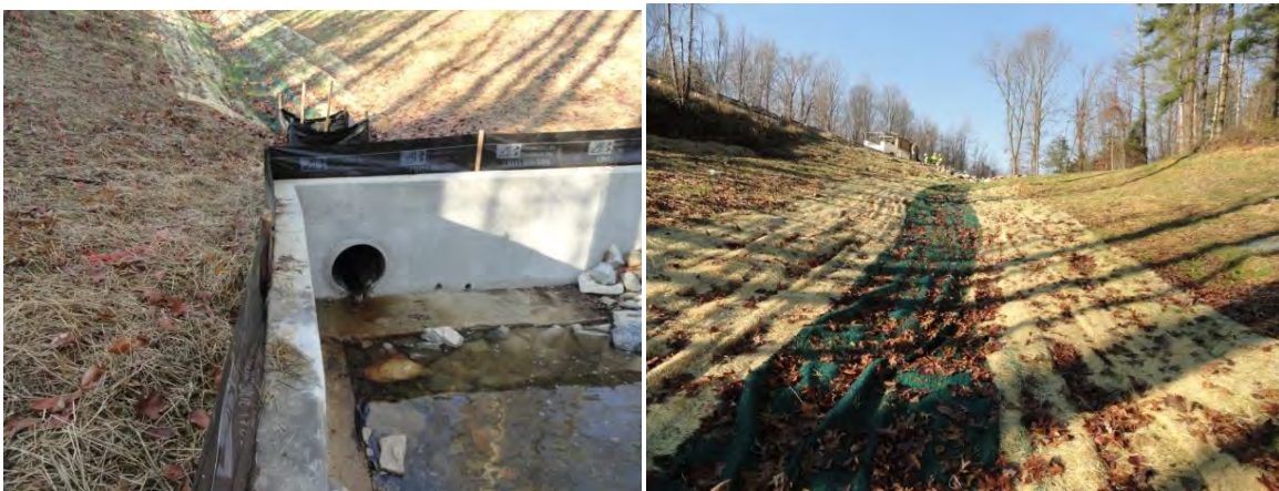
Figure 1-14 Stabilized Outfall along MD 4, Post-Construction
