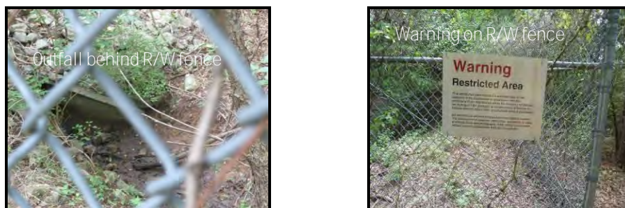
Figure 8.2.10A: Examples of Outfalls which are beyond SHA Right-of-Way
