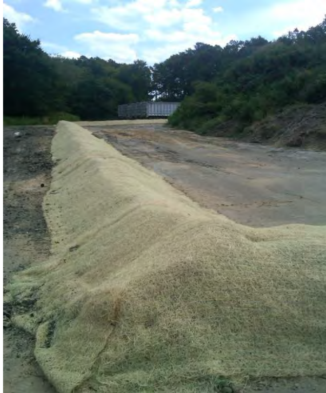
Figure 1-12 Installation of Earthen Berm around Soil Stockpile
