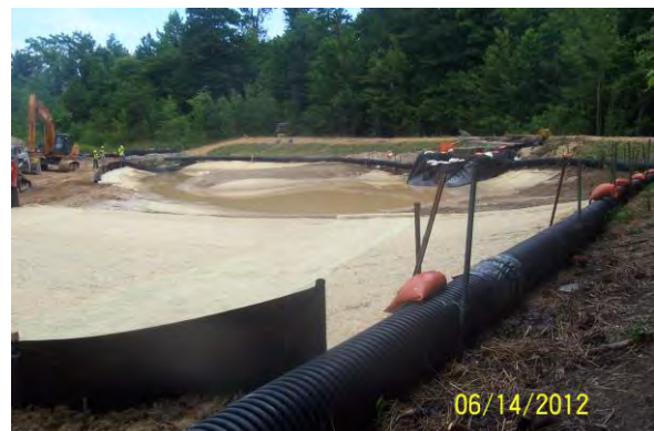
Figure 2-4 Nearing Completion of Work on SWM Facility 120036
