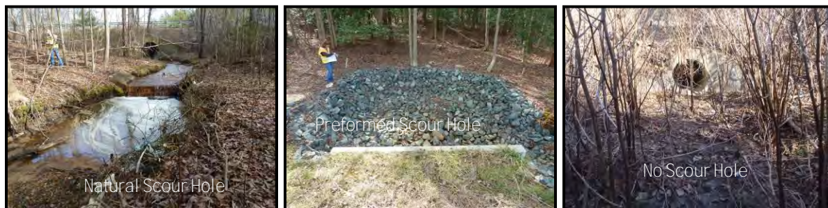
Figure 8.2.21: Examples of Different Types of Scour Holes
