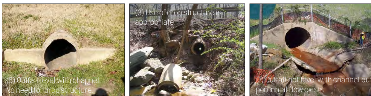
Figure 8.3.1: Examples of Outfalls with Potential for Drop Structures
