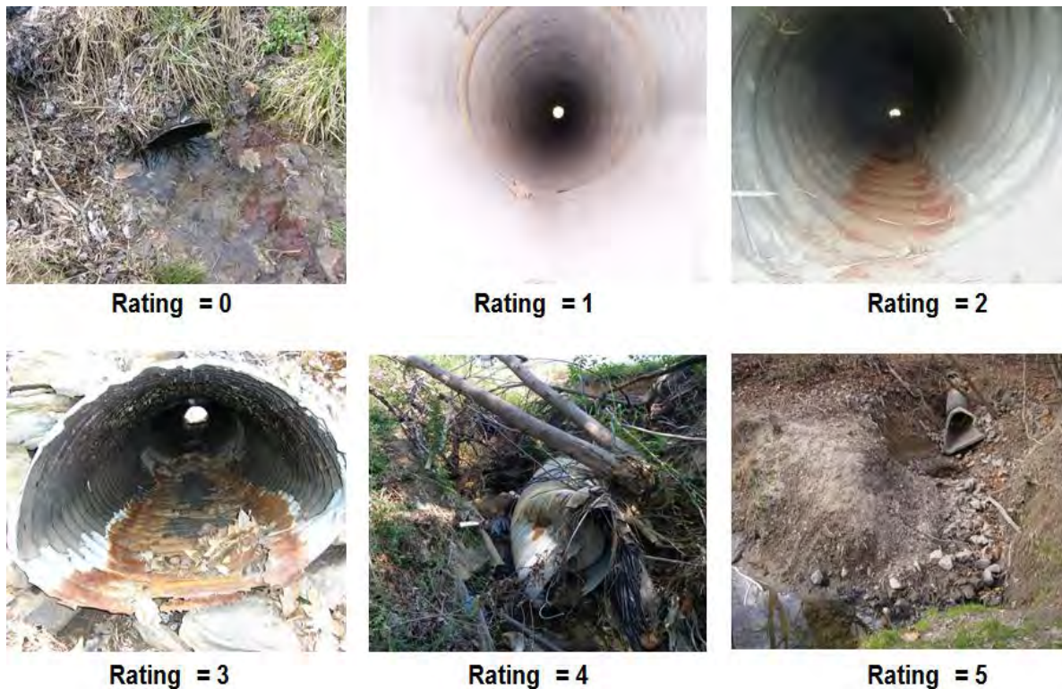
Figure 1-21 Illustrative Examples of Pipe Ratings
