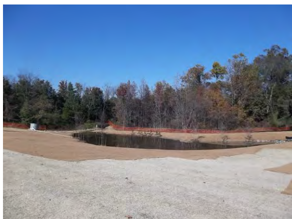
Figure 2-6 MD 4 SWM Facility Enhancement during Stabilization
