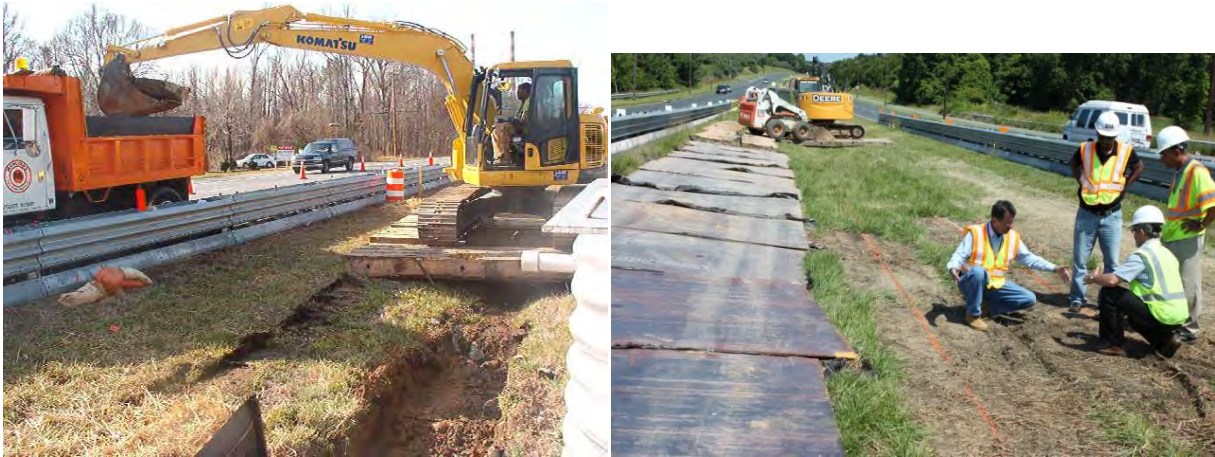
Figure 1-35 Bioswale Construction along MD 119 in Montgomery County
