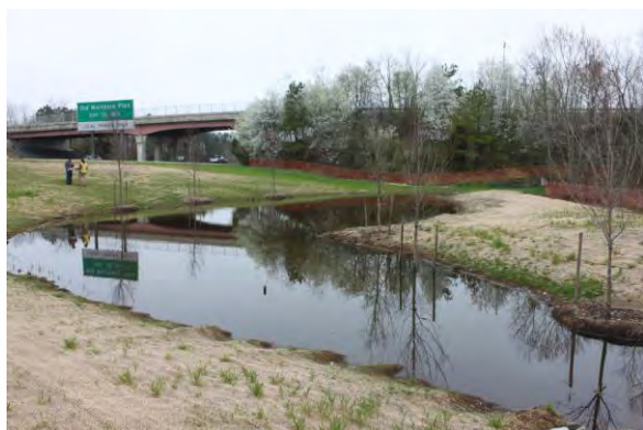
Figure 2-7 MD 4 SWM Facility Enhancement after Completion
