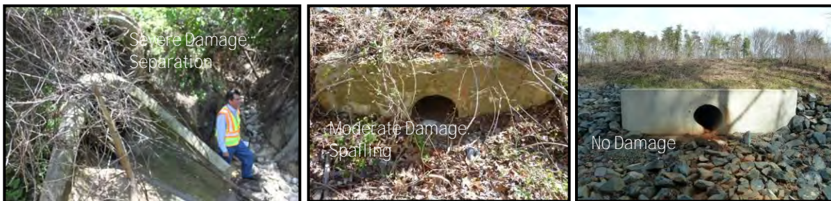
Figure 8.2.13: Examples of Outfall Structure Condition
