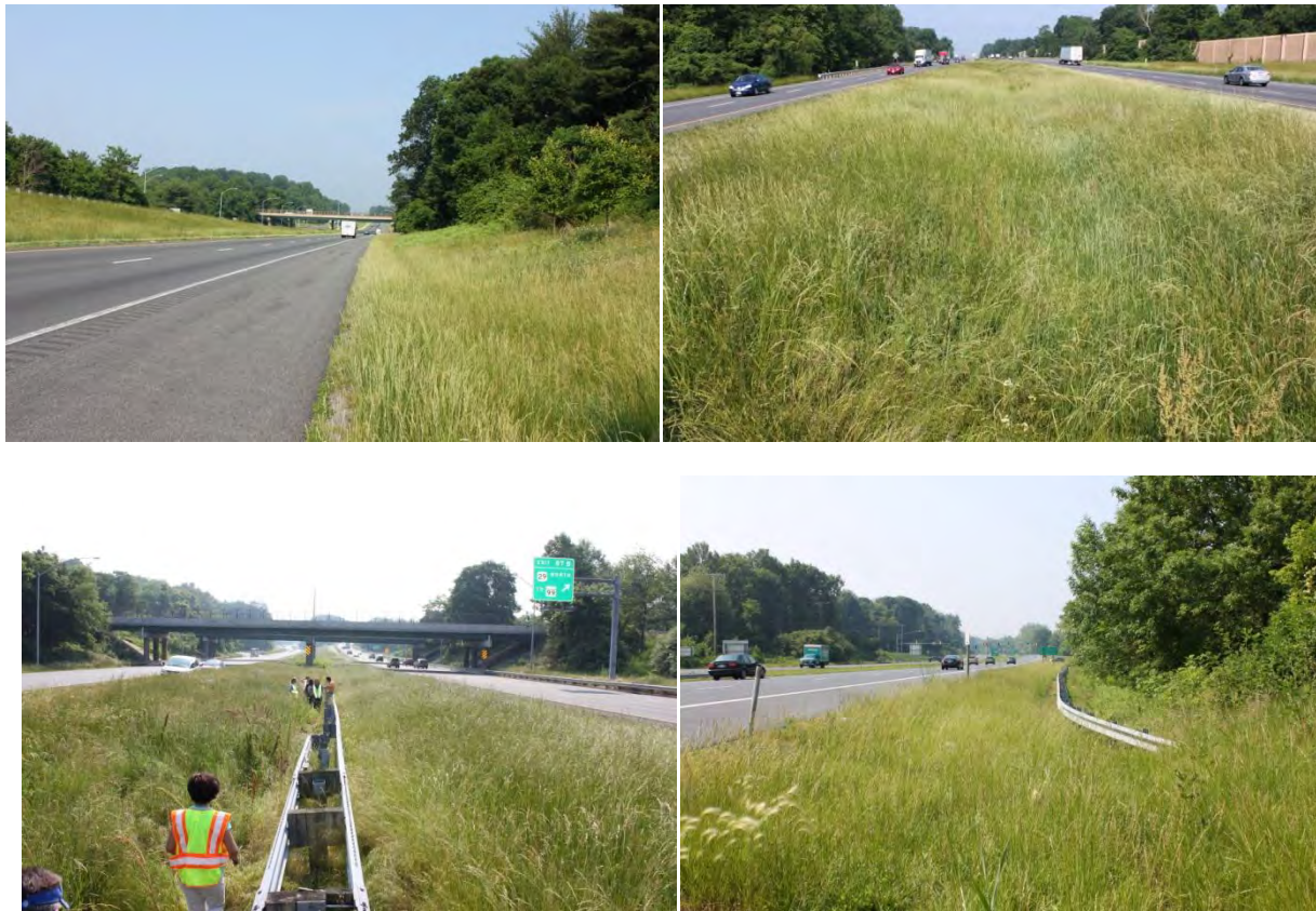
Figure 1-40 Examples of Grassed Swales under Study along I-70
