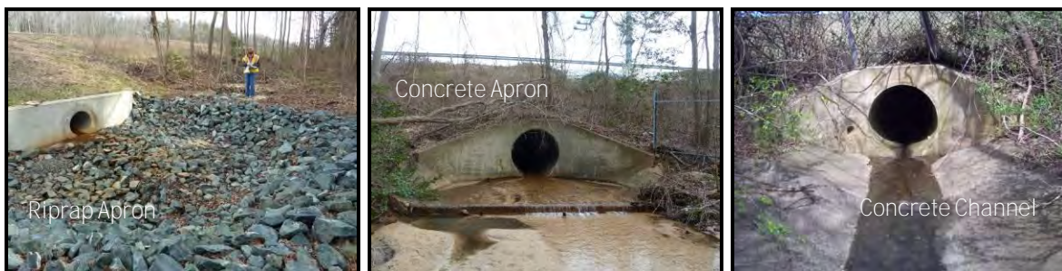
Figure 8.2.17: Examples of Outfall Protection Types
