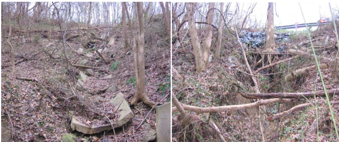
Figure 1-19 Undermined Channel and Washout along US 1 SB, Pre-Construction
