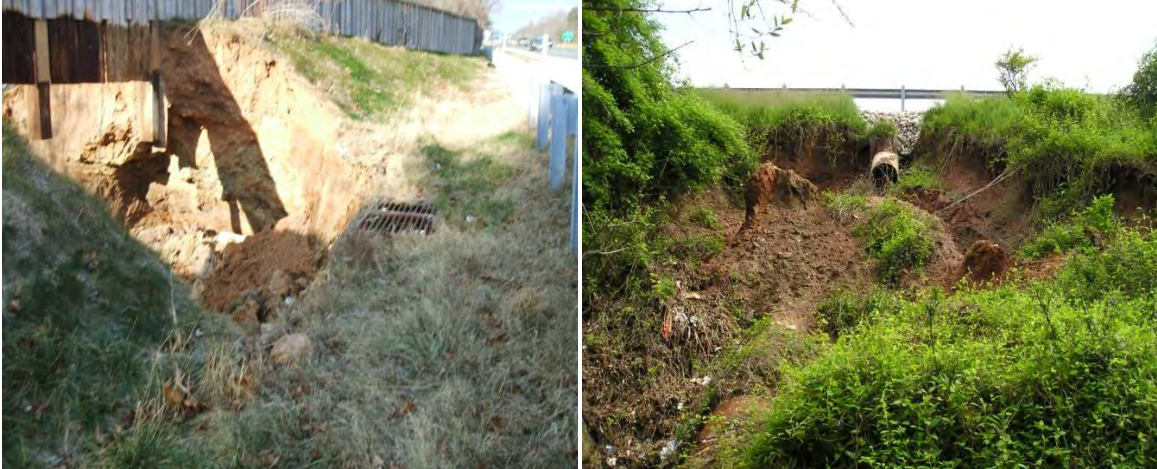
Figure 1-15 Inspected Outfalls along I-795 SB, Pre-Construction. Photo on left is site with existing timber noise barrier.
