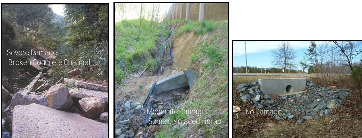
Figure 8.2.19: Examples of Outfall Protection Condition
