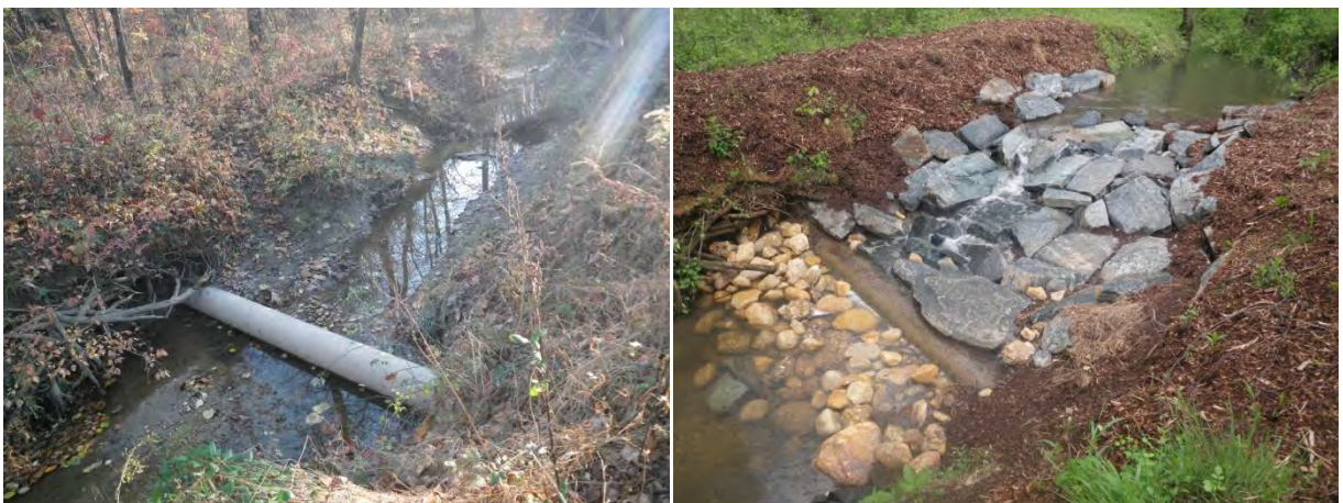
Figure 1-31 Dorsey Run Before (Left) and After (Right) Construction
