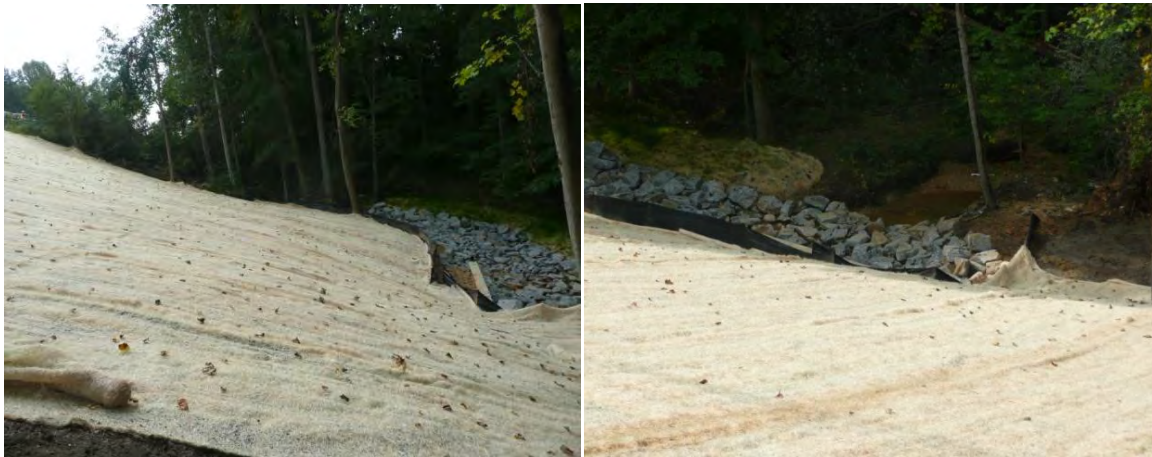
Figure 1-18 Stabilized Outfalls along US 301 SB, Post-Construction
