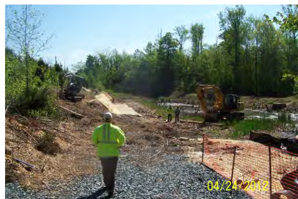
Figure 2-3 Works In Progress on SWM facility 120036
