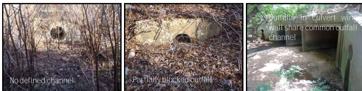
Figure 8.2.22: Examples of Outfall Channels
