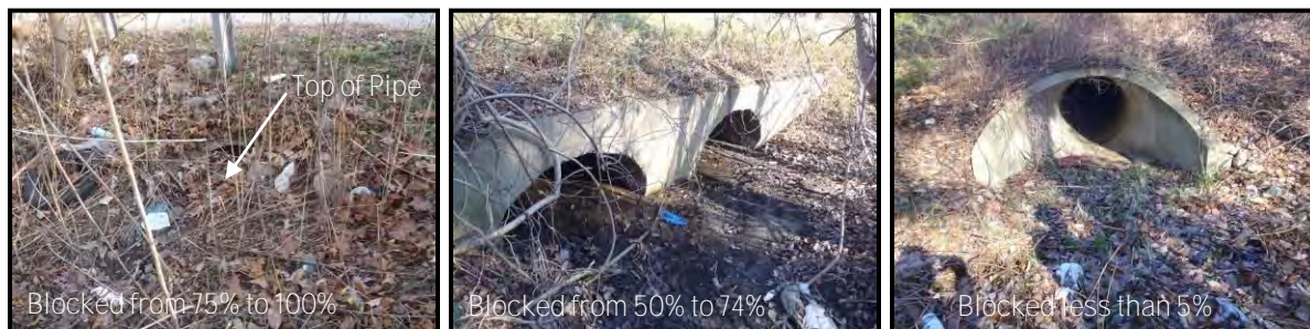
Figure 8.2.16: Examples of Outfall Sediment Blockage
