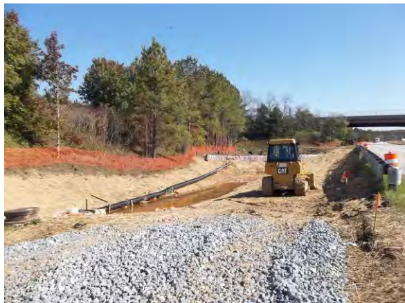
Figure 2-5 MD 4 SWM Facility Enhancement during Construction
