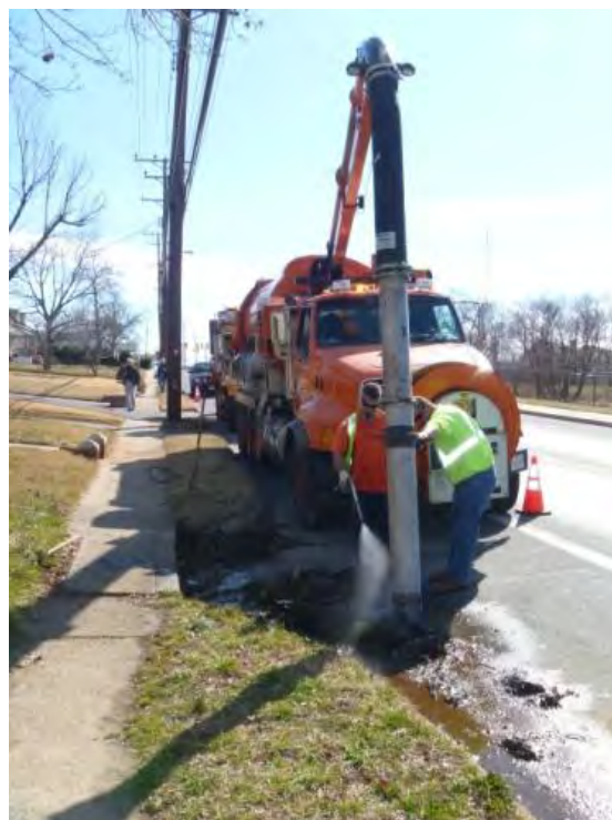
Figure 1-8 SHA Shop Personnel Operating Vacuum Truck to Clean Roadside Debris
