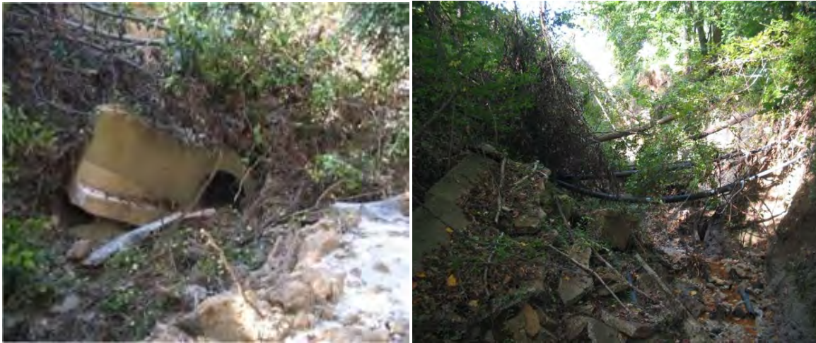
Figure 1-13 Inspected Outfall along MD 4, Pre-Construction
