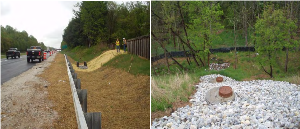
Figure 1-16 Stabilized Outfalls along I-795 SB, Post-Construction. Photo on left is site with existing timber noise barrier.
