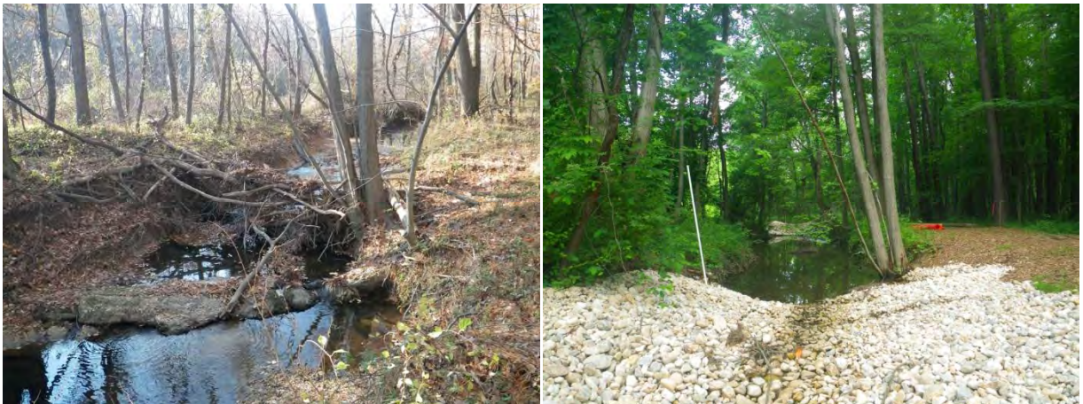
Figure 1-34 Dorsey Run Before (Left) and After (Right) Construction
