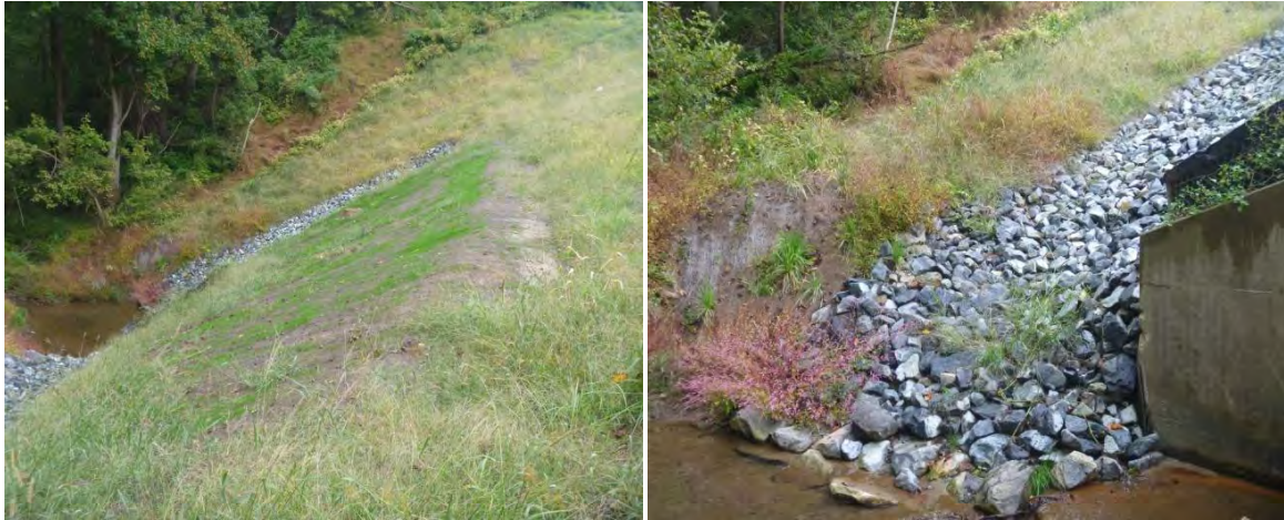
Figure 1-20 Stabilized slope and Channel along US 1 SB, Post-construction
