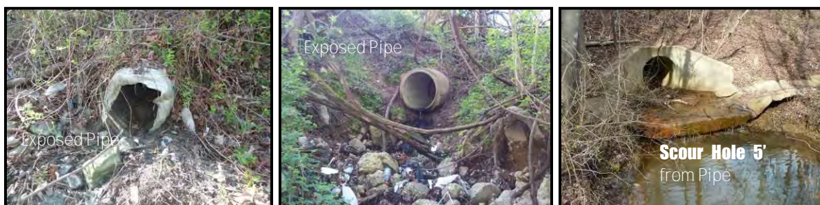
Figure 8.2.20: Examples of Horizontal Pipe Exposure
