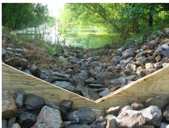
Figure 1-5 Discharge Weir at BMP 130348 for Wet Infiltration Study
