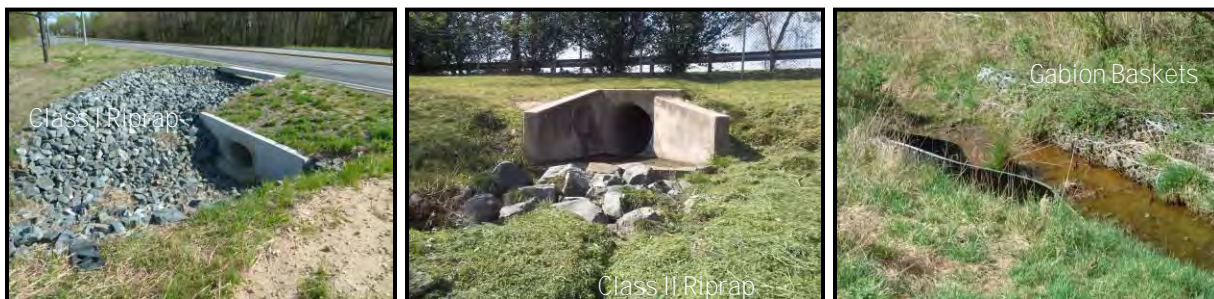
Figure 8.2.18: Examples of Riprap Types at Outfalls
