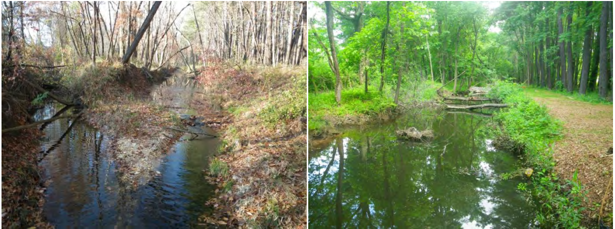
Figure 1-33 Dorsey Run Before (Left) and After (Right) Construction
