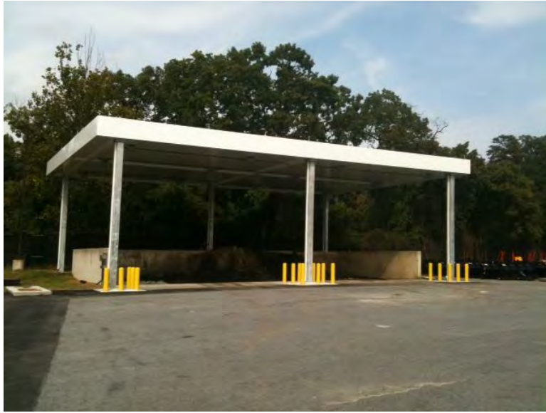
Figure 1-10 Upgrade to Structure used for Inlet Cleaning Waste Dewatering
