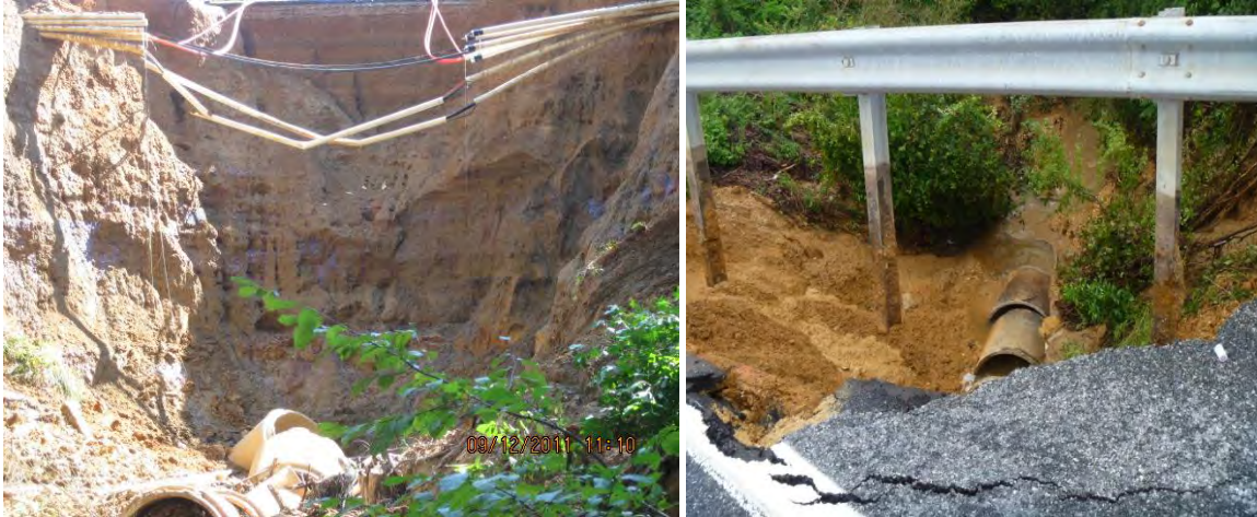
Figure 1-17 Eroded Outfalls along US 301 SB, Pre-Construction. Photo on left is southernmost site, with exposed fiber optic line.
