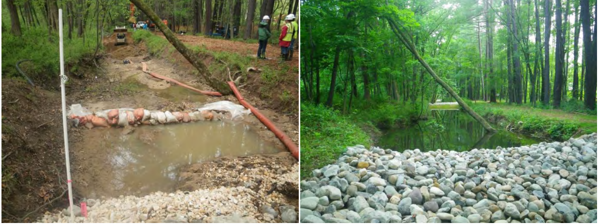
Figure 1-32 Dorsey Run Before (Left) and After (Right) Construction
