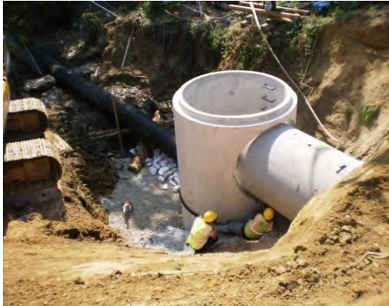
Figure 1-20 MD202 Outfall stabilization installation of drop structure
