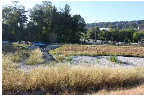
Figure 2-9 I-695 at Charles Street SWM Retrofit after construction completion
