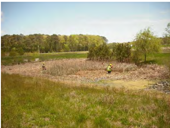
Figure 2-2 Routine maintenance activities in progress on SWM facility 230011
