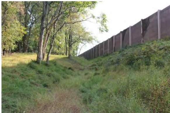
Figure 1-26 MD 100 Outfall and drainage swale stabilization after construction
