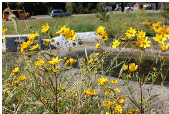
Figure 1- 29 MD 147 and I-695 SE Loop – SWM Water Quality Retrofit Project shortly after construction
