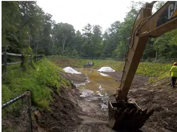
Figure 2-6 Nearing Completion of work on SWM Facility 020296
