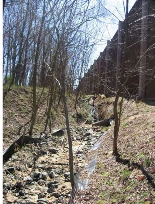
Figure 1-25 MD 100 drainage swale stabilization before construction
