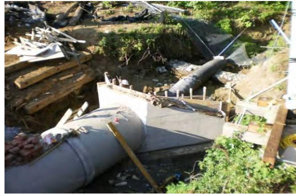
Figure 1-21 MD 202 Outfall stabilization headwall construction
