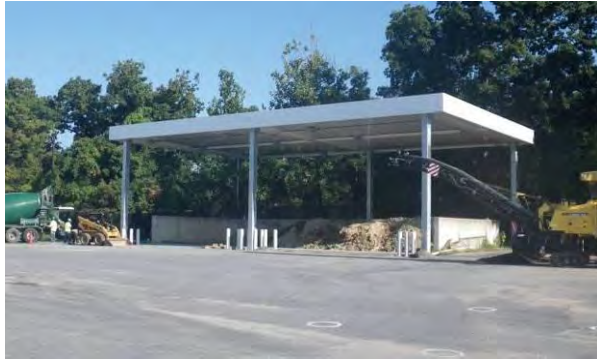
Figure 1-14 Structure used for Inlet Cleaning Waste Dewatering
