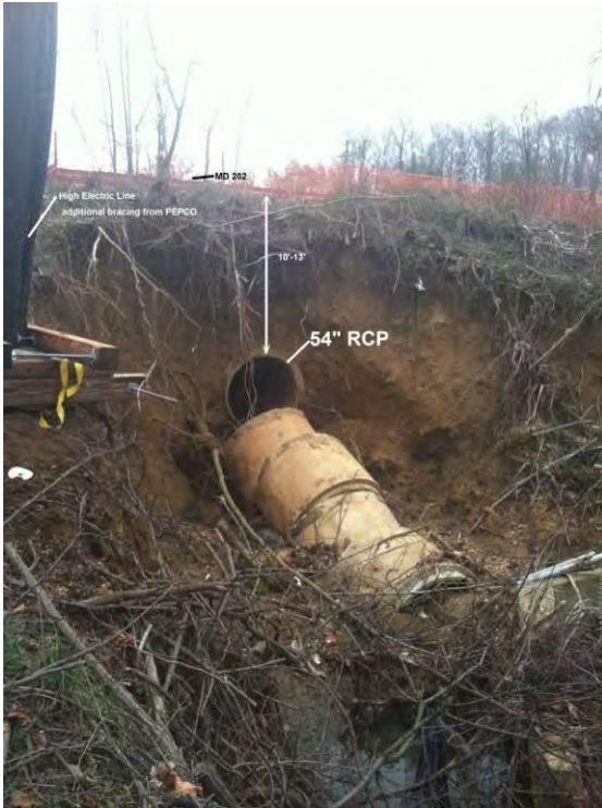
Figure 1-19 MD 202 Outfall stabilization before construction
