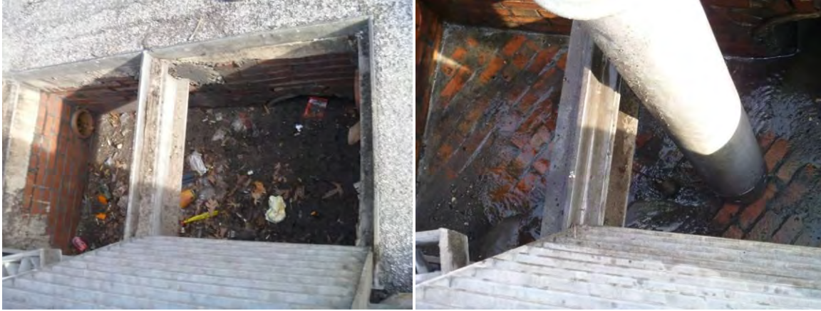
Figure 1-13 Inlet Before and After Vacuuming
