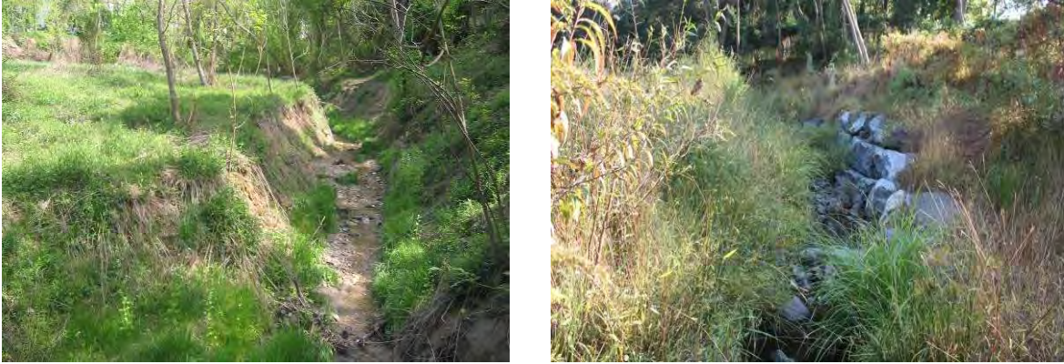
Figure 1- 36 Tributary to Red Branch restoration before and after construction
