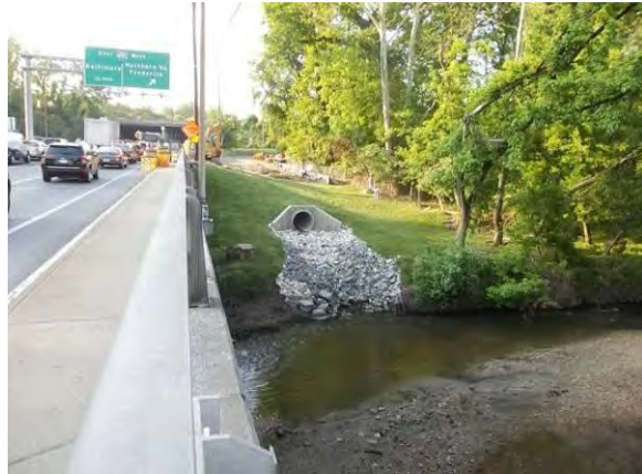
Figure 1-17 MD185 at Rock Creek Outfall restoration during and after construction
