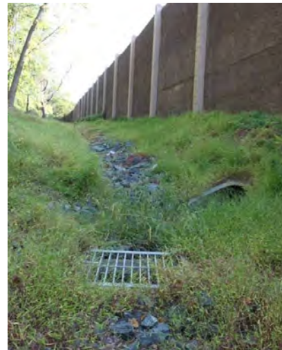
Figure 1-26 MD 100 Outfall and drainage swale stabilization after construction
