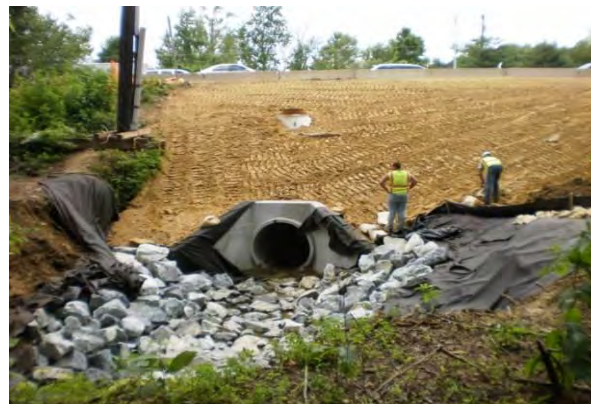
Figure 1-23 MD 202 Outfall stabilization after construction
