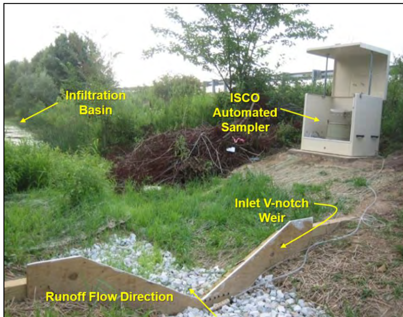
Figure 3. Photograph showing the sampler and weir installed at the inlet side of the infiltration basin.
