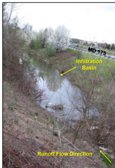
Figure 1. Photograph showing the infiltration basin located along MD 175 East. Photo, looking west, shows single concentrated inflow point to the infiltration basin.
