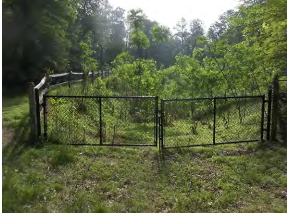
Figure 2-5 SWM Facility 020296 prior remedial maintenance
