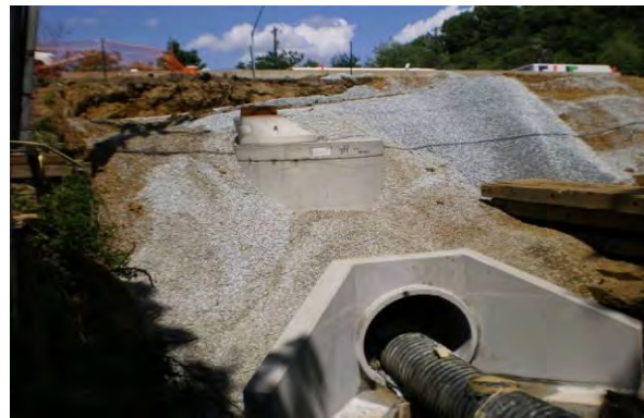
Figure 1-22 MD 202 Outfall stabilization during construction
