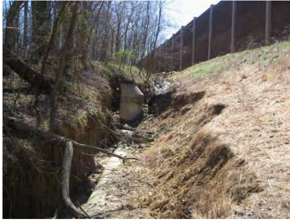
Figure 1-24 MD 100 Outfall stabilization before construction
