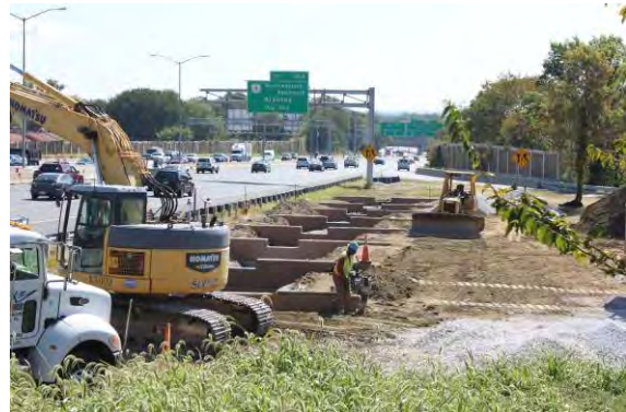
Figure 2-8 I-695 Widening - SWM facility during construction
