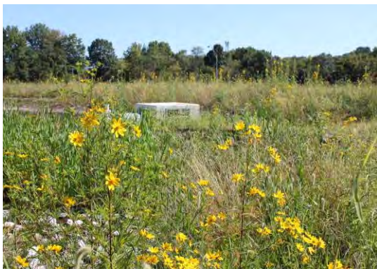
Figure 2-7 I-695 at MD 147 SWM retrofit after construction
