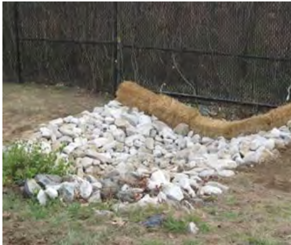
Figure 1-15 Stormwater Outfall Improvements at SHA Maintenance Shop
