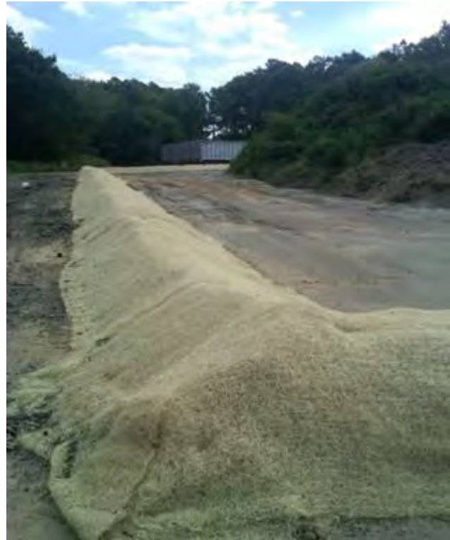
Figure 1-16 Installation of Earthen Berm around Soil Stockpile
