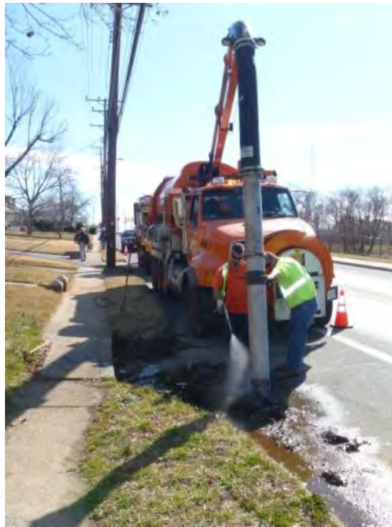
Figure 1-12 SHA Shop Personnel Operating Vacuum Truck to Clean Roadside Debris
