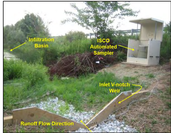
Figure 1-5 Wet Infiltration Basin Study – Site Monitoring Set Up
