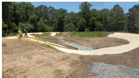
Figure 2-4 Works in progress on SWM facility 020697
