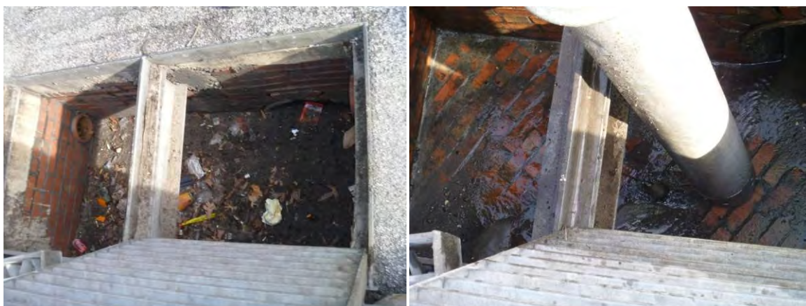
Figure 1-16: Inlet Before and After Vacuuming
