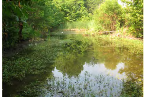
Figure 2-5 Infiltration Basin Rated IV (significant flooding and water not able to be retained in the original footprint.)
