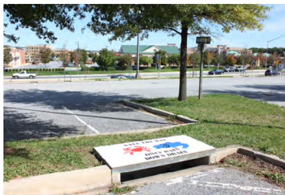
Figure 1-24: Finished Stencil Design on Storm Drain
