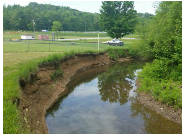
Figure 1-38: Existing Conditions at Little Tonoloway Creek in Washington County
