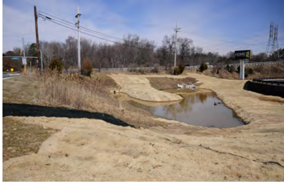
Figure 2-6: Major maintenance performed on BMP 030181 in Baltimore County
