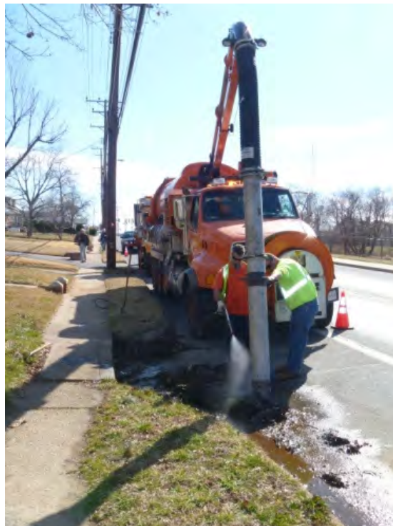
Figure 1-15: SHA Shop Personnel Operating Vacuum Truck to Clean Roadside Debris
