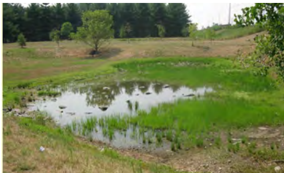
Figure 2-4: Infiltration Basin Rated III (Infiltration is hampered and flooding beginning)
