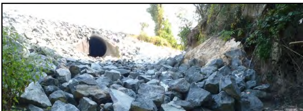
Figure 1-11: Stabilized Outfall, I-97 in Anne Arundel County
