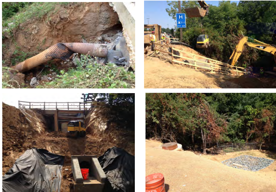
Figure 1-17: Outfall Remediation at I-270 in Montgomery County
