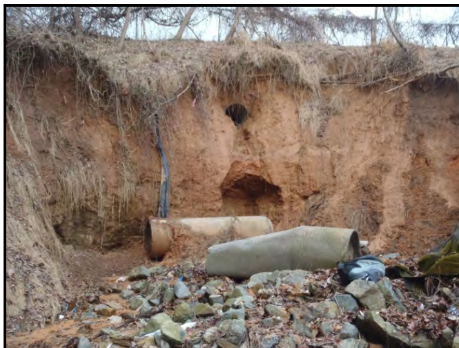
Figure 1-10: Outfall in need of Stabilization, I-97 in Anne Arundel County
