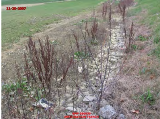
Figure 2-3: Infiltration Trench Rated II requiring vegetation and trash removal
