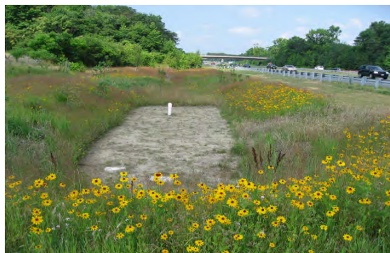
Figure 2-2: Infiltration Sand Filter Rated I
