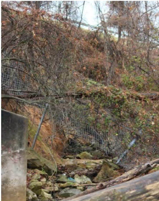
Figure 1-32: Stormwater Retrofit Site at Minebank Run
