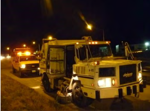
Figure 1-14: Street Sweeping often takes place at night due to high traffic volumes in urbanized counties
