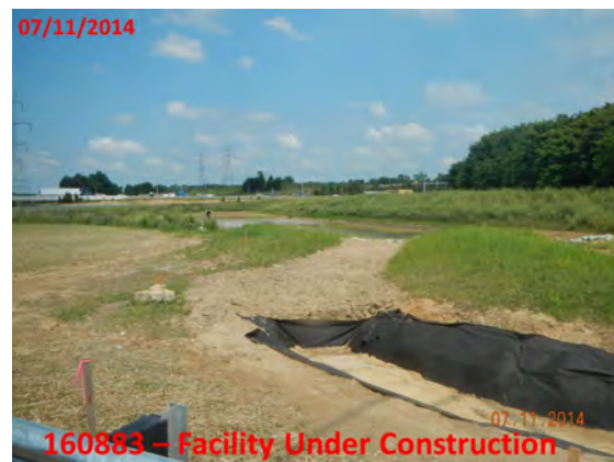
Figure 2-7 – SWM Facility 160883 Under Retrofit Construction
