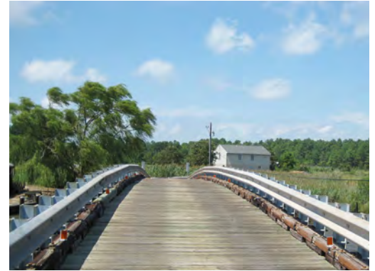
Figure 4-62 Bridge rail should better match wooden structure at Bestpitch
