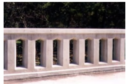
Figure 4-64– Open concrete parapet walls such as found on the Marshy Hope Creek Bridge (page 65) can be replicated to TL-2 standards using the Texas T411 Parapet Wall (source FHWA Bridge Guide, 2005)
