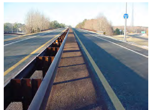
Figure 4-59 – MD 90 shoulder and guardrail
