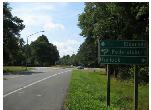
Figure 4-52 Existing roundabout near Federalsburg
