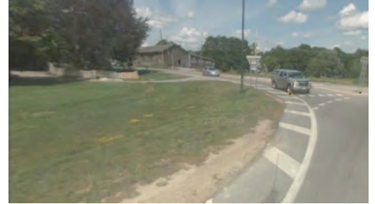
Figure 4-54 Pavement edge without curbing in upstate New York has deteriorated (Source Google Earth photograph)
