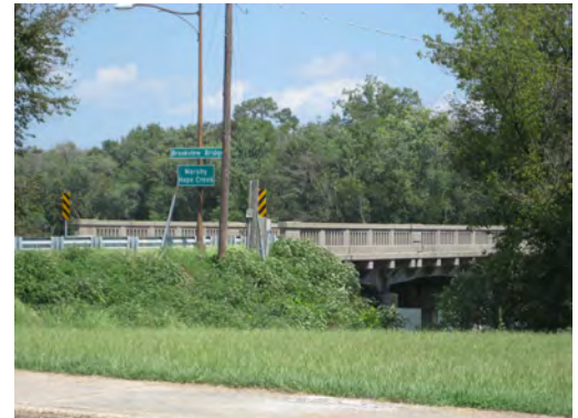
Fig. 4-8 Brookview Bridge over Marshyhope Creek
