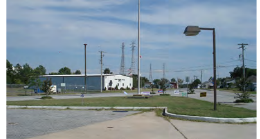
Fig. 4-5 Transmission lines near Vienna, MD
