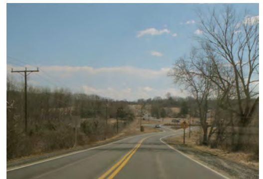
Figure 4-56 – Roundabout on Route 50 east of Gilberts Corner in context
