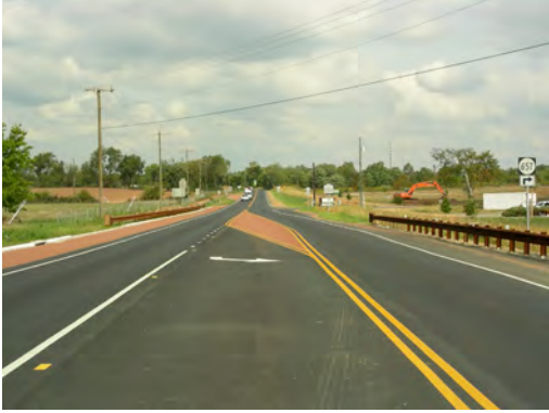
Figure 4-60 – US Route 15 near Leesburg, VA
