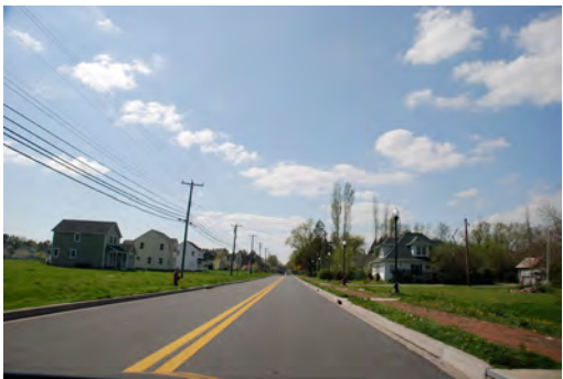
Figure 4-49 Transition approaching East New Market
