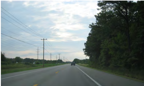
Figure 3-20 MD 33 is listed as a high priority in the Highway Needs Inventory and if reconstructed would provide an opportunity for context sensitive solutions approaches to enhance the less attractive portions of the corridor
