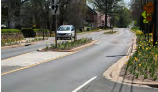
Figure 4-57 Splitter islands installed in Upperville, Virginia to slow traffic coming through the rural town
