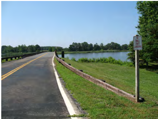
Figure 4-61 – Example of well matched wooden approach rail on bridge to Wye Island (Wye Island Road)
