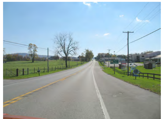
Figure 29 Western entrance to Boonsboro
