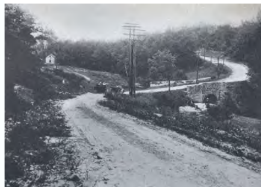
Figure 11 Puzzley Run Bridge, 1930s
