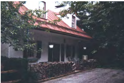
Figure 36 Former toll house on Frederick Pike at the Jug Bridge over the Monocacy
