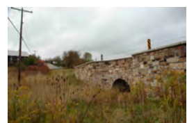
Figure 7 Maryland SHA utilized Context Sensitive Design approaches for rehabilitating the Sideling Creek bridge (top) and the stone bridge at Little Meadows (bottom)
