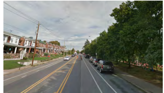
Figure 47 4200 Block of Frederick Avenue - consideration should be given to using a different type of pavement or pavement marking to differentiate either the parking or bicycle lanes from the travel lanes. Street trees on the north side could also help enclose the street and add more visual friction," encouraging drivers to slow travel speeds
