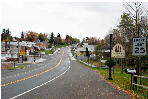
Figure 25 Frostburg western entrance, looking east
