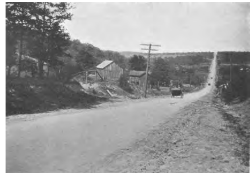
Figure 18 The Long Stretch during the revival era (Photograph Courtesy of FHWA)
