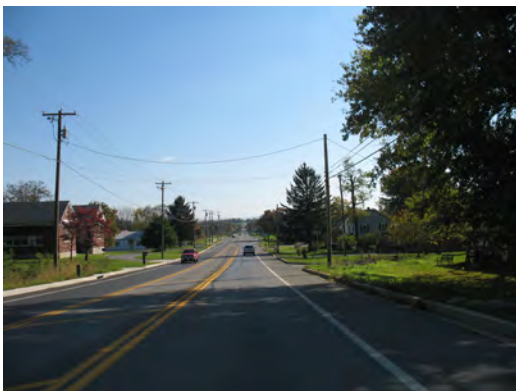
Figure 32 Looking east approaching Hagerstown near Greencastle Pike
