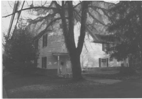
Figure 35 Former toll house on Old National Pike at Braddock Heights
