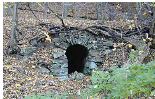
Figure 23 Stone culvert along the original Greene Street alignment of the National Road (Photograph Courtesy of Steve Colby)
