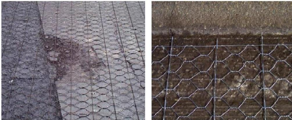
**Figure 13: General Configuration of Two Types of Steel Reinforcement**
