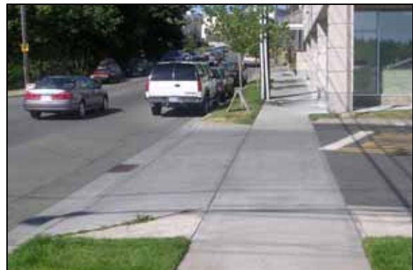
Figure 9.9 - Example of a Continuous Pedestrian Route over a Depressed Curb Entrance where there is a Buffer between the Sidewalk and the Curb (An example application of Standard No. 630.02)
