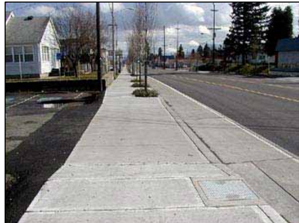
Figure 9.9 - Example of a Continuous Pedestrian Route over a Depressed Curb Entrance with Vertical Deflection (An example application of Standard No. 630.01)
