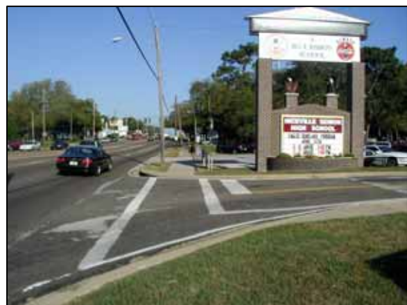
Figure 9.10 - Example of a Commercial Two-Way Entrance
