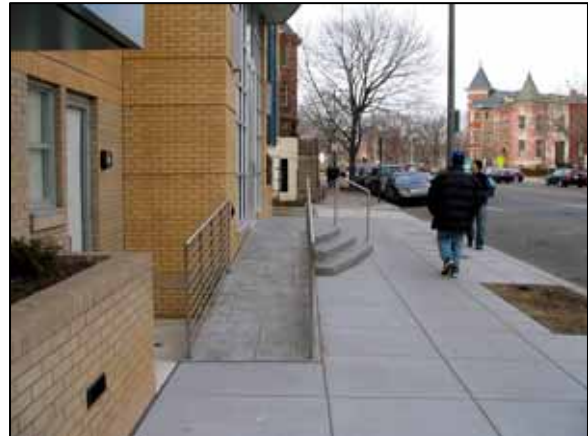
Figure 9.6 - Example of Building Entrance Higher than Sidewalk
