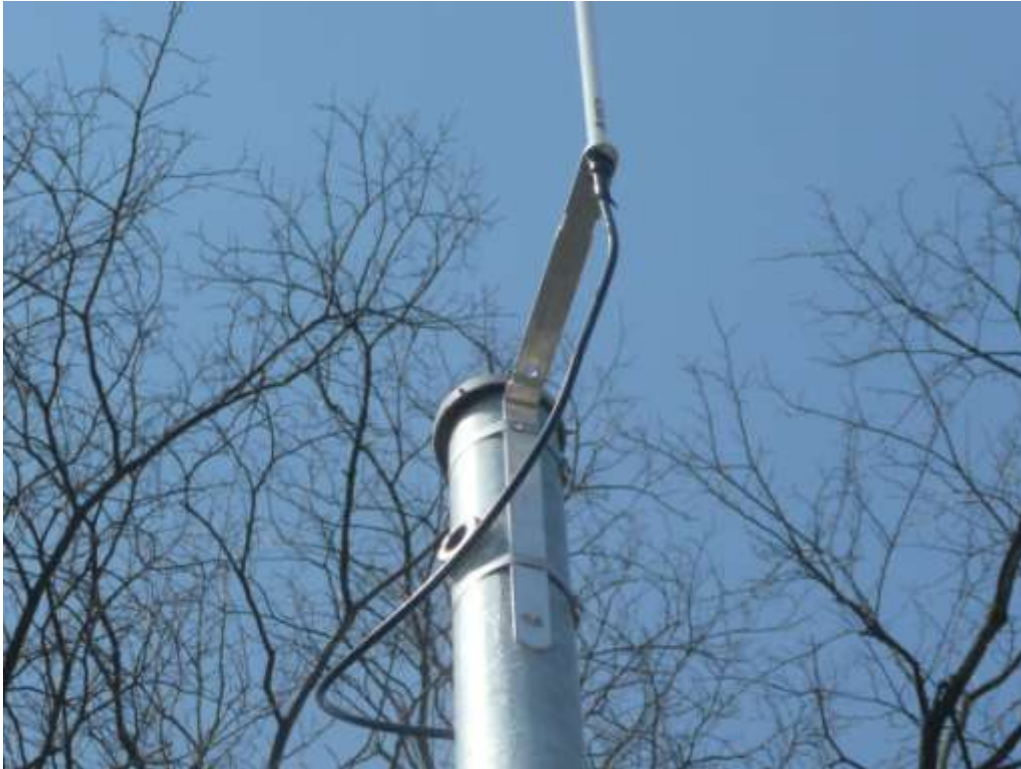
Figure 62. Antenna Cable Routing at the Pilot VWS
