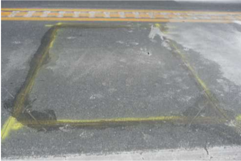
Figure 6. Loop Detector at the Pilot VWS
