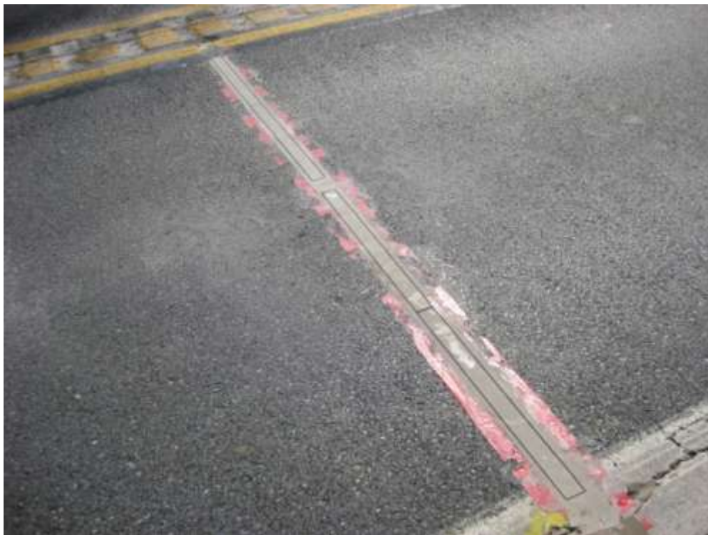
Figure 5. Weigh-In-Motion (WIM) Sensor at the Pilot VWS (Two Sets)
