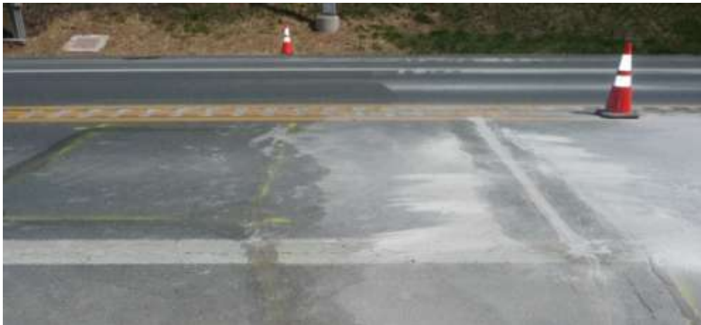
Figure 7. Loop Detector and Quartz Piezo WIM Sensor Layout at the Pilot VWS
