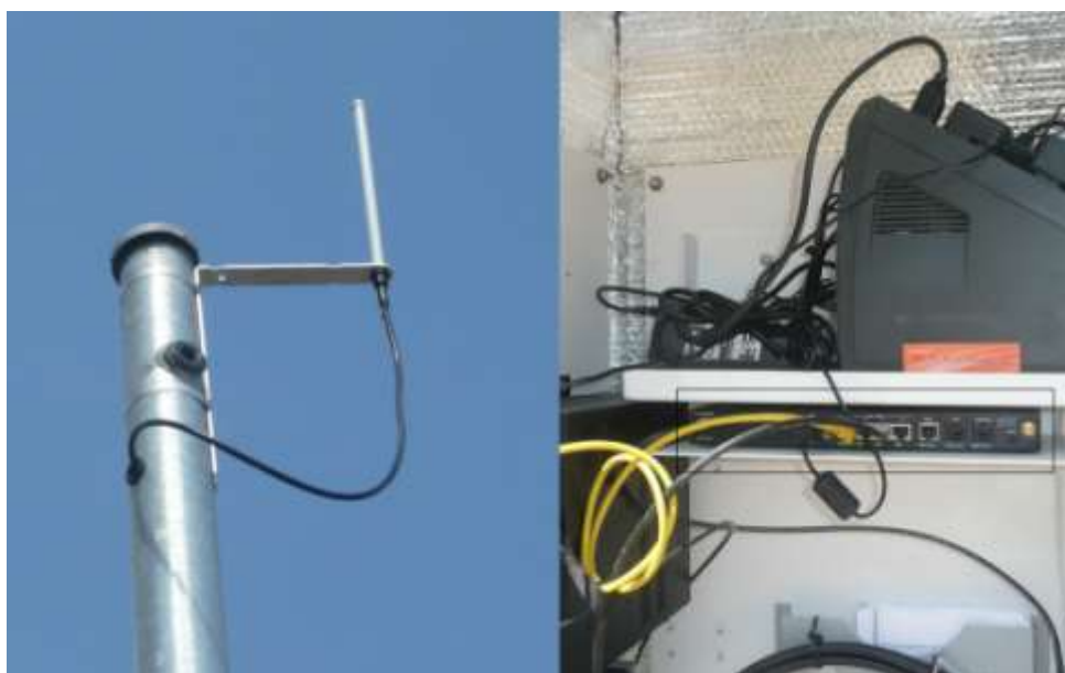
Figure 14. Cell Antenna and Proxicast Cell Router at the Pilot VWS
