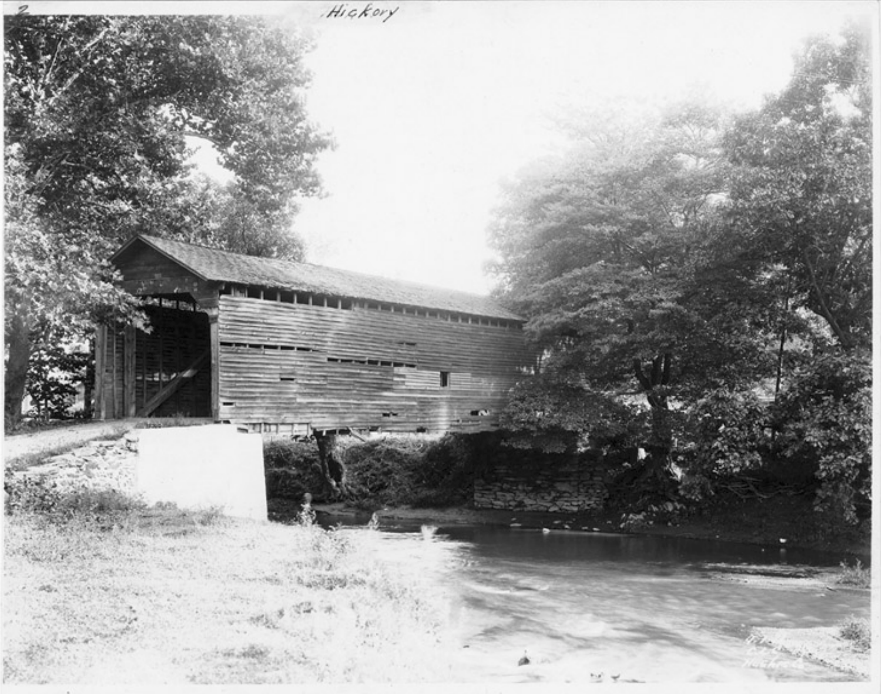
PLATE 1: Typical Timber Covered Bridge: Bridge at Hickory
