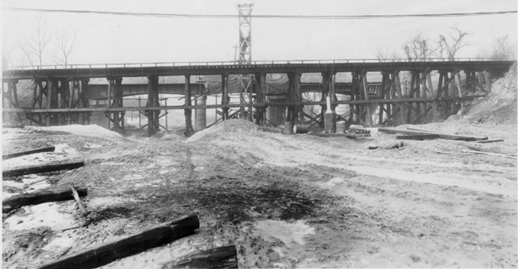
PLATE 3: Typical Timber Trestle: Bridge Crossing Gwynns Falls in Baltimore
