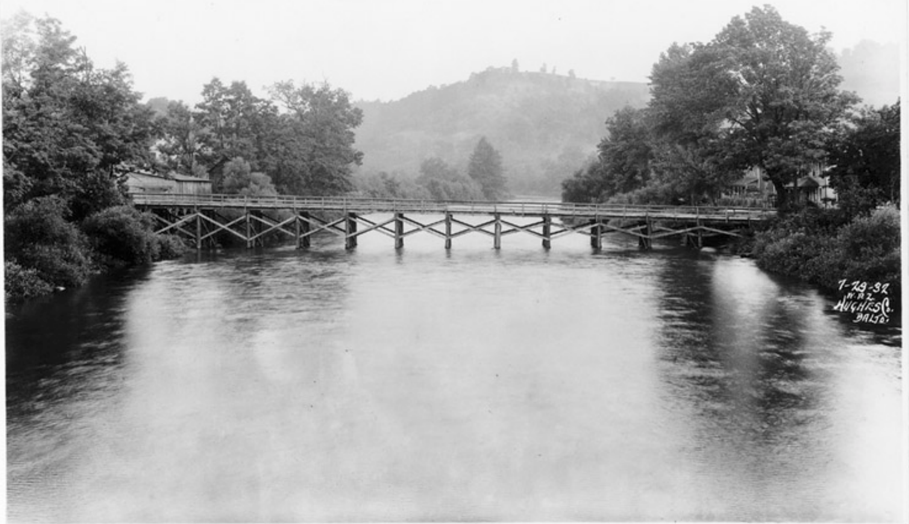
PLATE 2: Typical Timber Multiple-Span Beam Bridge: Bridge at Friendsville
