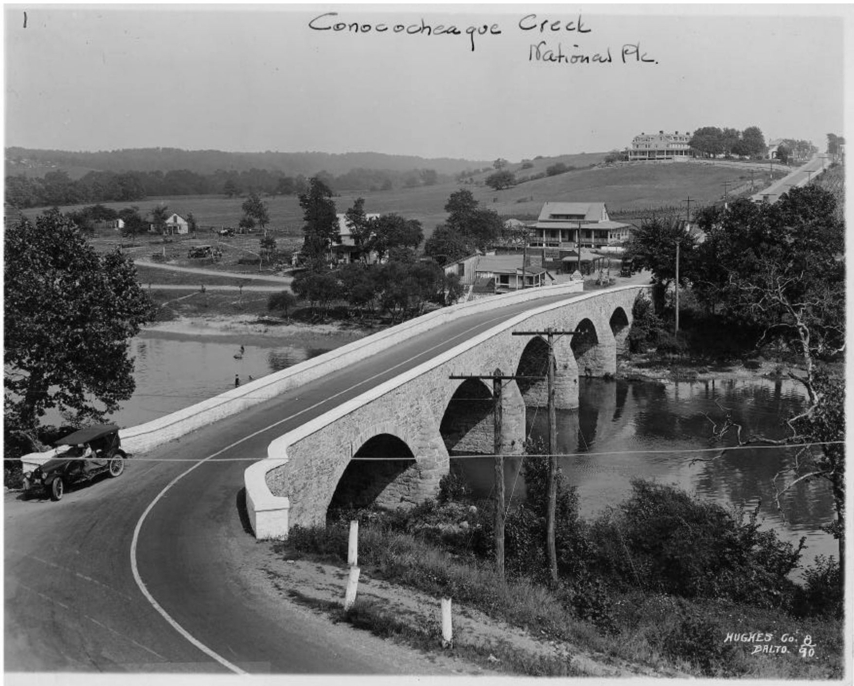
PLATE 4: Typical Multiple-Span Stone Arch Bridge: Wilson's Bridge Crossing Conococheague Creek on the National Pike
