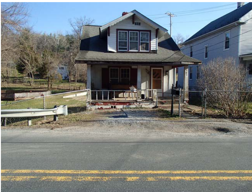
Figure 3-2. Dwelling at 703 West Potomac Street, Part of the Brunswick Historic District (NRHP # F-2-009)
