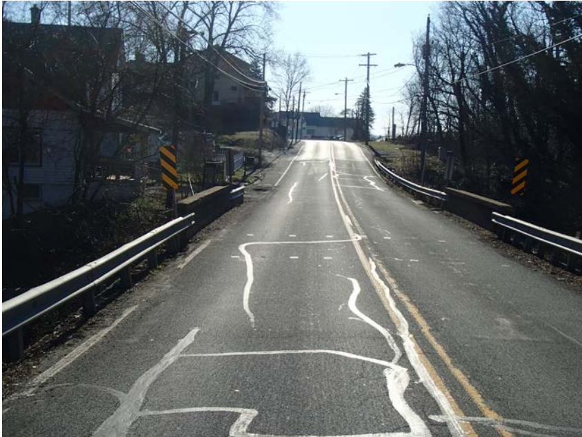
Figure 3-3. Looking East on MD 478 at Bridge No. 10089 and 703 West Potomac Street
