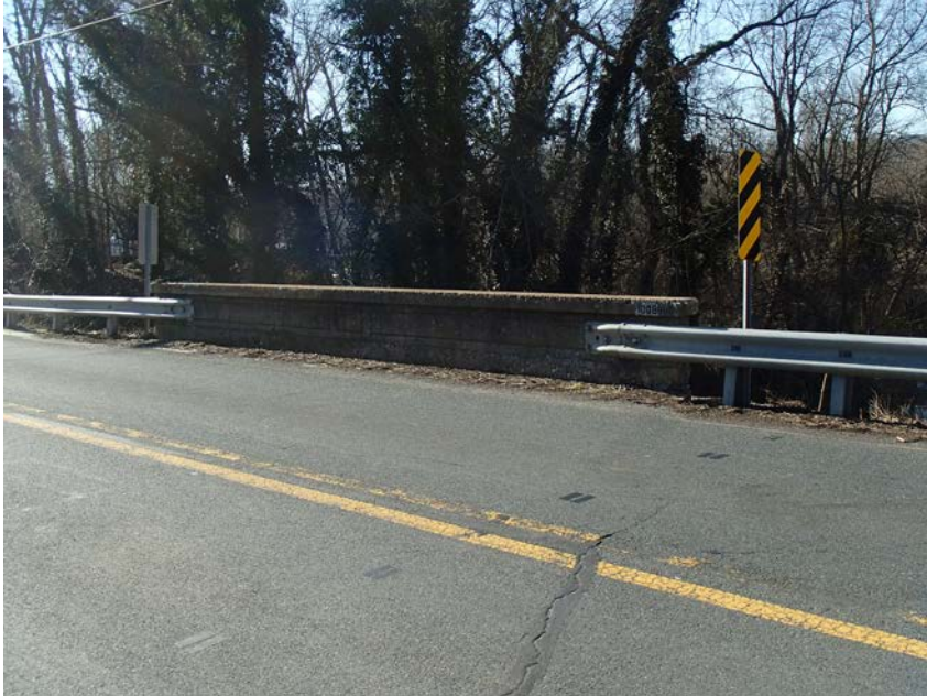
Figure 3-1. SHA Bridge No. 10089 (MIHP # F-2-92)
