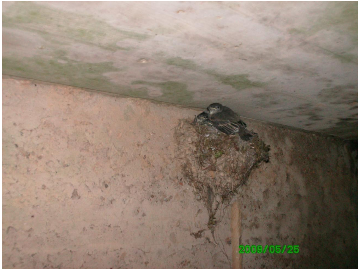
Figure 15. Eastern phoebe nestlings in a nest on a wall of a box culvert in Maryland.
