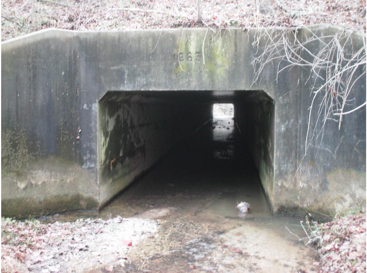
Figure 2. Culvert 02015X0 is 8 feet (2.4 m) wide, 6 feet (1.8 m) tall by 104 feet (31.7 m) long with 3 inches (7.6 cm) of water. This box culvert cell had a concrete substrate.
