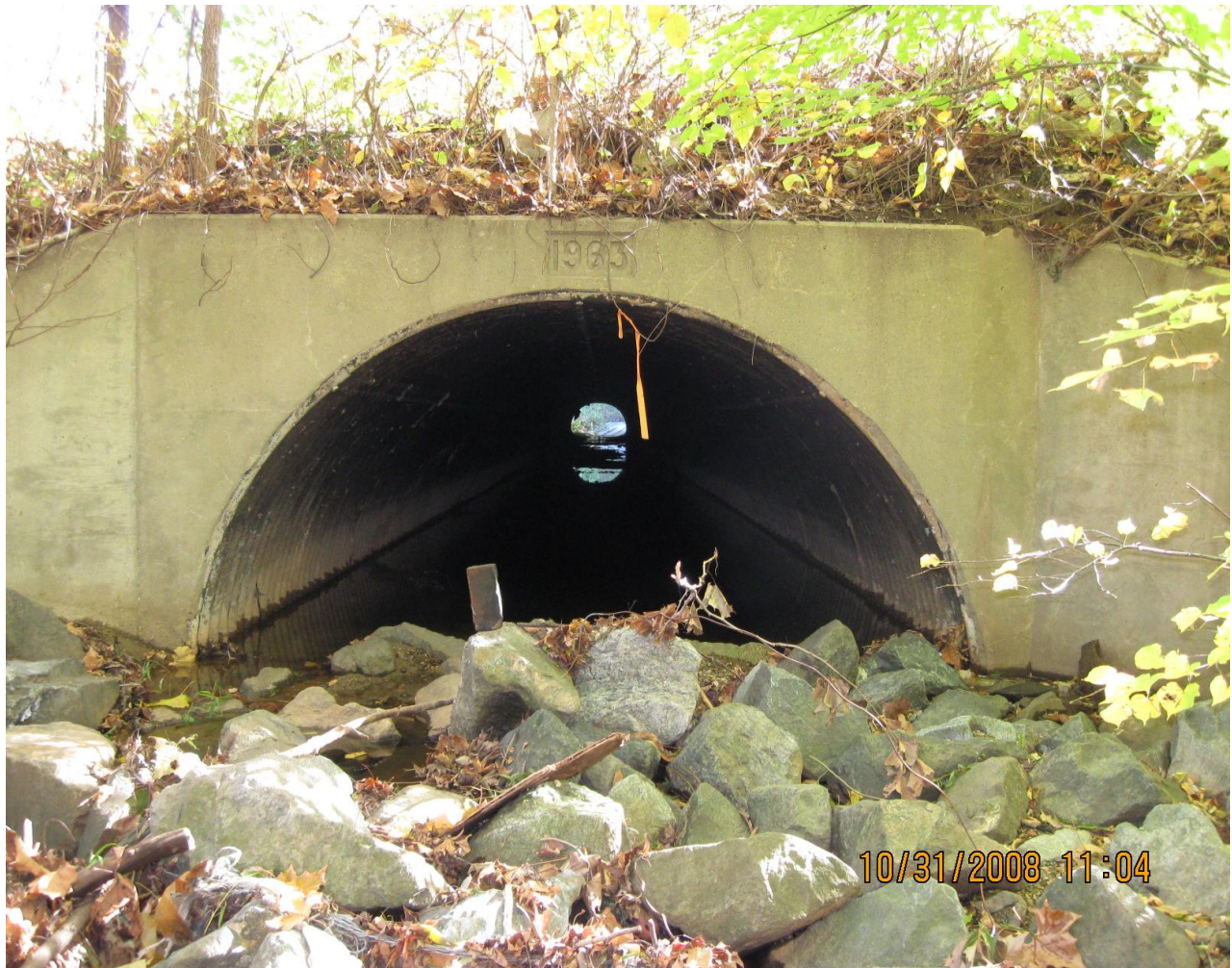
Figure 1. Culvert 15138X0 is 11 feet, 10 inches (3.6 m) wide, 7 feet 7 inches (2.3 m) tall, and 256 feet (78.8 m) long with 6 inches (15 cm) of water. This arch culvert cell had a gravel and sand substrate.
