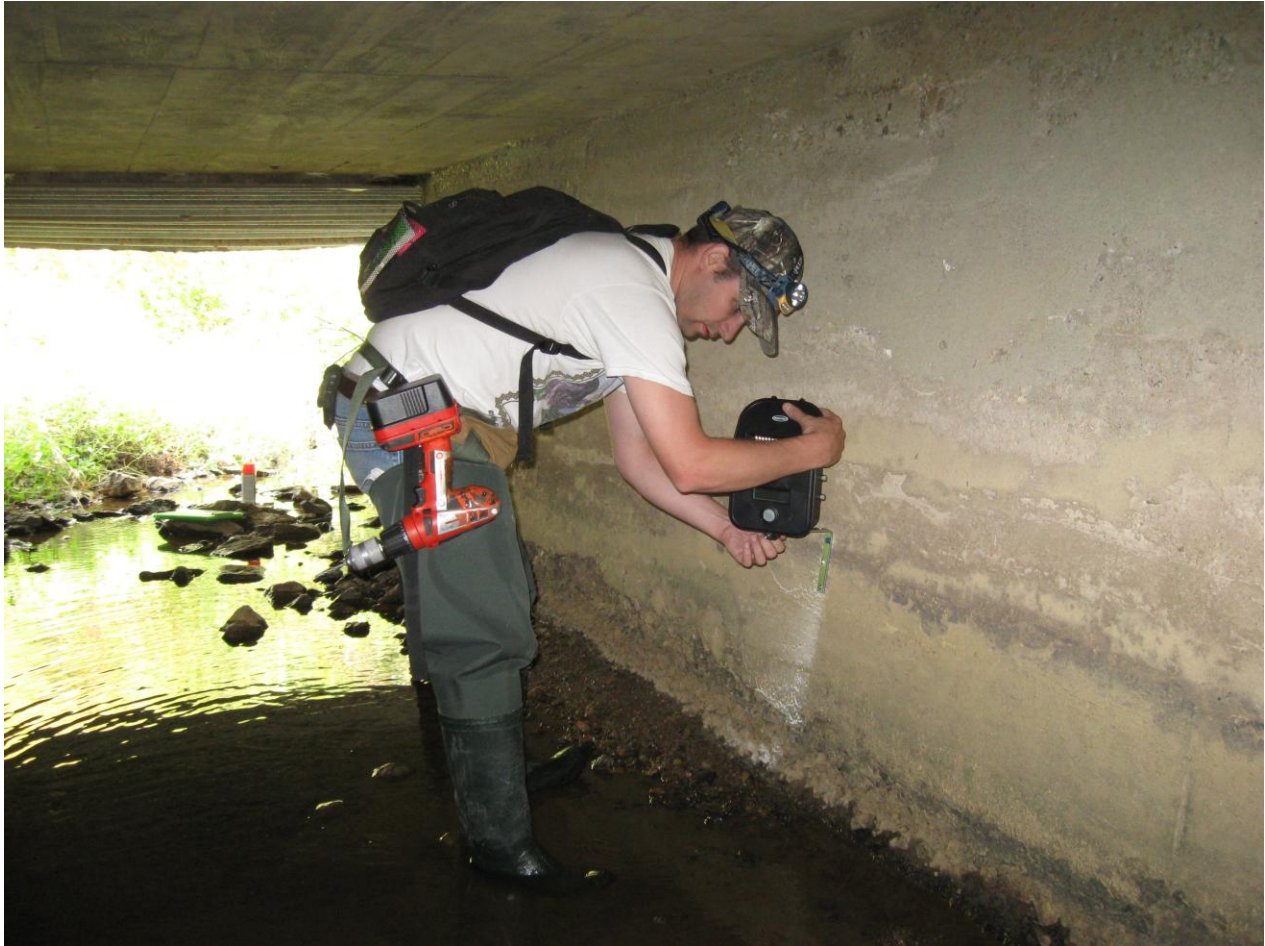
Figure 4. Installation of an infrared, motion-detecting trail camera on an angle bracket in a box culvert.
