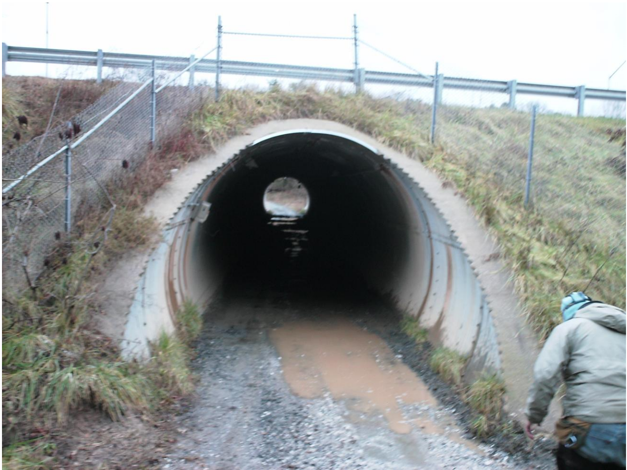
Figure 3. Culvert 02159X0 functions as an equestrian underpass. It is 15 feet (4.5 m) in diameter, 242 feet (73.7 m) long, and essentially dry. This cylinder culvert cell has 5 feet, 10 inches (1.8 m) of type 1 fencing and a gravel substrate.
