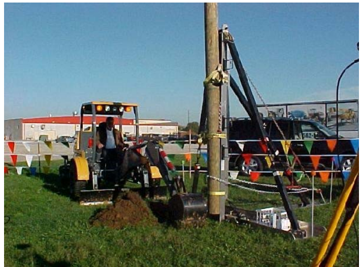
Figure 1: Example of Temporary Pole Brace
