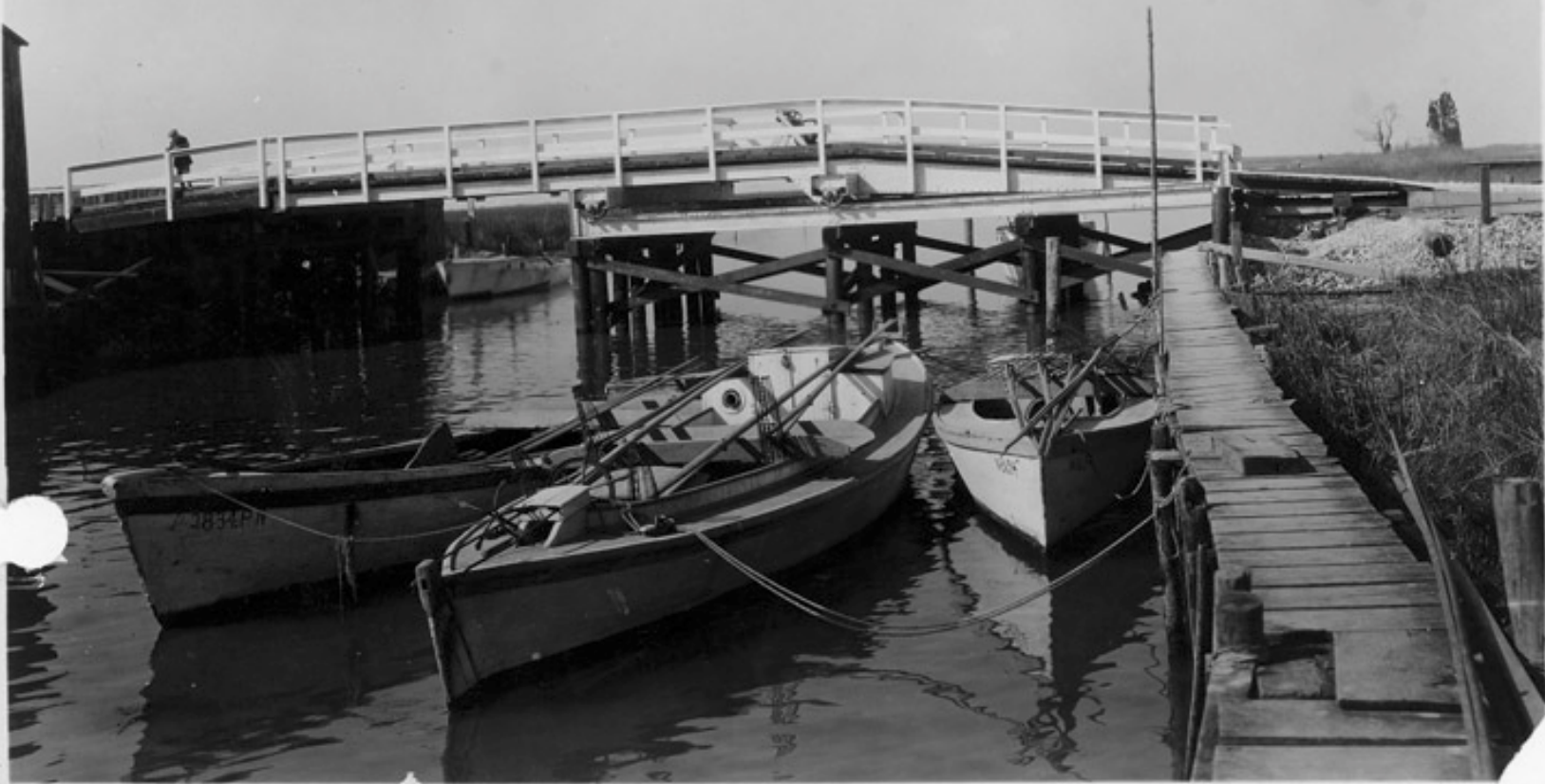
PLATE 9: Rare Retractable Movable Bridge: Bridge Crossing Knapps Narrows at Tilghman Island
