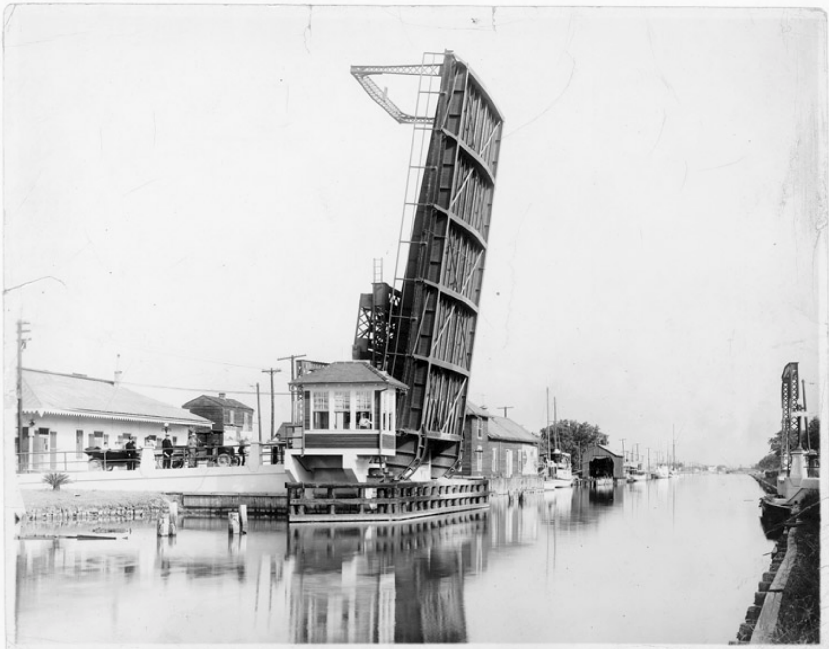
PLATE 8: Typical Single-Leaf Bascule Movable Bridge: Bridge at Kent Narrows
