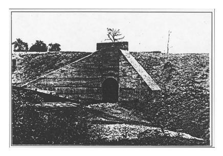
Figure 3.10. 1903 arched concrete culvert ( Source: Maryland Geological Survey 1903: Plate XI, Figure 2).
