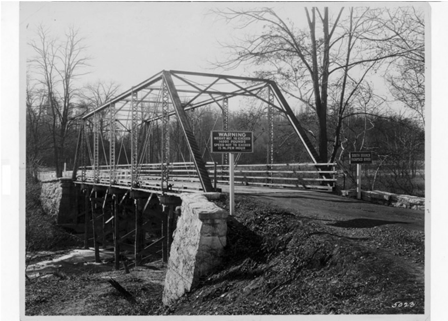
PLATE 5: Typical Metal Pratt Through Truss Bridge: Bridge Crossing the South Branch of the Patapsco River at Henryton
