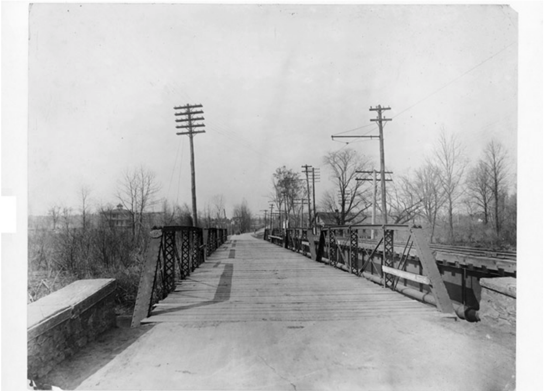
PLATE 6: Typical Metal Multiple-Span Pratt Pony Truss Bridge: Bridge Crossing Winter's Run at Edgewood
