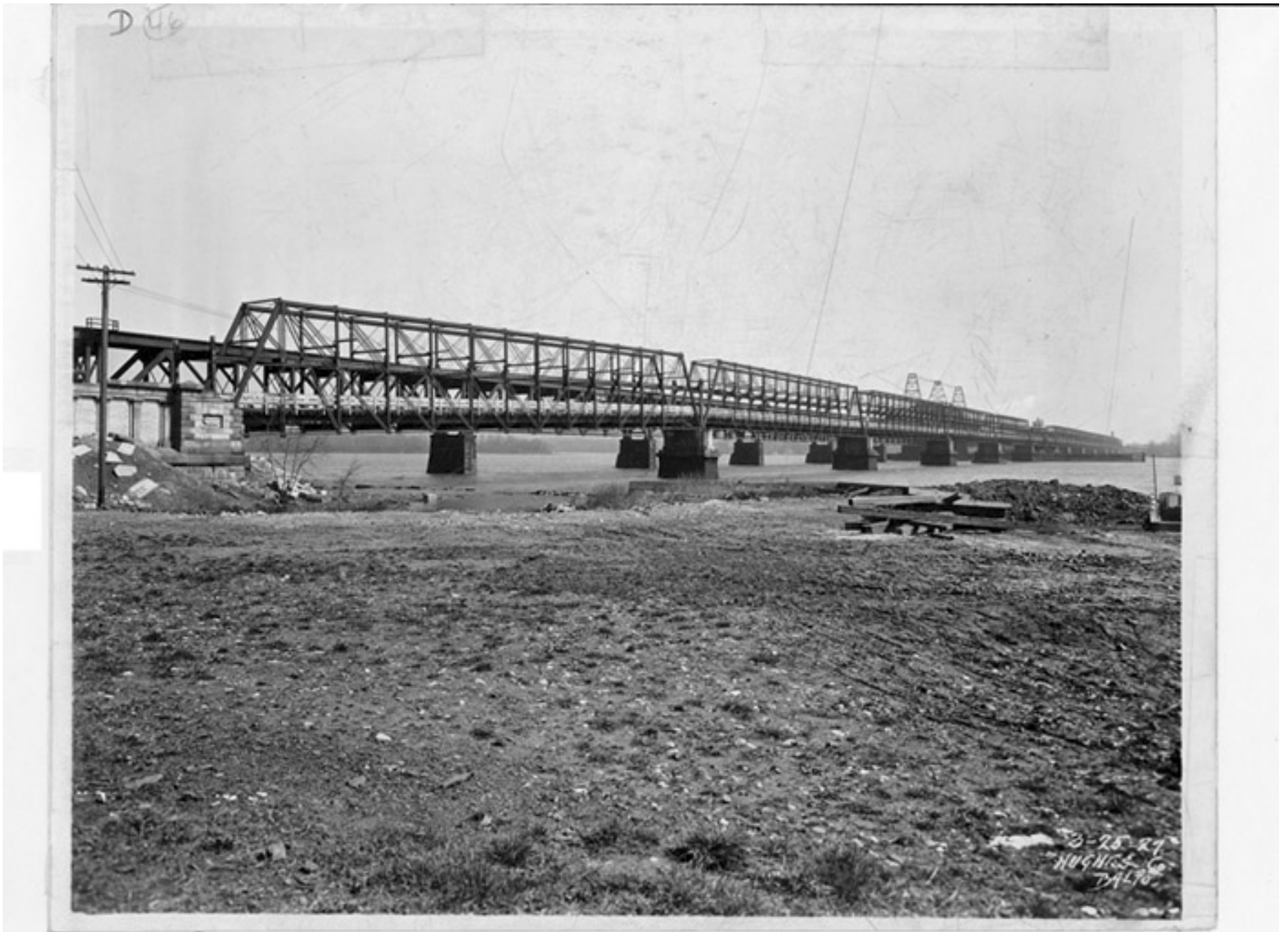
PLATE 7: Typical Metal Double-Intersection Pratt Truss Bridge: Bridge at Havre de Grace
