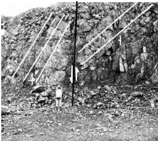
Figure 32. – Fault and associated fracturing within the Lime Kiln Member of the Frederick Formation within the Frederick Quarry. Down-dropped block on the southeast (left) places overturned Lime Kiln against right-side-up, southeast-dipping Lime Kiln in the foot-wall (right). Fracturing to the right of the fault is a combination of both axial planar cleavage and tension fractures associated with the fault.
