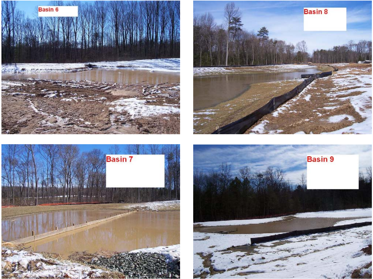
Figure 1. Photos of site basins at construction site MD 43 in Baltimore County, winter 2005.
