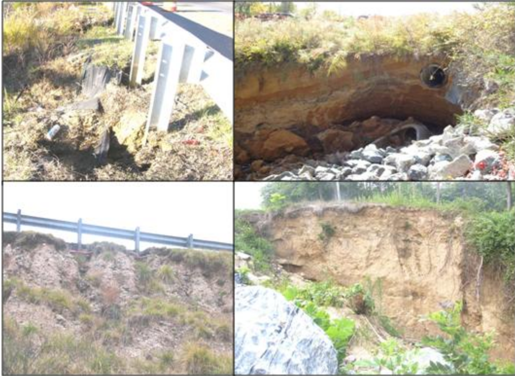
Figure 2.1: A collage of some of the different types of slope failures that have occurred in the State of Maryland
