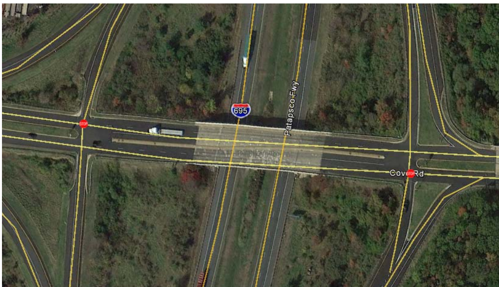
Figure 24. Two “D4” Stop-Controlled Ramp Terminals at Interchange of I-695 and Cove Road
