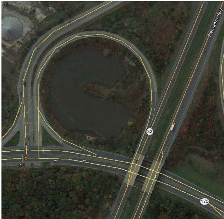
Figure 25. An “A2” Signalized Ramp Terminal at Interchange of Patuxent Freeway (MD-32) and Annapolis Road (MD-175)
