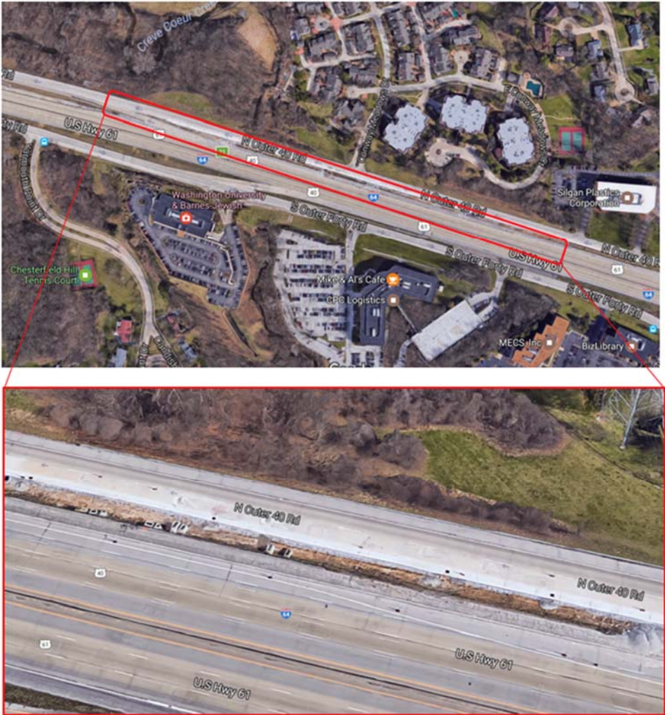
Figure 4-11. Aerial view of the Missouri I-64 evaluation site
