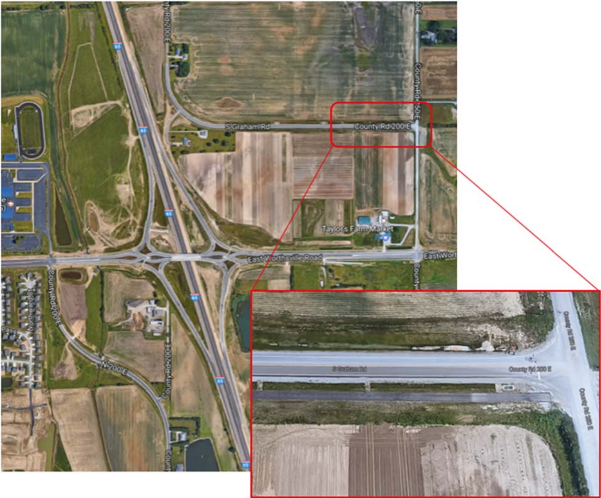
Figure 4-13. Aerial view of the Indiana Graham road evaluation site
