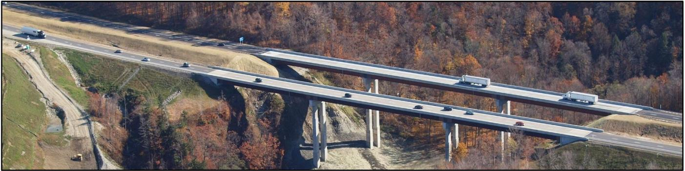
new bridges are a total of 746' long x 48' wide. Fay designed and constructed the 180-foot high piers to support the bridge which are among the tallest in all of Pennsylvania. Each bridge was built with 3,000 CY of substructure concrete, consisting of 50' x 41' spread footers, with 180' tall piers. The deck required 1,600 CY of concrete.
