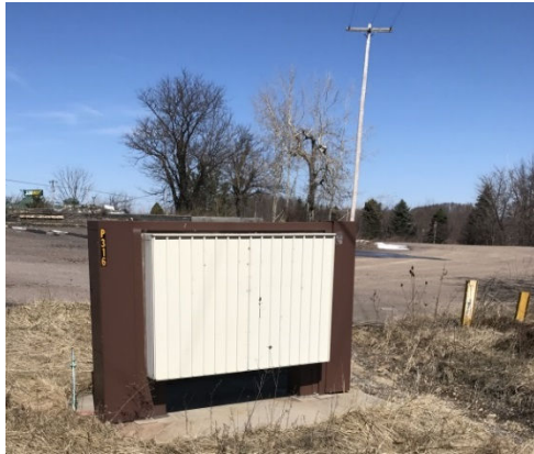
Above is the switch box on US 40 Alt
