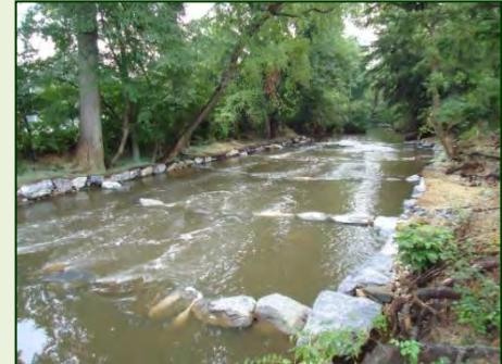
are constructed out of large imbricated riprap to create safe areas for fish to spawn and provide at least one foot of water flow over fish blockages within Rock Creek.
