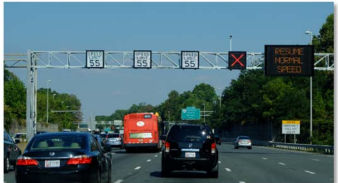
VDOT D-B I-66 ATMS designed by Parsons Brinckerhoff
