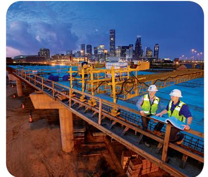
**The Houston METRO Light Rail Expansion DB** included three new corridors, totaling approximately 15 miles of double-track LRT, 23 stations, storage and inspection facilities, system safety and operational upgrades to the existing 7.5-mile LRT system, 58 new light rail vehicles, a new operations control center, and major renovations to the existing operations control center to allow it to operate as a backup.
