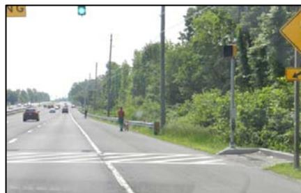
existing MD 4 will be reclassified as an Urban Other Principal Arterial and posted at 45mph. The north and southbound roadways will be closed and narrowed to 34-feet (2 – 11ft travel lanes, a 4-ft inside shoulder and an 8-ft outside shoulder) to force the motorists to slow down through the project limits.
