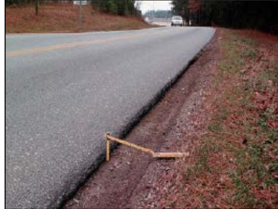
Figure 4.5 Shoulder Drop Off Source: FHWA "Safety Edge" Brochure
