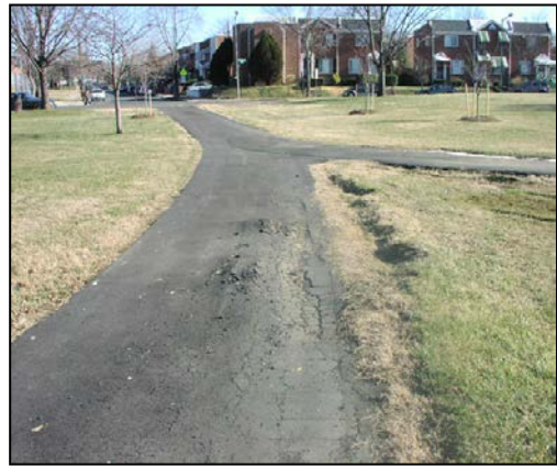
Figure 7.3 - Poorly Designed Trail Surface
