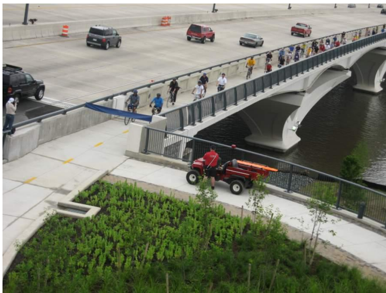
Figure 8.2 Woodrow Wilson Bridge Trail
