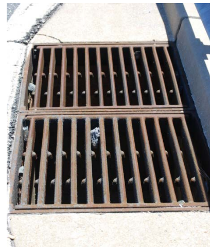
Figure 4.6 Non-Compliant Inlet Grate
