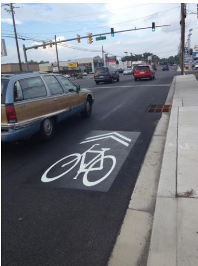
Figure 3.2 Shared Lane Marking (Sharrow) U.S. 113 in Salisbury
