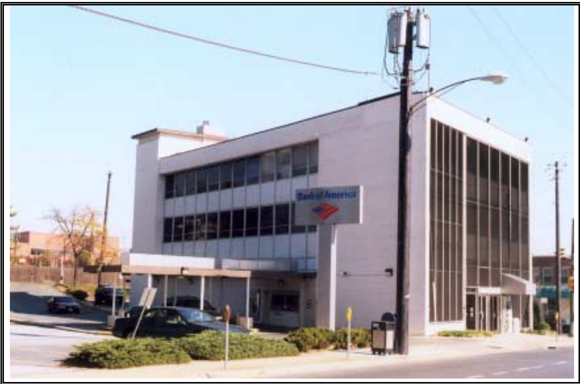
Plate 28: Office Building (Bank of America, 2601 University Boulevard, Wheaton, Montgomery County)
