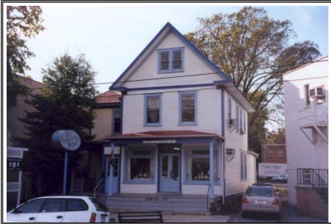
Plate 23: Vernacular Commercial Building (10410-10414 Howard Avenue, Kensington, Montgomery County)
