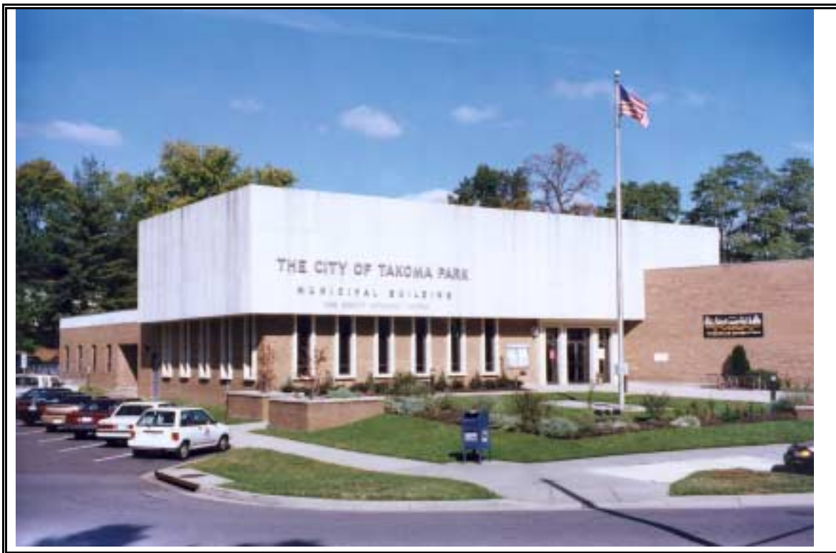
Plate 31: Municipal Building (Maple Avenue, Takoma Park, Montgomery County)
