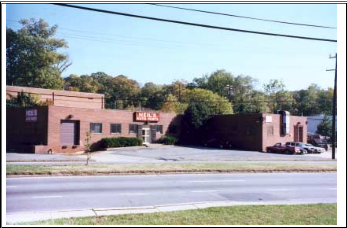
Plate 25: Industrial Building (Kenilworth Avenue, Edmonston, Prince George's County)
