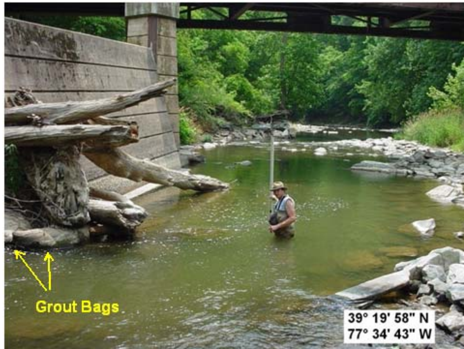
Photo 89: Scour hole (4.5' deep) and grout bags (left) at Pier D.
