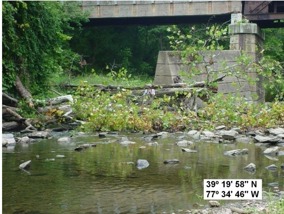
Photo 92: Debris collected at wall in front of Pier D.
