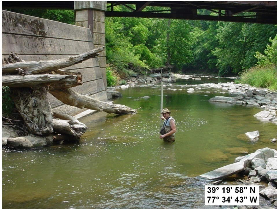
Photo 89: Looking downstream, scour hole at retaining wall above Pier D, pool depth 4'.
