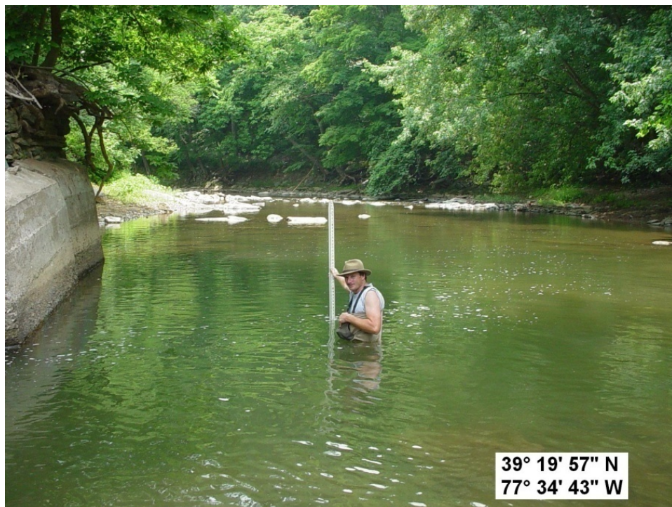
Photo 69: Scour hole (>5.5' deep) at old bridge abutment.
