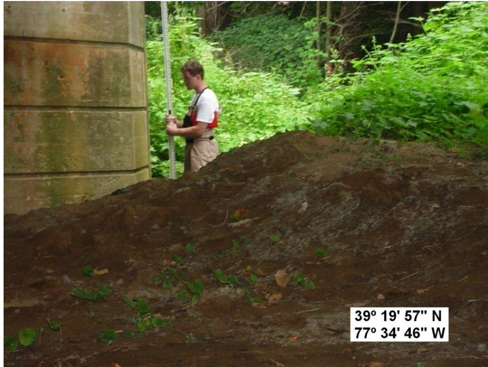
Photo 83: Scour at Pier B and deposition in the B-C span.
