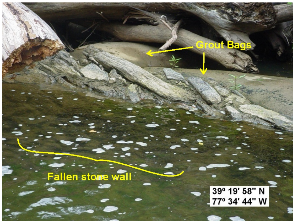
Photo 91: Broken stone wall and grout bags at upstream wall of Pier D.
