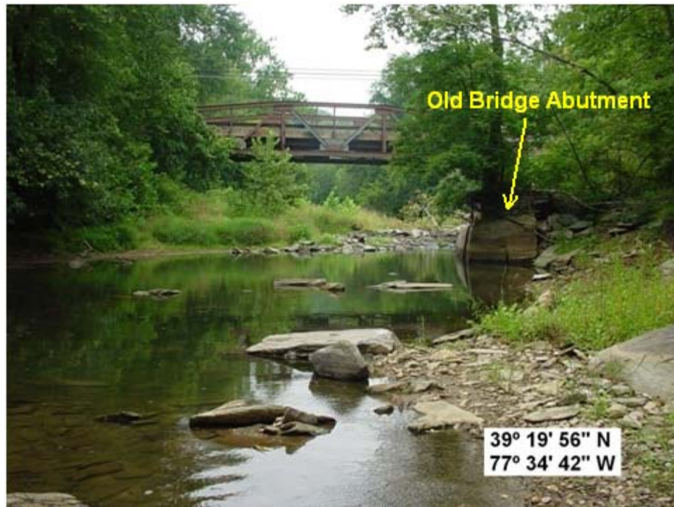
Photo 67: Looking upstream, old bridge abutment (with 5.5' deep scour hole) on right receiving majority of flow redirected by MD 464 Pier D
