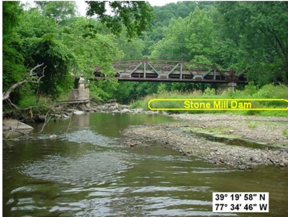
Photo 101: Approach flows constricted by 6' high stone mill dam on right (in vegetation) and high banks with debris jam on left.
