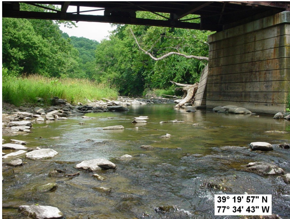
Photo 74: Remnants of stone mill dam compose substrate for LFHG feature at MD 464 Bridge.
