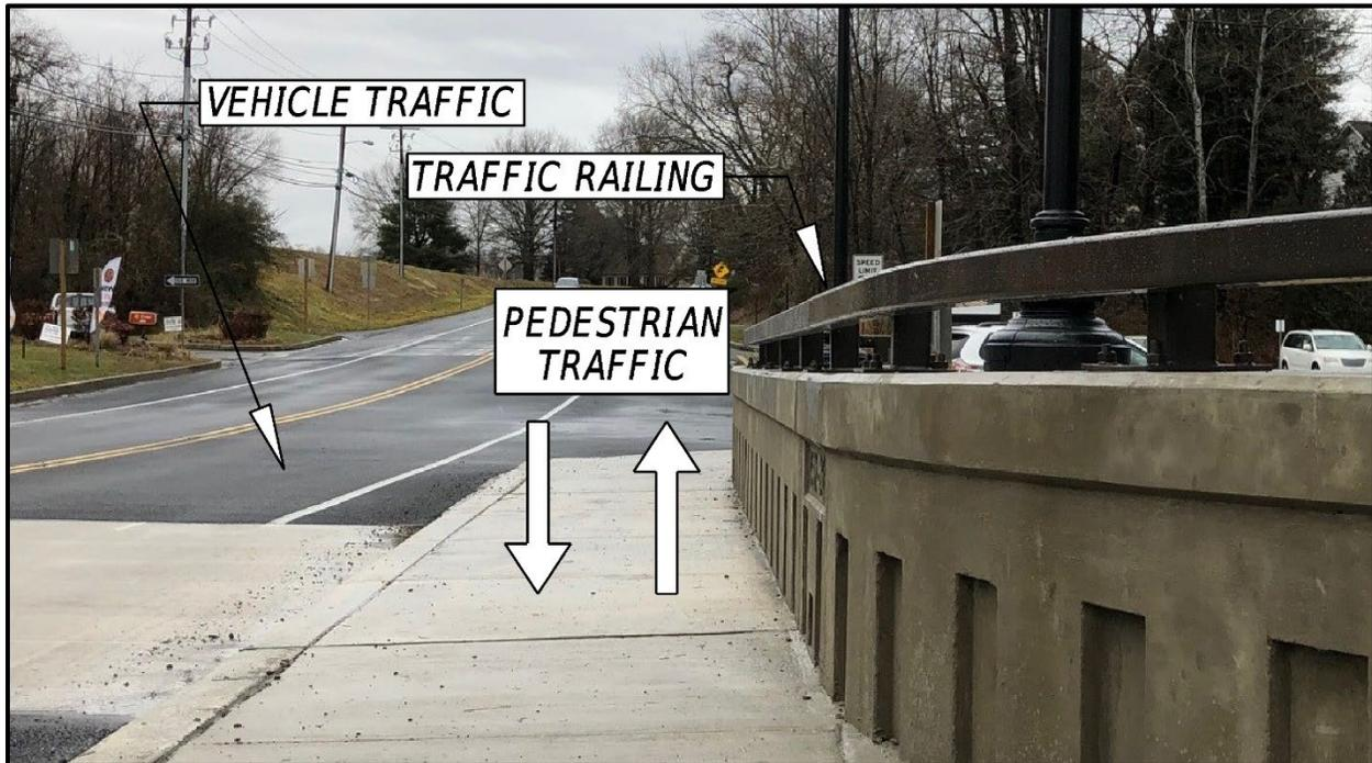
*Figure 2-2: Low-Speed Roadway with Pedestrian Facility*
