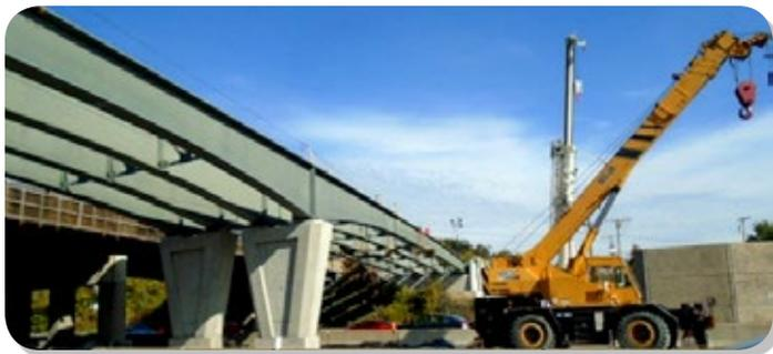
*Setting new steel beams for the Old Harford Road Bridge as part of the I-695 between MD 41 and MD 147 interchange reconstruction project*
