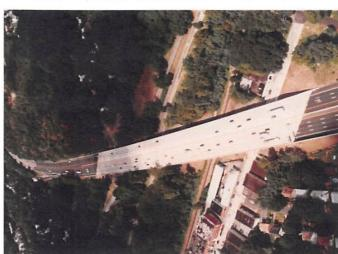
**Belt Parkway and Interchange over Ocean Parkway.** This project involved demolition of the existing bridge and replacement while managing more than 160,000 vehicles per day; using an innovative "Inverset" Bridge System. The interchange and Bridge replacement project resulted in additional lanes, shoulders and significant span increase to augment future traffic congestion relief.
