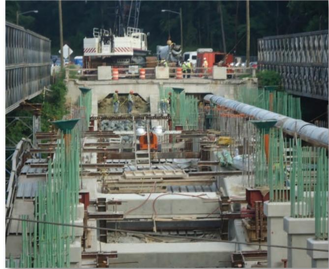
**US 1 (Washington Blvd.) Bridge over CSX Transportation – Baltimore County – \$34.0 million:** This project replaces the bridge over the rail tracks, and the new structure will be 120 feet longer and 4 feet higher to enable CSX Transportation to add future rail lines, a rail service road and added height to allow for double stacked freight cars. The wider structure will provide wide shoulders, as well as a
