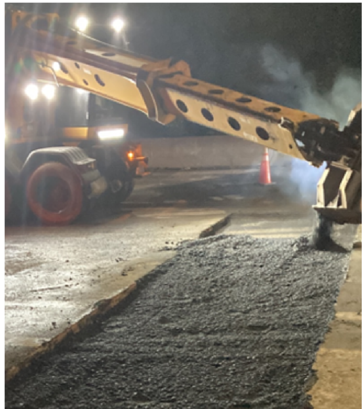
Crews applying asphalt lifts after filling in the void under I-97 Anne Arundel County
