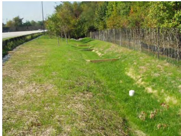
Dry swale after construction
