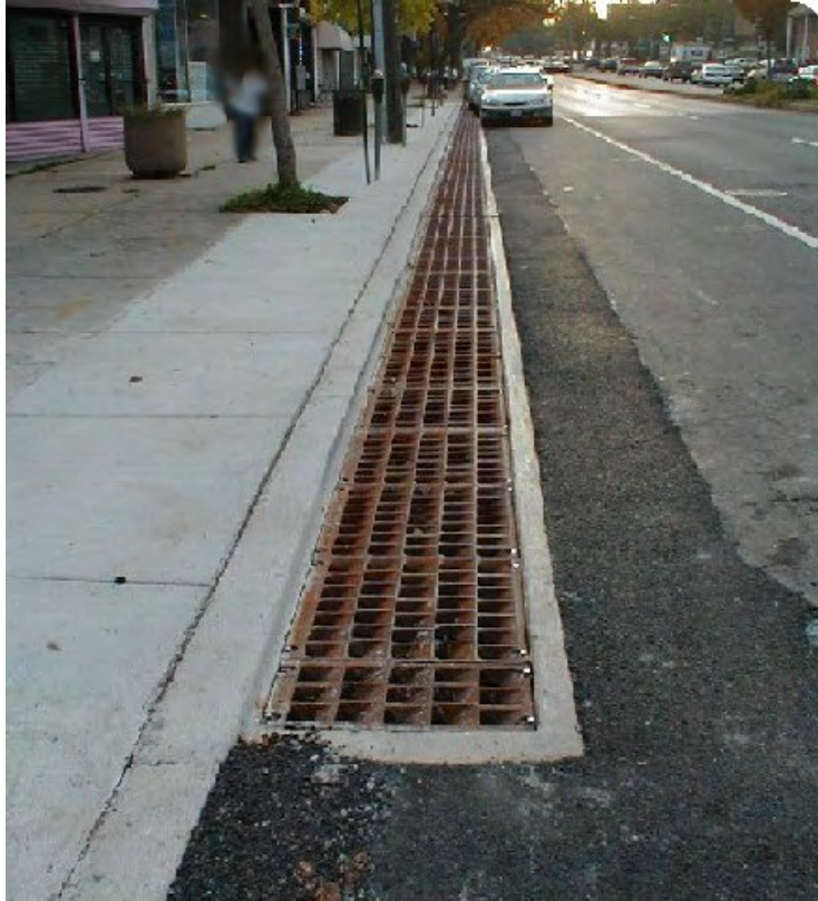
Figure 12. Completed gutter filter, fall 2003.
