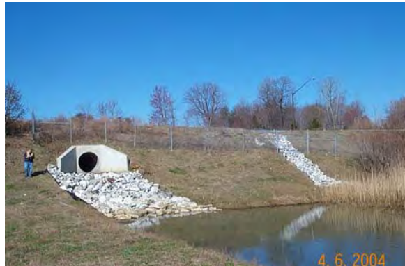
Photo 6 – 60" RCP inflow and 3' curb opening and riprap channel inflow on the west side of the BMP
