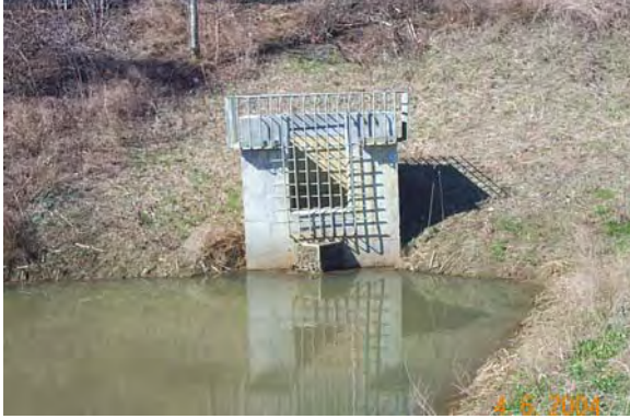
Photo 7 – Control structure with trash rack on the south west side of the facility
