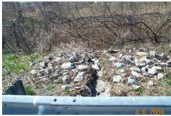
Photo 17 – Erosion around and in the riprap inflow on the north side of the facility
