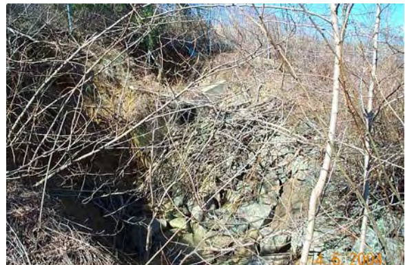
Photo 10 – Damaged headwall to the 30" RCP inflow
