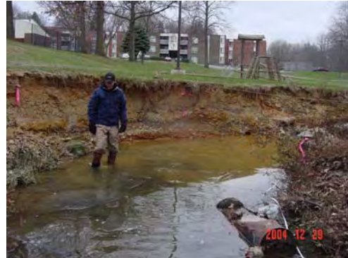
Study Reach D showing channel migration and high bank erosion area.
