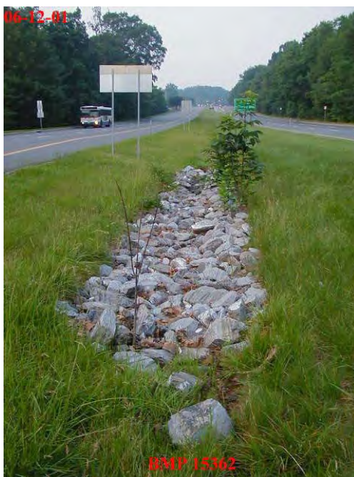
Figure 7. Example of an infiltration trench located in Montgomery County, MD.
