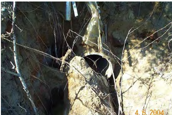
Photo 11 – Separated 30" RCP pipe causing heavy erosion
