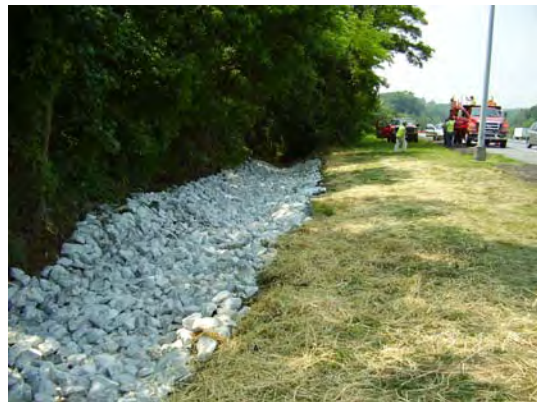
Figure 3-4: Installation of Infiltration Trench Monitoring Well and Media Replacement
