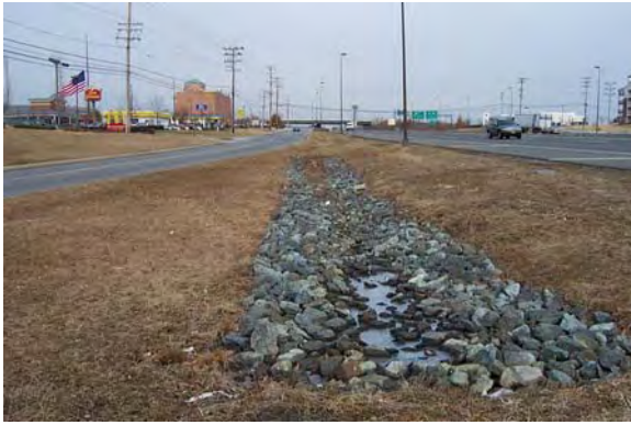
Infiltration trench at US 301
