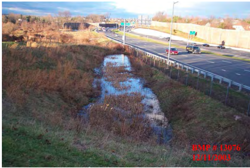
Figure 3. Example of a shallow marsh BMP located in Howard County, MD.
