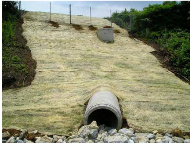
Figure 3-3 SWM Pond Slope Stabilization
