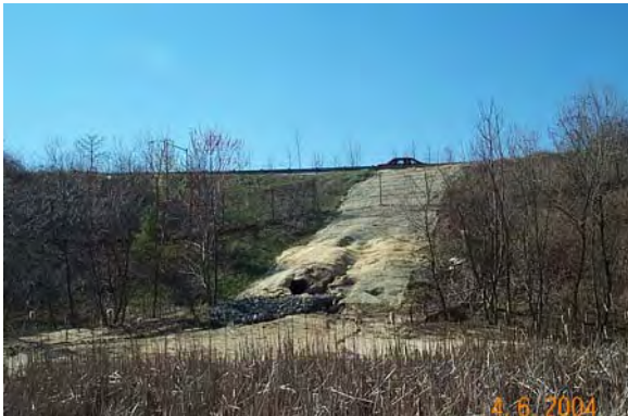
Photo 5 – 27" HDPE pipe inflow with unstable slope on the south side of the facility
