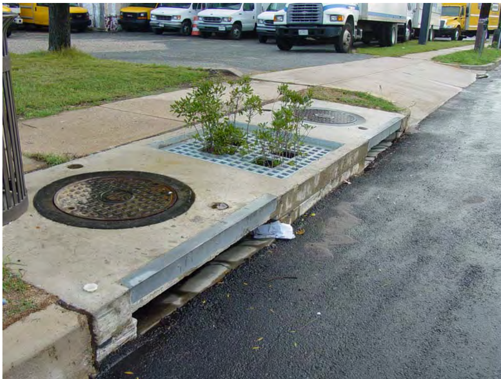
Figure 13. Completed bioretention inlets, fall 2004.
