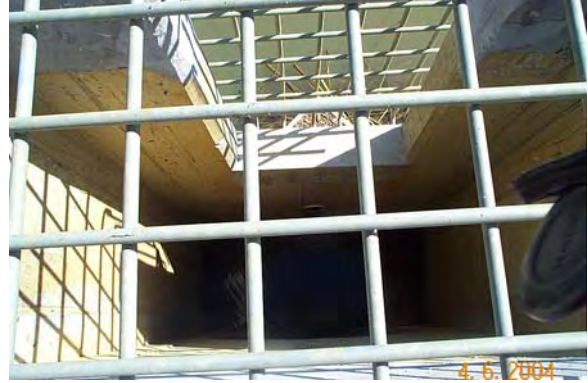
Photo 8 – Control structure interior
