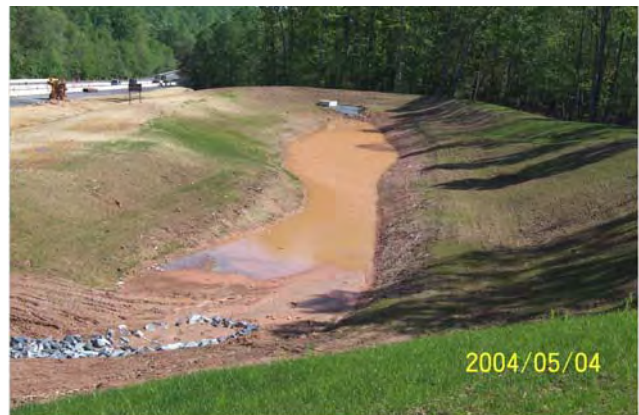
Example of Sediment Basin (from SHA BEST Training Material)
