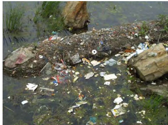
Litter and debris accumulated in a SWM BMP.
