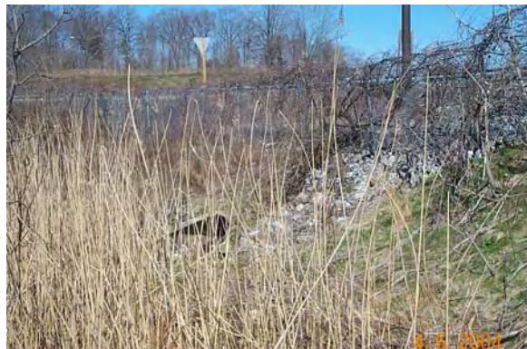
Photo 16 – 36” RCP inflow and a riprap inflow on the north side of the facility
