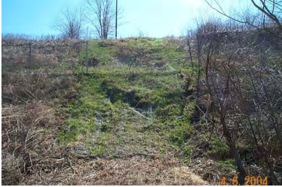
Photo 13 – Fence gap and failing slope on the south east side of the facility
