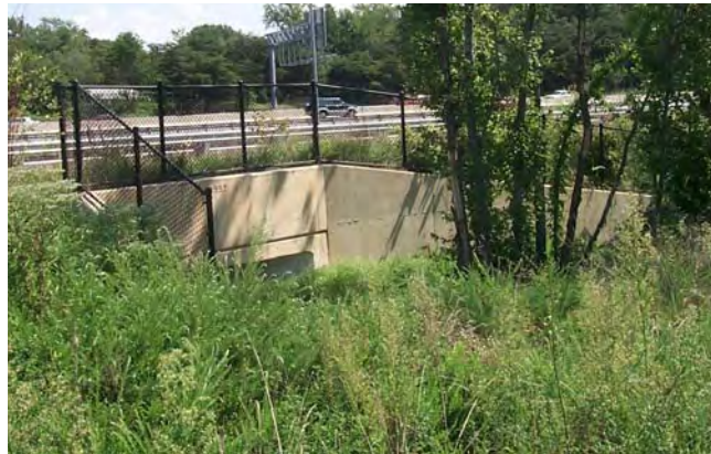
Figure 7. Chain Link Railing at Endwall
