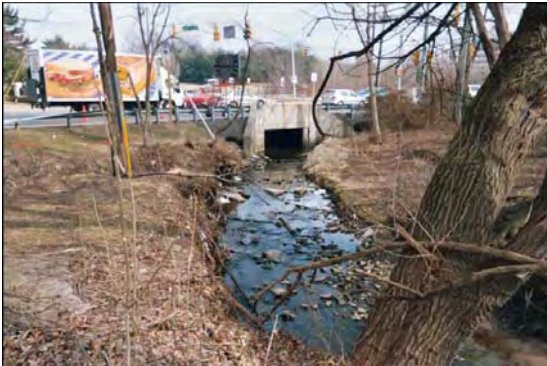
Upstream Project Limit – MD 117, Clopper Road Crossing
