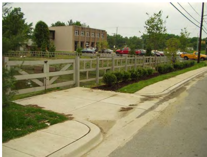
Figure 9. Concrete Apron Provided at Maintenance Access
