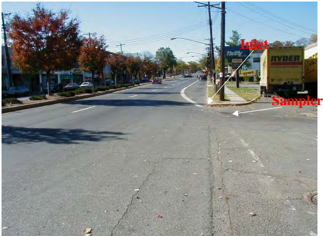
Figure 2. Stormwater monitoring site at Mt. Rainier with samplers below grade.
