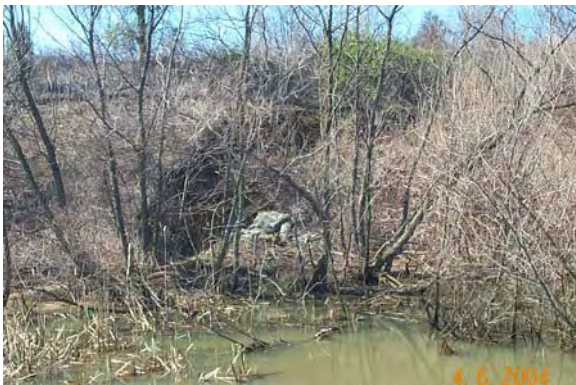
Photo 9 - Heavy erosion around broken 30" RCP inflow on the south side of the BMP
