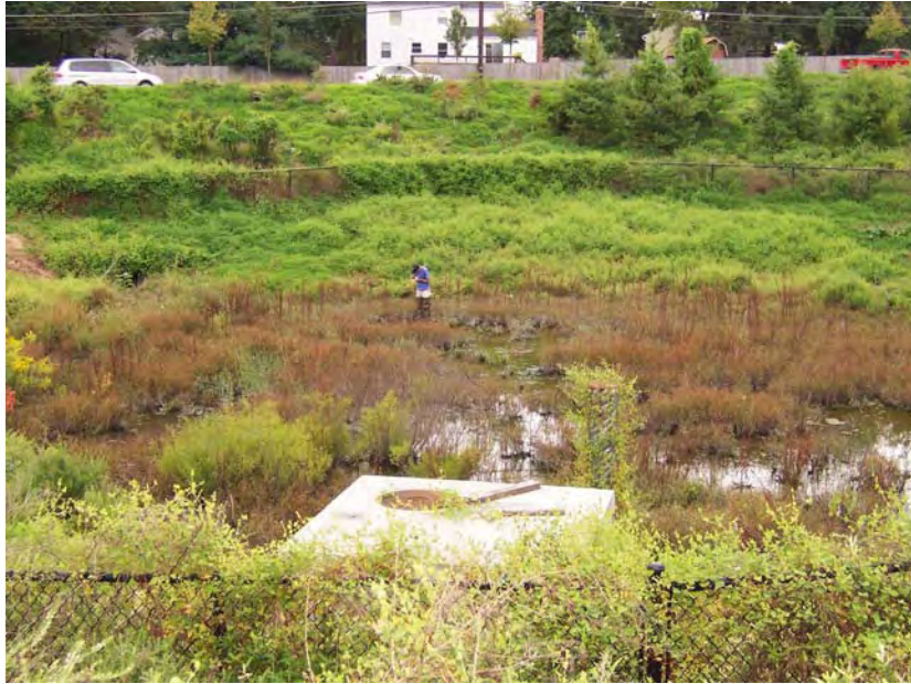
Figure 5. Example of a detention pond BMP located in Montgomery County, MD.
