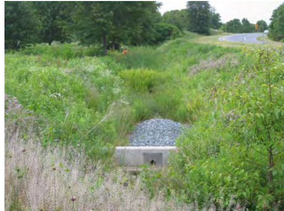
Dry Swale in Howard County during Field Inspection
