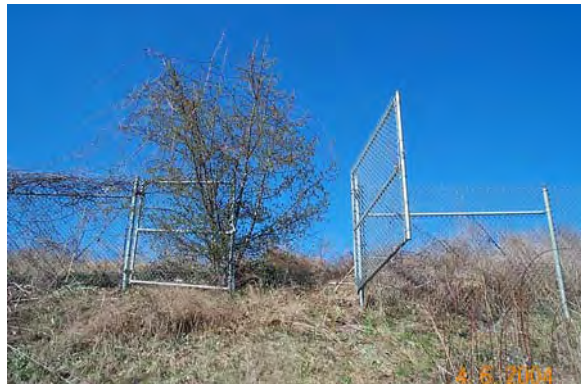
Photo 4 – Steep slope with a tree at the entrance with no chain and lock on the west side of the BMP
