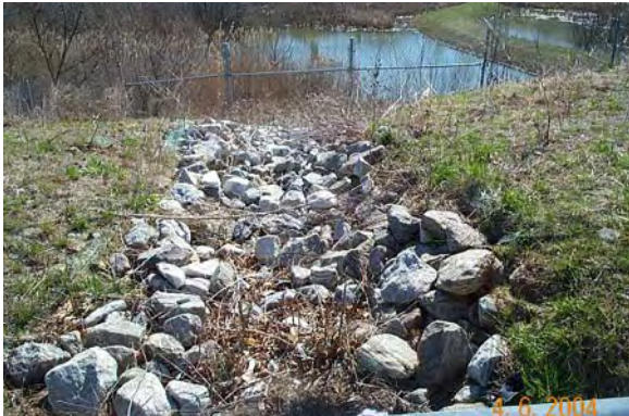
Photo 1 – Debris in the riprap from the curb opening on the west side of the facility
