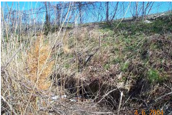
Photo 15 – Heavy trash and sediment in the area of the 18” RCP inflow on the north side of the BMP
