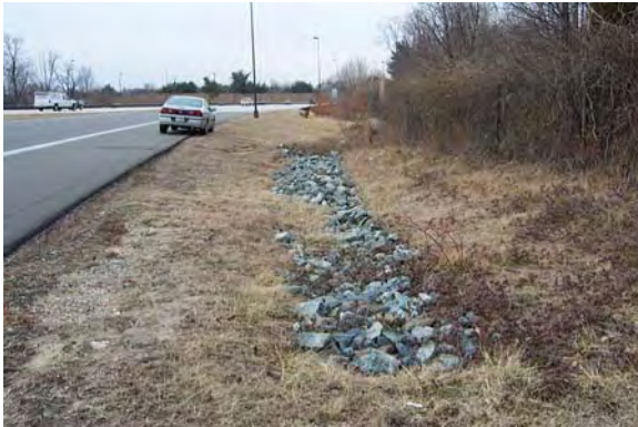
Infiltration trench at US 301
