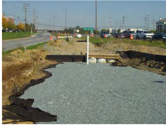
Bioretention under construction
