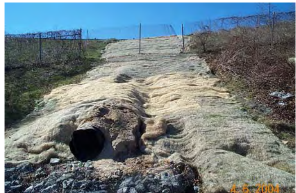
Photo 12 – 27" HDPE pipe inflow and recently regraded slope on the south side of the BMP
