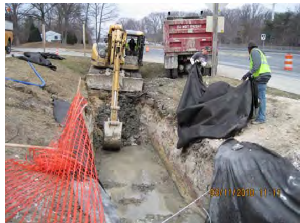
Figure 2-3 Removal of Sediment from Infiltration Trench and Media Replacement in Harford County (BMP 120063)
