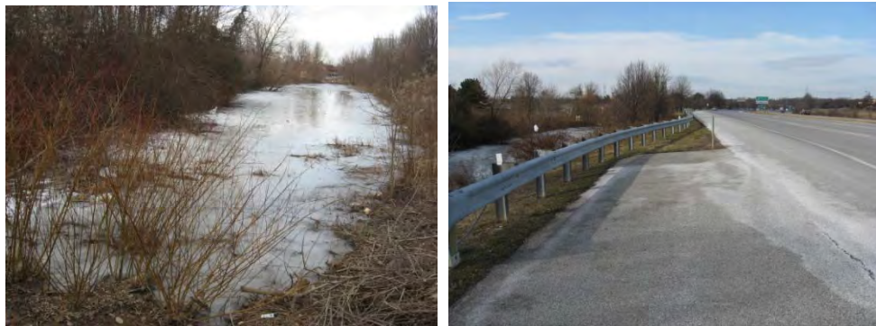
Figure 20. Sample chloride concentrations during the Jan 17, 2010 event at the study site. Photographs show the frozen BMP (left) and adjoining highway (right), one day prior to the event.
