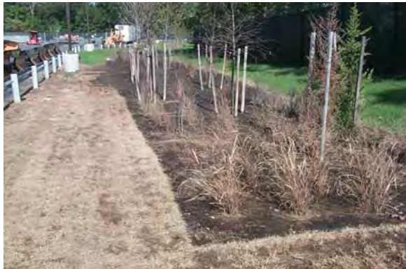
Figure 2-15 Failed Bioretention at SHA Glen Burnie Maintenance Shop
