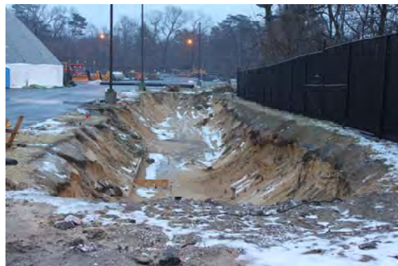
Figure 2-18 Construction progress of Sand Filter Installation at SHA Glen Burnie Maintenance Shop
