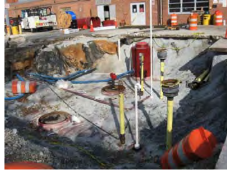
Underground Storage Tank System Upgrades
