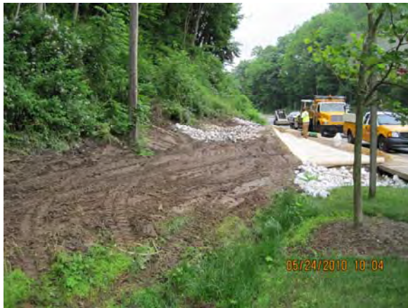
Figure 2-9 Example of SHA Actions to Prevent Off-site sedimentation source from contaminating downstream Infiltration Practice
