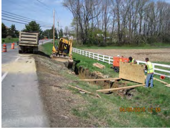
Figure 2-4 Infiltration Trench Replacement in Harford County (BMP120039)
