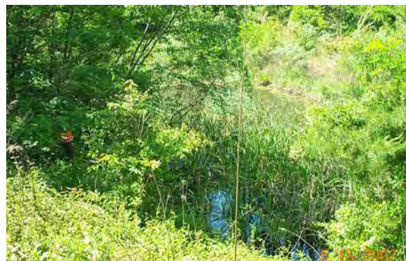
Figure 2-7 Infiltration Basins in Howard and Anne Arundel County Functioning as Wetland/ Wet SWM Facilities - Suggested Retrofits by Nature
