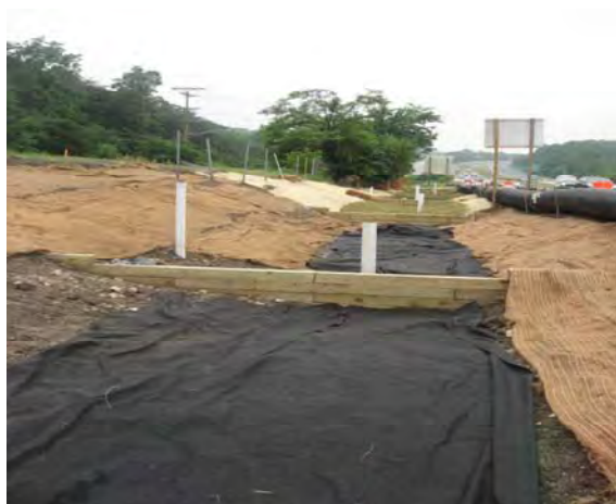
Figure 2-13 Construction of Retrofit of Failed Infiltration Trenches into Dry Swales at I-97
