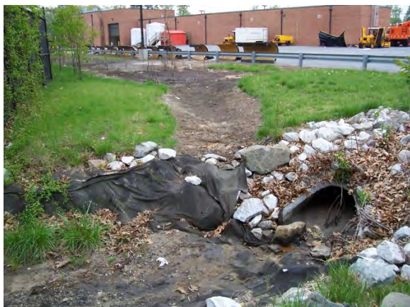
Figure 2-16 Deteriorated outfall at SHA Glen Burnie Maintenance Shop
