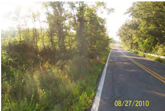
Figure 2-5 Infiltration Trench Replacement in Prince Georges County (before)
