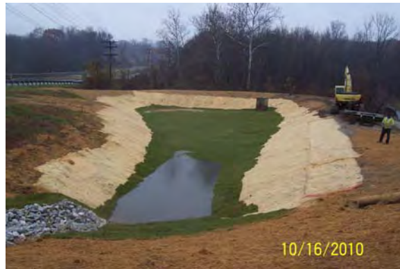
Figure 2-12 Infiltration Basin Remedial Activities completed
