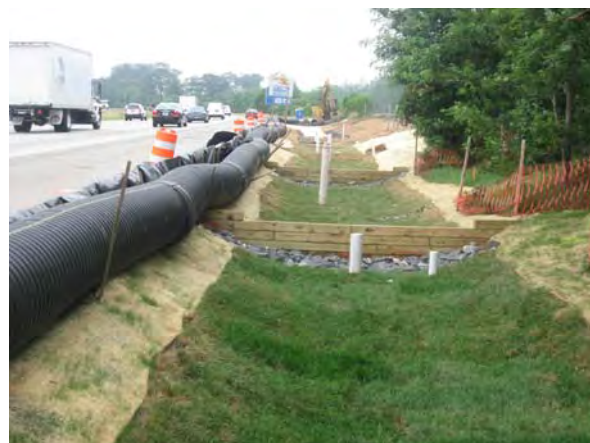
Figure 2-14 Construction of Retrofit of Failed Infiltration Trenches into Dry Swales at I-97
