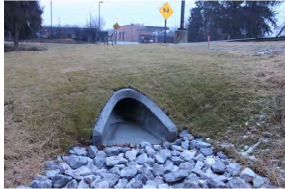
Figure 2-17 Improved outfall at SHA Glen Burnie Maintenance Shop
