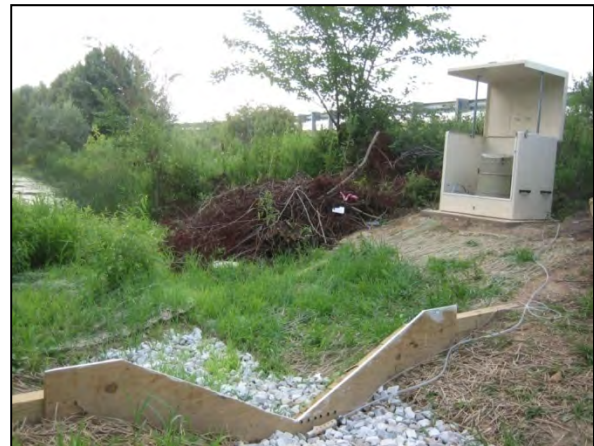
Instrumentation at Failed Infiltration Basin No. 130348
