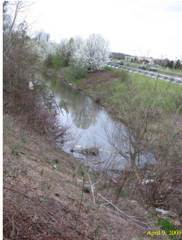
Figure 4. BMP 13348 located along MD 175 EB. Photo, looking west, shows single concentrated inflow point to the BMP. Some additional flow will occur from sides of the BMP.
