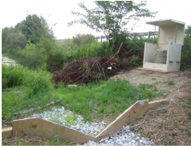
Figure 6. Photo showing the sampler and weir installed at the inlet side of the BMP.
