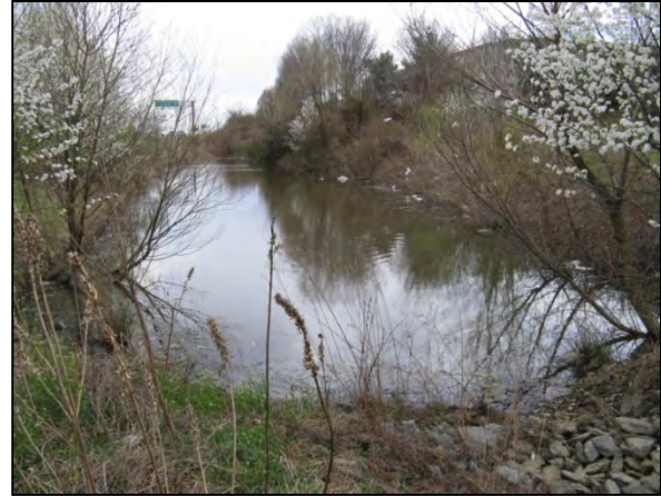
View of BMP 130348 at Outflow Point – Failed Infiltration Basin Currently Monitored
