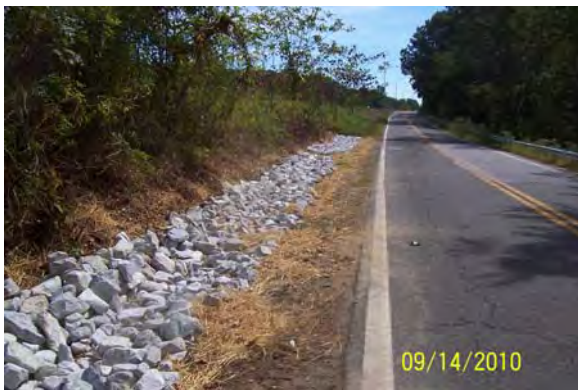
Figure 2-6 Infiltration Trench Replacement in Prince Georges County (after)
