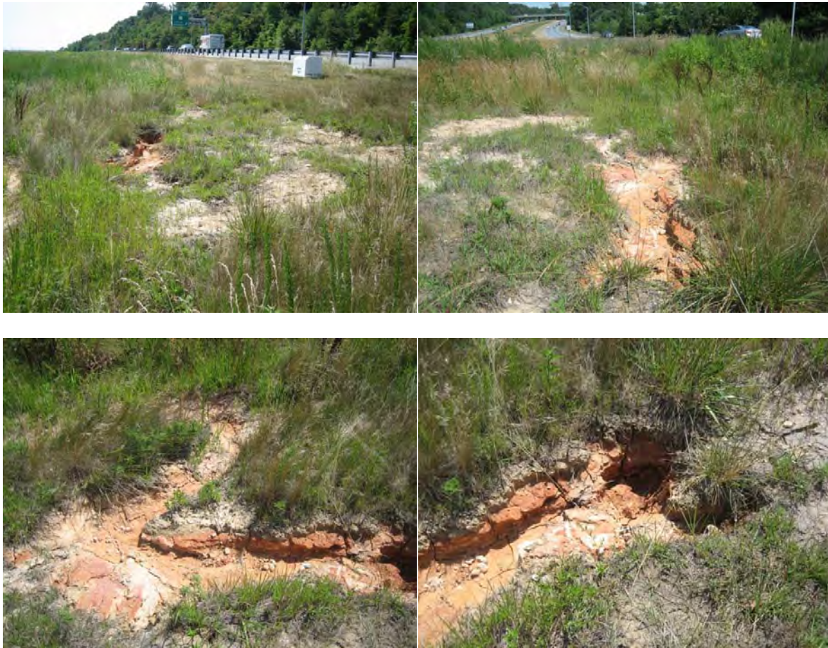
Figure 10. Pits caused by erosion near direct channel
