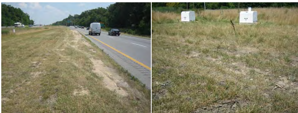
Figure 2. Bare spots on pretreatment area of MDE swale.
