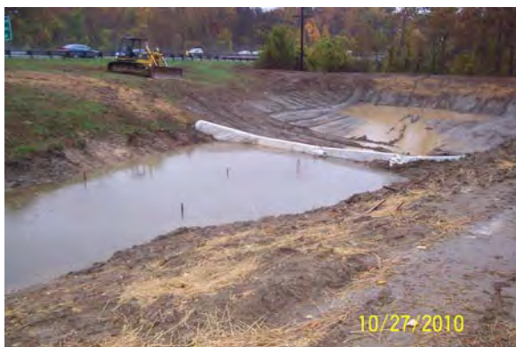
Figure 2-11 Existing Infiltration Basin during Remedial Activities
