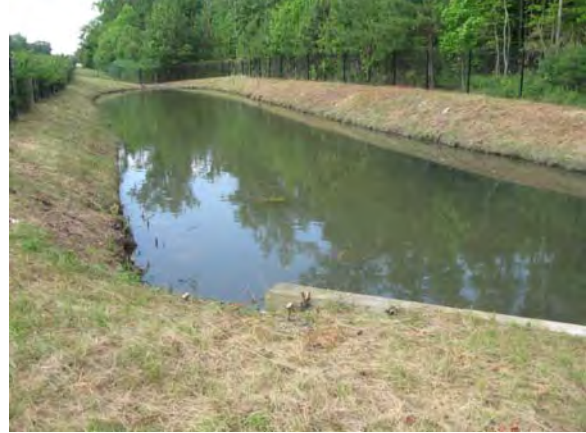
Figure 2-2 Minor Maintenance Activities BMP 080069 After Maintenance
