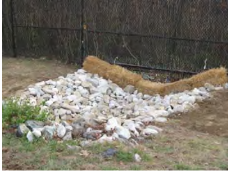
Storm Water Outfall Improvements at SHA Maintenance Shop
