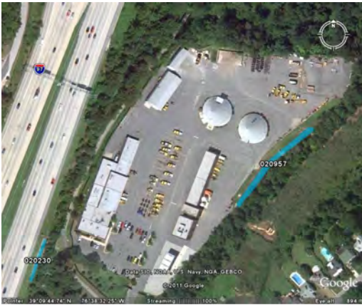
Figure 2-11: Glen Burnie Maintenance Shop Retrofit Project Location
