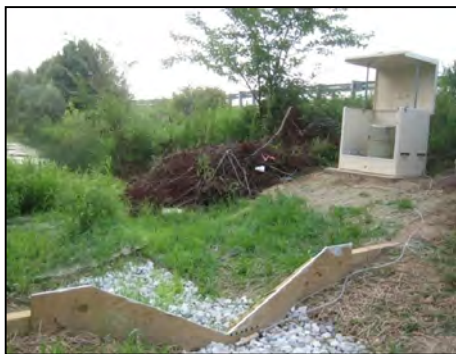
Figure 1-9: Instrumentation at Failed Infiltration Basin No. 130348
