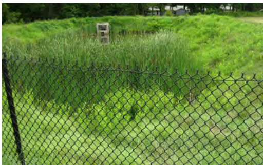
Figure 2-3: Minor Maintenance Activities BMP 080065 Before Maintenance
