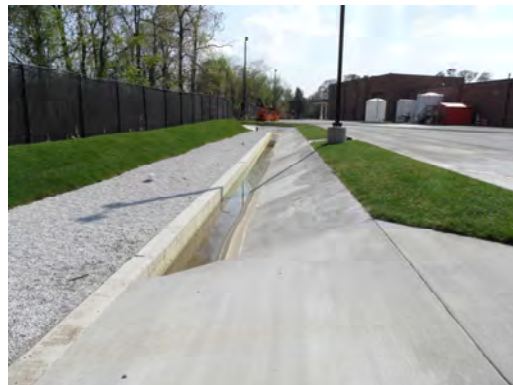
Figure 2-13: Sand Filter Installation at SHA Glen Burnie Maintenance Shop –After Construction
