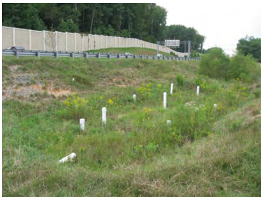
Figure 2-11: Sand Filter (BMP130259) Before Maintenance, Howard County
