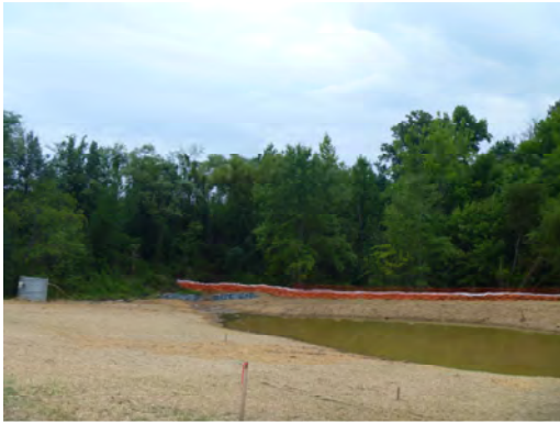
Figure 2-14: MD 4 SWM Functional Enhancement Project During Construction
