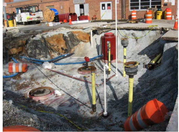
Figure 1-17: Underground Storage Tank System
