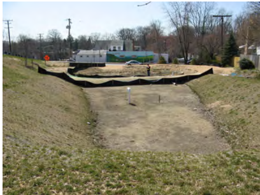
Figure 2-7: Sand Filter Maintenance (BMP030035) Baltimore County
