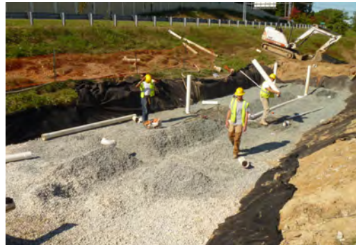
Figure 2-12: Sand Filter (BMP130259) During Maintenance, Howard County
