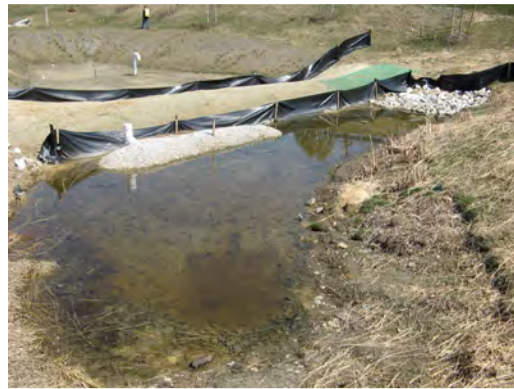
Figure 2-8: Sand Filter Forebay Before Maintenance (BMP030035) Baltimore County
