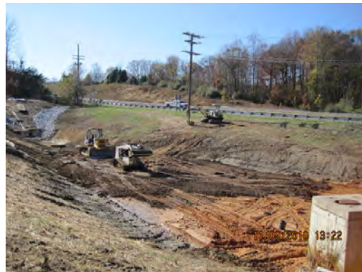
Figure 2-5: Removal of Sediment from Infiltration Basin in Howard County (BMP 130316)
