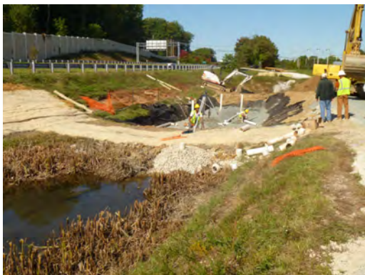
Figure 2-10: Sand Filter (BMP130259) During Maintenance, Howard County
