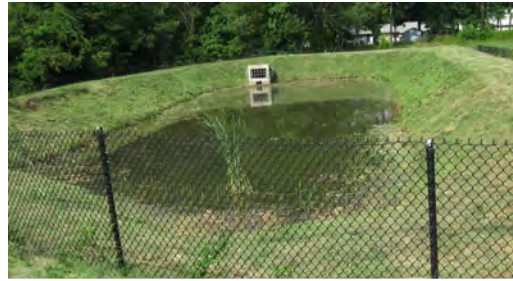
Figure 2-4: Minor Maintenance Activities-BMP 080065 After Maintenance
