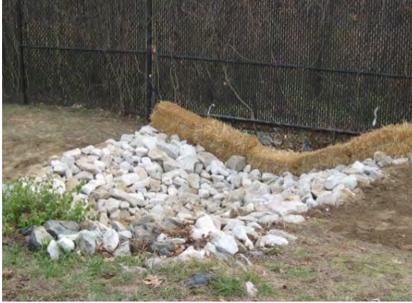
Figure 1-16: Stormwater Outfall Improvements at SHA
