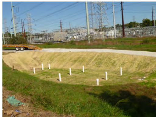
Figure 2-13: Sand Filter (BMP130258) After Maintenance, Howard County
