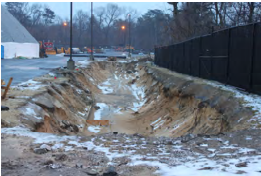
Figure 2-12: Sand Filter Installation at SHA Glen Burnie Maintenance Shop – During Construction
