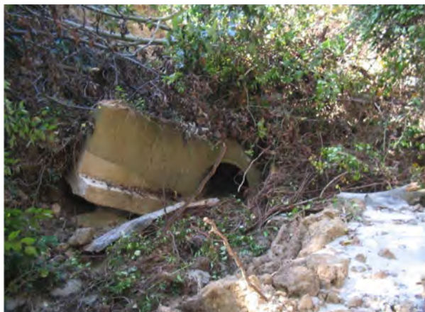
Figure 1-21: Inspected outfall along MD 4
