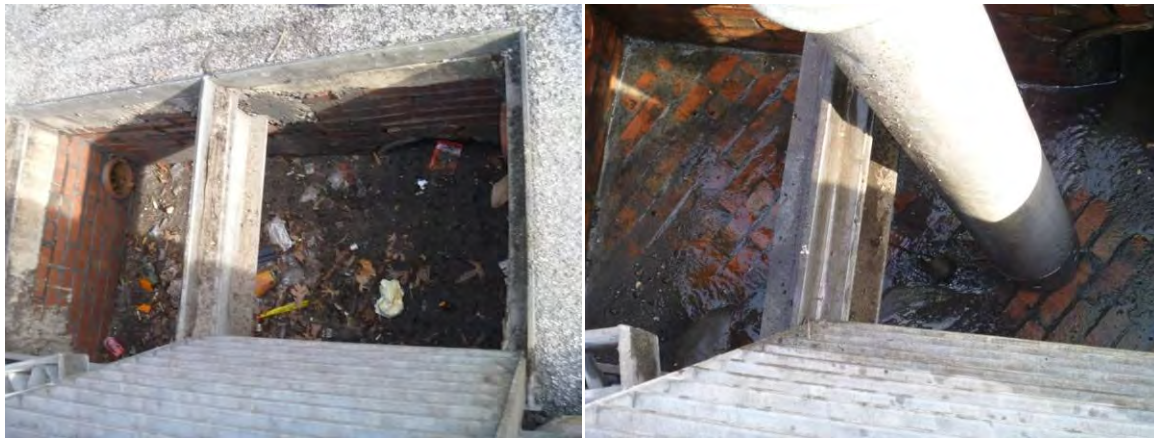
Figure 1-17: Inlet Before and After Vacuuming
