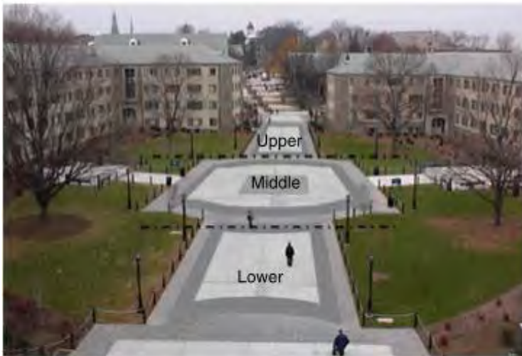
Figure. 3-12. Photograph of Villanova University of permeable pavement infiltration bed system in courtyard documented in Horst et al. (2011).
