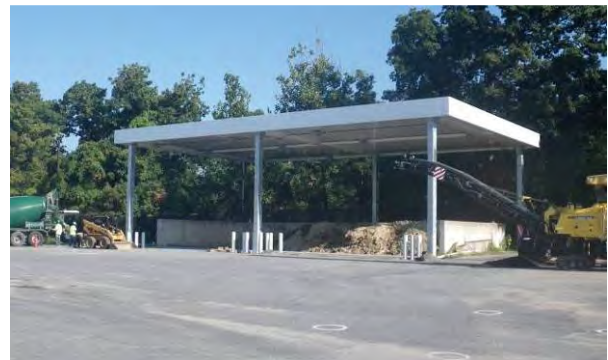
Figure 1-18: Structure used for Inlet Cleaning Waste Dewatering
