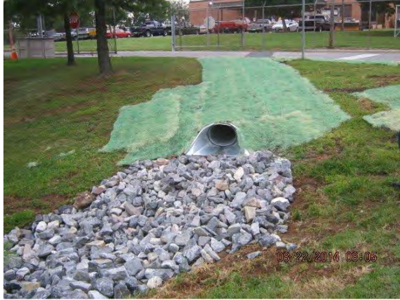
Figure 1-19: Stormwater Outfall Improvements at SHA Maintenance Shop
