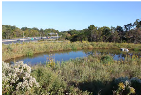
Figure 1-33: MD 147 and I-695 SE Loop – SWM Water Quality Retrofit Project – a year after construction
