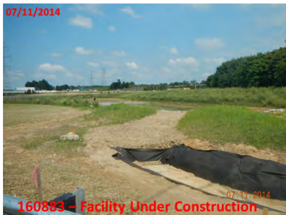
Figure 2-4 – SWM Facility 160883 Under Retrofit Construction
