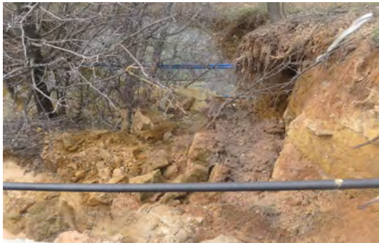
Figure 1-24: I-450 at US 50 Outfall Stabilization Before Construction
