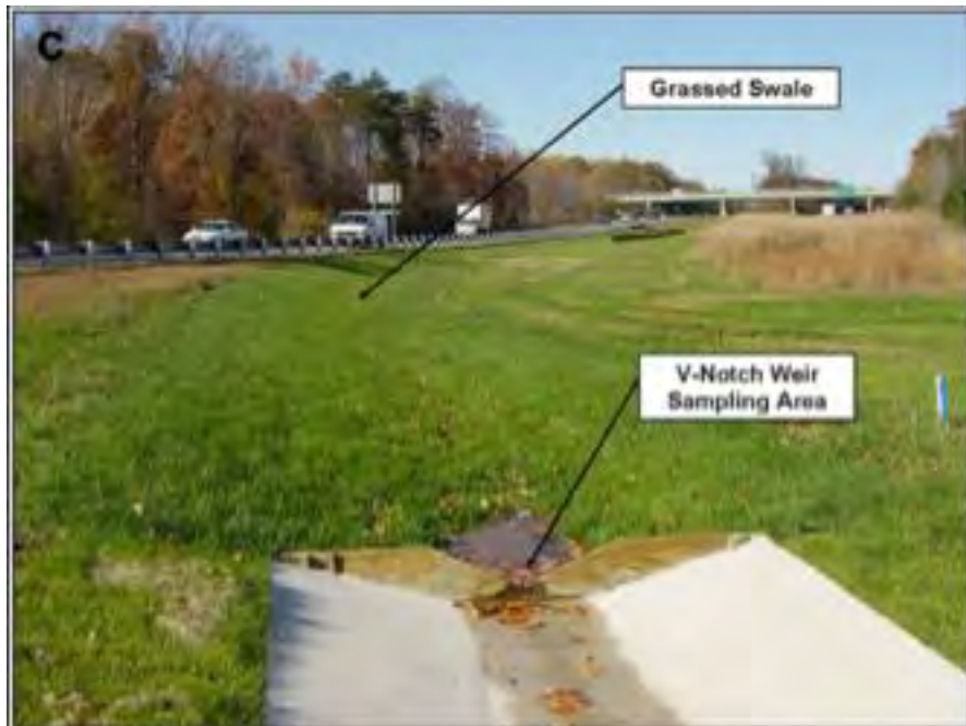
Figure. 3-6. Roadside grassed swale in Savage, MD Source: Davis et al. (2012)
