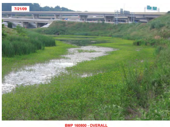
Figure 2-5 – SWM Facility 160800 After Construction
