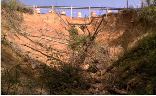
Figure 1-23: MD 210 Outfall Stabilization Before Construction
