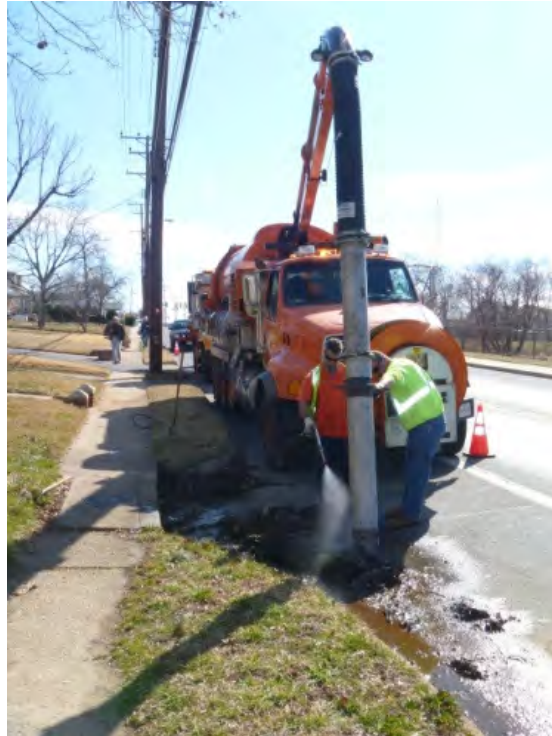
Figure 1-16: SHA Shop Personnel Operating Vacuum Truck to Clean Roadside Debris
