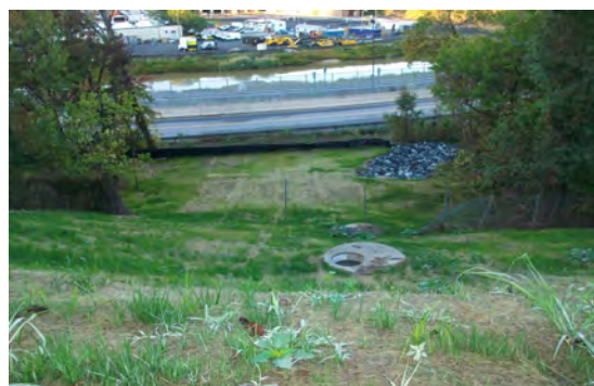
Figure 1-22: I-495 Outfall Stabilization After Construction
