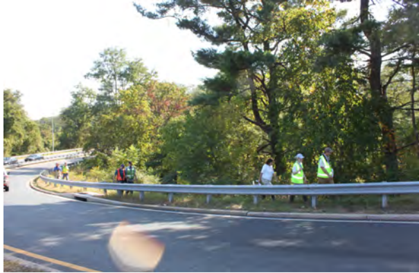
Figure 1-32: I-695 at Cromwell Bridge Minebank Run Retrofit Site
