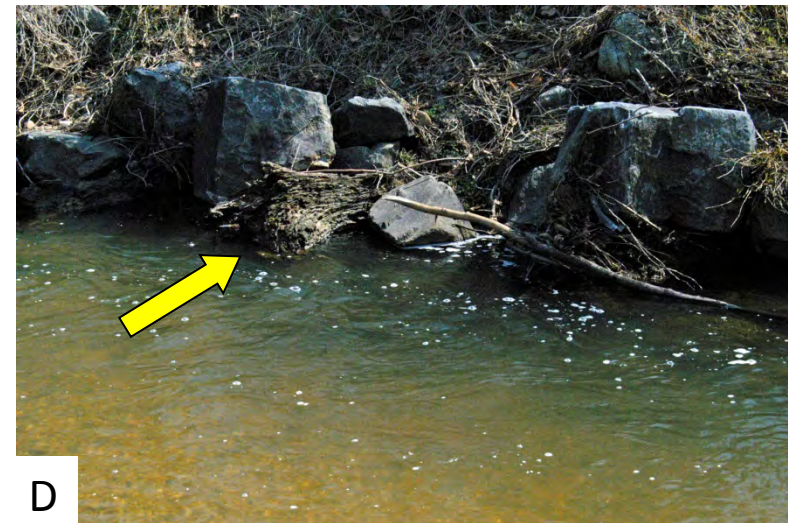
Figure LPB 2. Stream restoration structures in Little Paint Branch. A) stream bank stabilization and root wads along east side of LPB; B) upstream view of LPB near Middle Restoration site; C) cross vane – note depth of water and substrate; and D) close up of root wad showing some decomposition over time.
