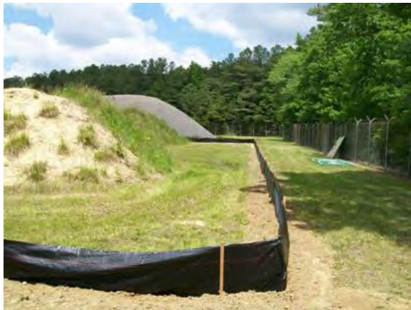
Figure 1-20: Installation of Silt Fencing around Soil Stockpile
