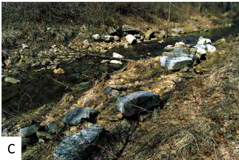
Figure PIC 2. Physical habitat of Piney Creek – A) upstream control area; B) slumping area adjacent to I-83 on the west bank of Piney Creek; C) destroyed J-vane – note downcutting of stream bed; and D) large road drainage culvert upstream of control area on Piney Creek.
