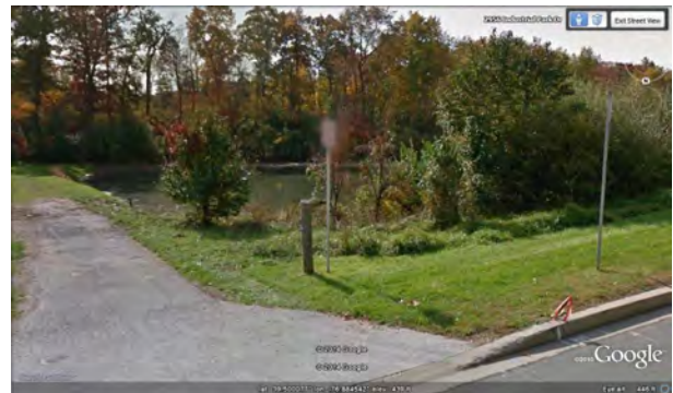
Figure 1-36: Finksburg Industrial Park Pond Retrofit Project before Construction
