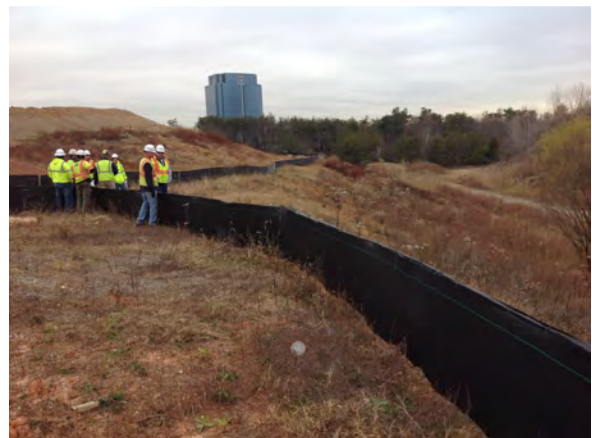
Figure 1-4: EPA Inspection of Erosion and Sediment Control Measures on a Construction Site
