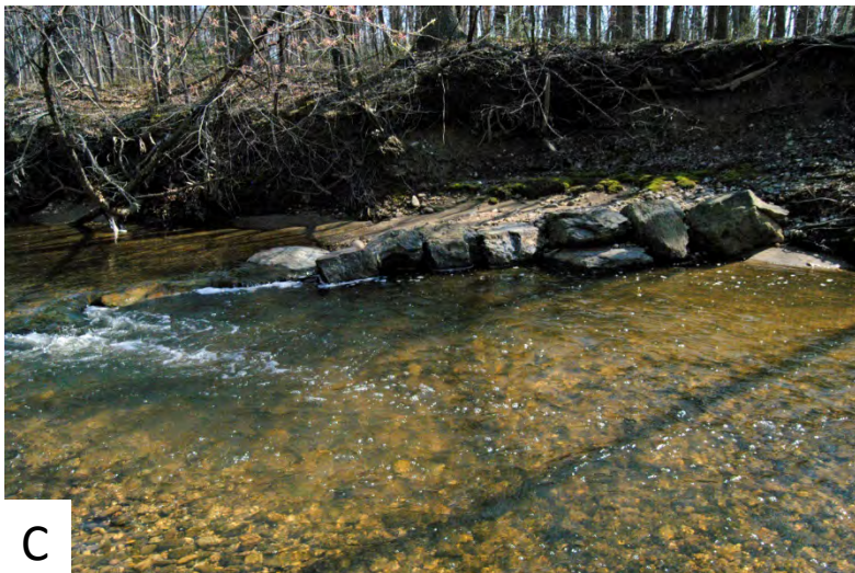
Figure LPB 2. Stream restoration structures in Little Paint Branch. A) stream bank stabilization and root wads along east side of LPB; B) upstream view of LPB near Middle Restoration site; C) cross vane – note depth of water and substrate; and D) close up of root wad showing some decomposition over time.
