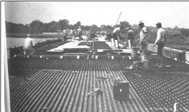
Construction photograph of the composite timber concrete bridge at Patuxent NAS published on the cover of the July 1953 issue of BuDocks Technical Digest .
