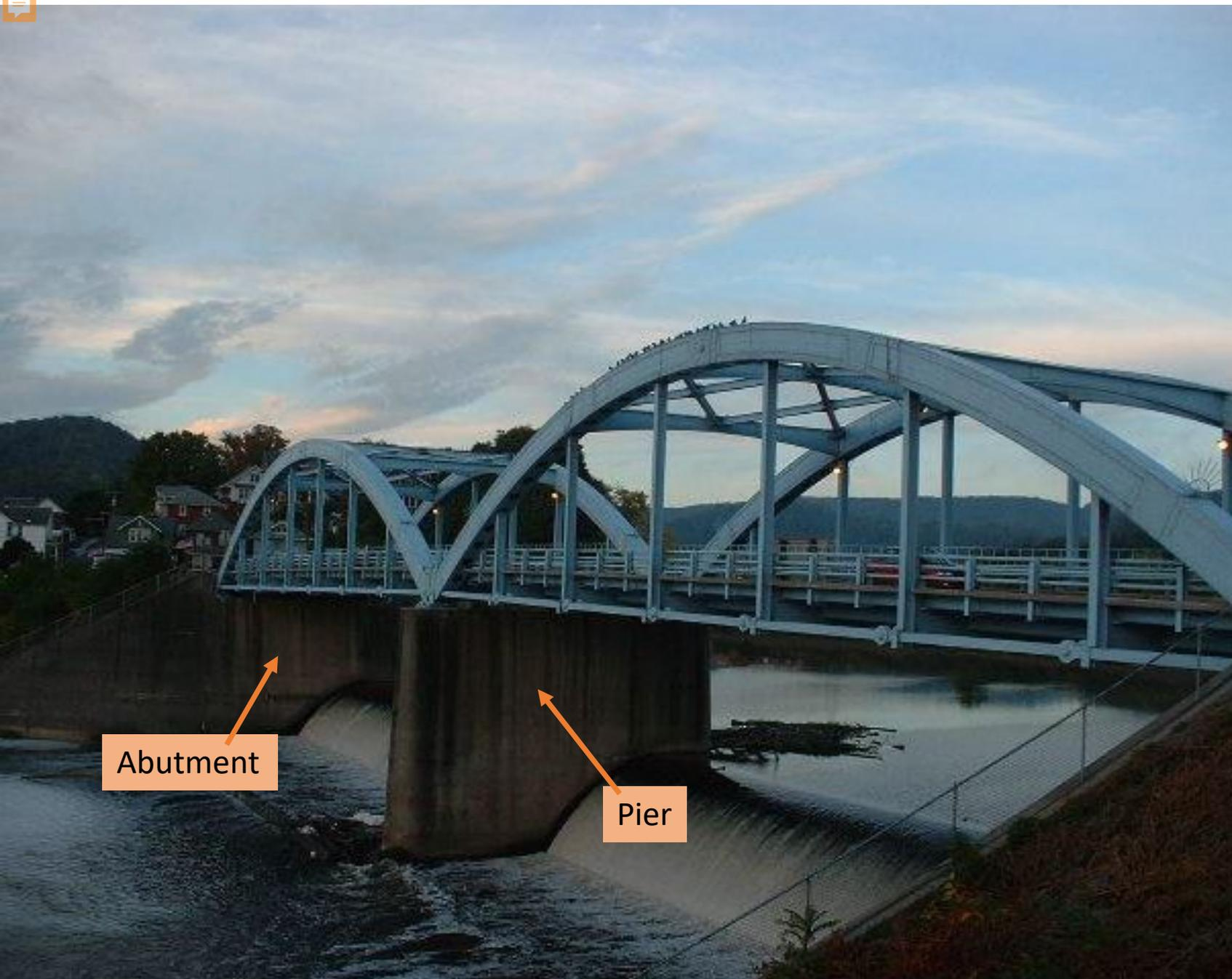
**Abutments** and **piers** are two bridge parts that are affected by a bridge's site location.
