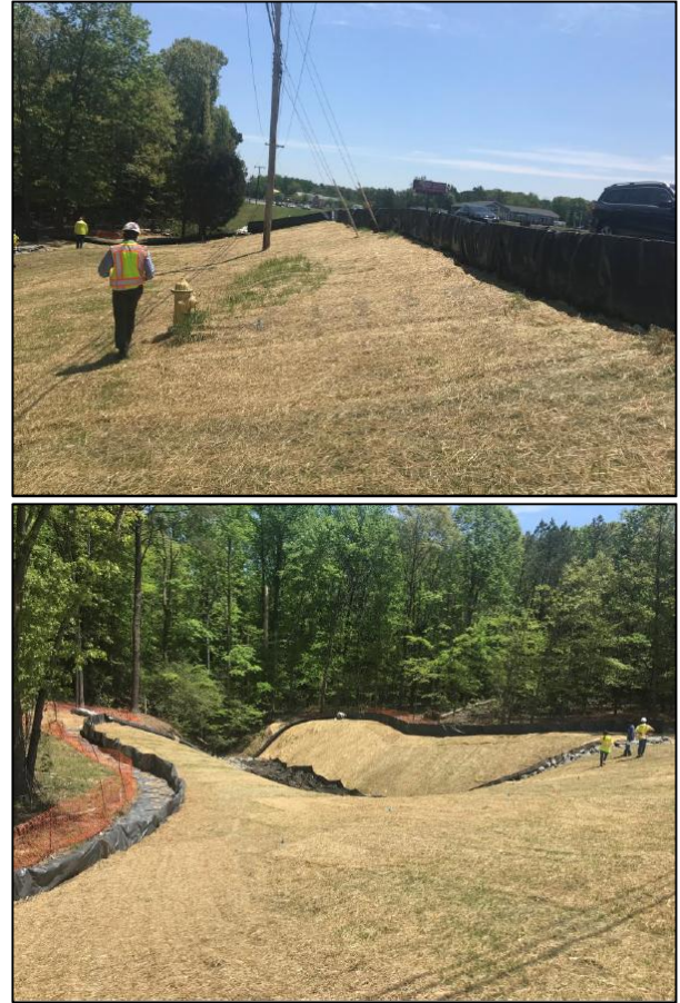
Figure 2-16: Site No.2 Near Construction Completion. Upper picture shows area stabilized (outfall failure use to be near the wooden pole) and lower picture shows the stabilized downstream channel
