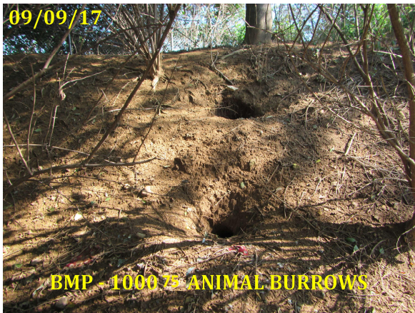
Figure 2-7: Pond Embankment Animal Holes Rated "C"
