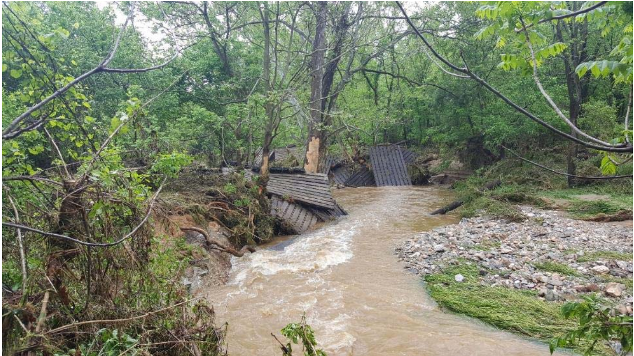
9 - Section of Little Catoclin Creek looking downstream of USGS station 01636846 showing massive timber mats used to support heavy earth-moving equipment stacked against the banks of Little Catoclin Creek.
