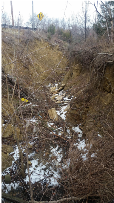
Before: Excess Erosion Threatens Roadway and Guardrail
