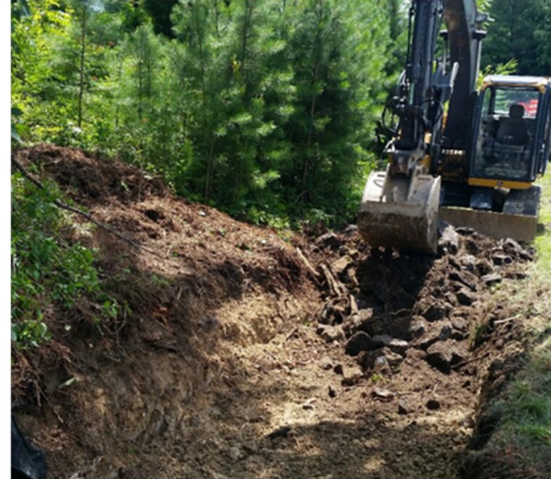
BMP 020354 Excavate Spent Material and Excess Sediment from Infiltration Trench
