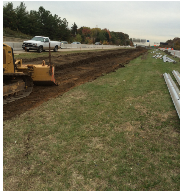
Figure 1-47: Grass Swale Upgrade along I-97
