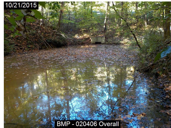
Figure 2-30: Pond Rated “VI” (Abandoned due to difficult access making routine and/or major maintenance not feasible)
