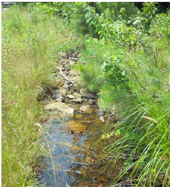
Before – Overgrowth, Standing Water & Media Replacement Needed
