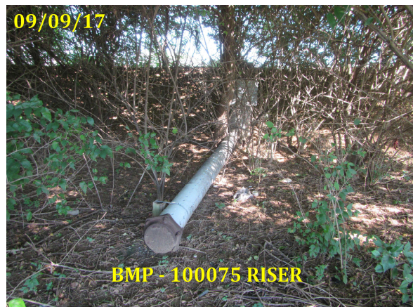
Figure 2-6: Pond Riser Rated "C"
