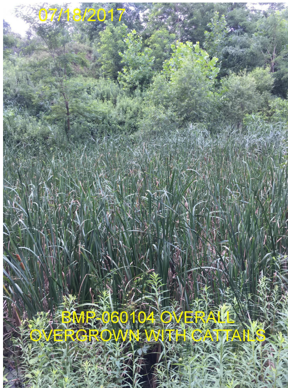
Figure 2-26: Pond Rated "III" (overgrowth of cattails, woody vegetation growth on embankment, and additional sediment removal likely needed )
