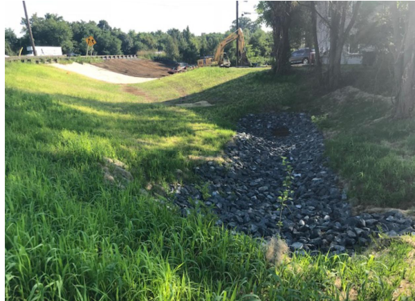
After: Stabilized Slopes, Vegetation Beginning, Rip Rap added for additional protection
