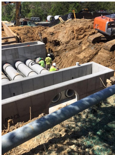
During – Installing Principle Spillway Pipes For Safe Passage of Large Storms
