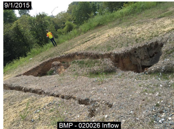
Figure 2-27: Pond Rated "IV" (excessive erosion of inflow requiring embankment rebuilding)
