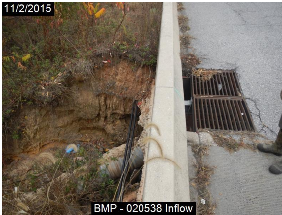
Figure 2-29: Infiltration Trench Rated “V” (severe erosion near inflow threatens roadway)
