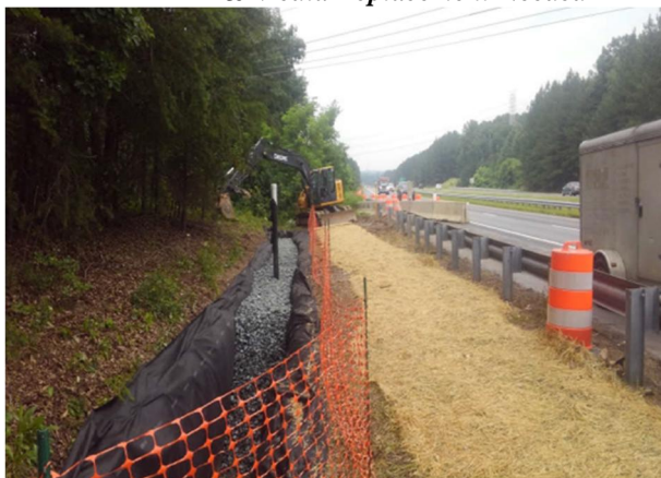
During – Remediation Activities, Stone Backfilling
