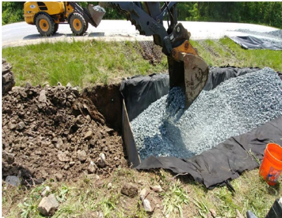
BMP 020143 Stone Backfill for Infiltration Trench
