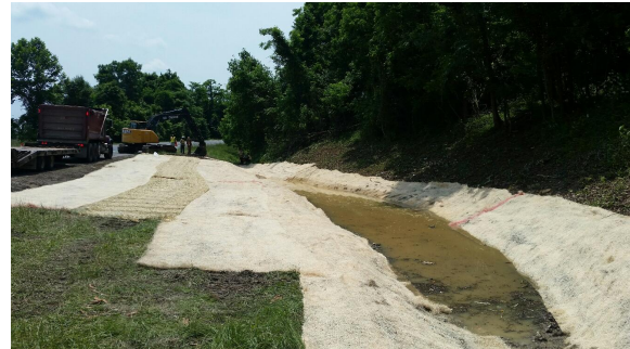
Figure 2-35: Post Remediation of Infiltration Trench – still holding water, contractor noted that with no recent rains trench held water for 3 days
