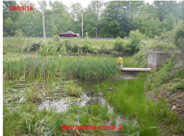
Figure 2-5: Pond and Riser Rated "B"
