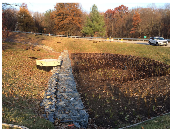
Figure 1-42: Bioretention BMP in Frederick County - Under Construction
