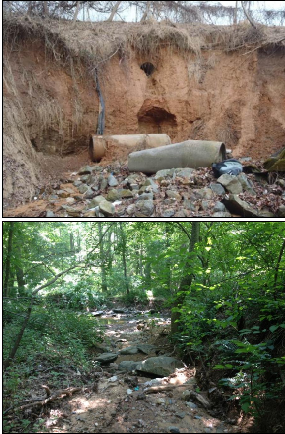
Figure 2-17: I-270 at Montrose Road Outfall Failure. Upper picture shows outfall failure and lower picture shows the sediment accumulated in the channel
