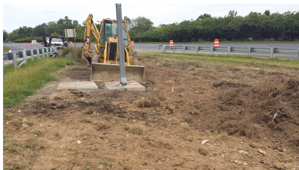
Figure 1-41: Bioretention BMP in Frederick County - Under Construction
