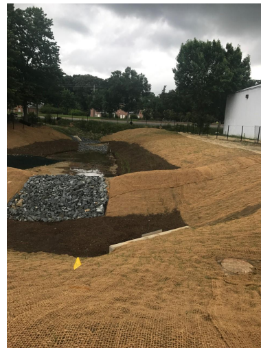
During –Installation of Matting, Stone Backfill for Forbay weir
