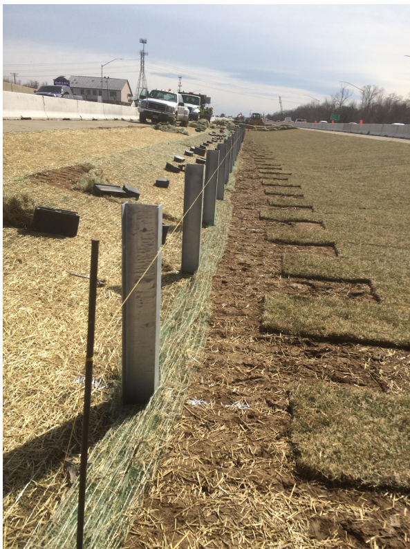
Figure 1-46: Grass Swale Upgrade along I-97
