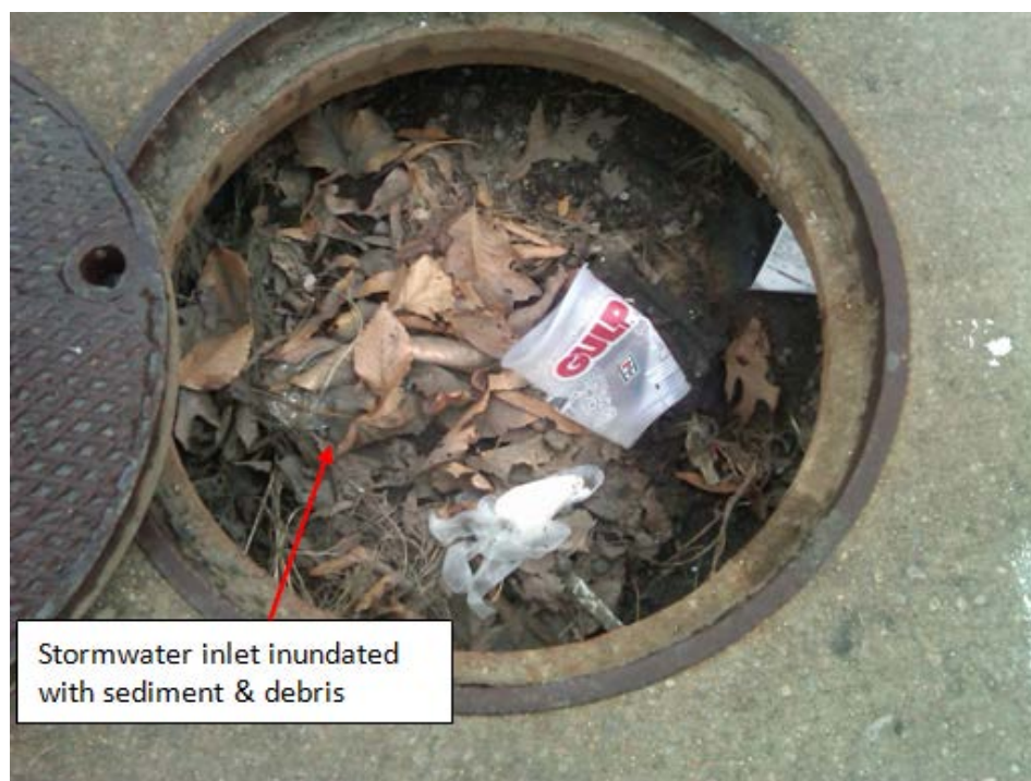
Figure 4: Stormwater inlet in front of the church on Indian Head Highway (inside manhole)
