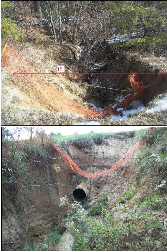
Figure 2-15: Site No.2 Outfall Failure.
