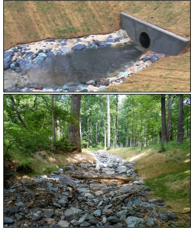
Figure 2-18: I-270 at Montrose Road Outfall Stabilization. Upper picture is of stabilized outfall at I-270 at Montrose Road. Lower picture is of restored downstream channel at I-270 at Montrose Road.
