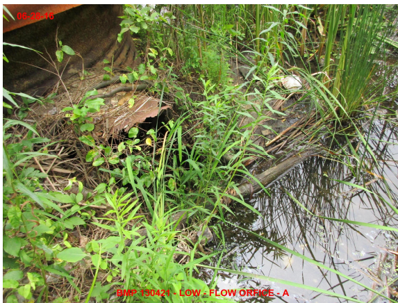
Figure 2-8: Pond Low Flow in Riser Rated "D"
