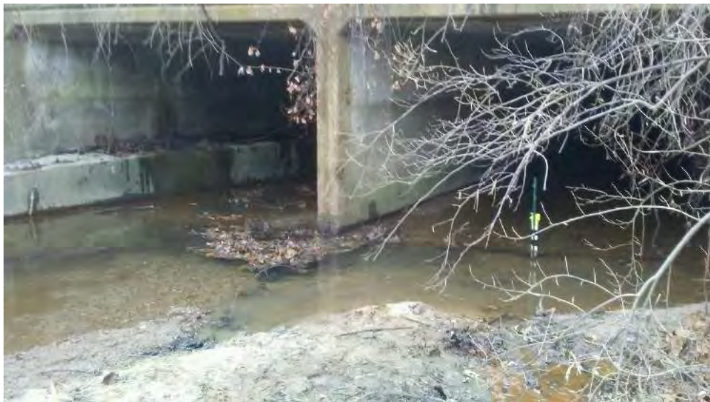
Photograph 68. 12/14/2018: After clearing of debris jam at box culvert for Flow Station 1
