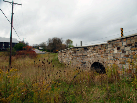
Work on the Little Meadows Bridge along the Historic National Road
