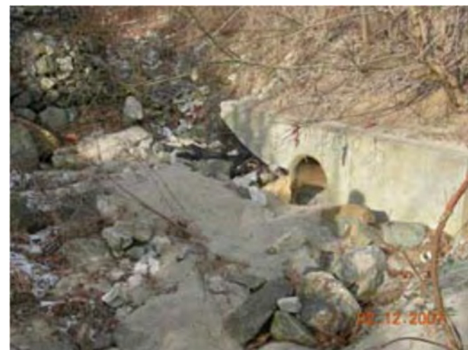
Major Sediment Accumulation at Outfall
