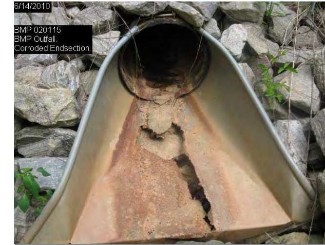
Deteriorated CMP End Structure
