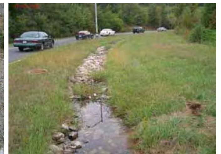
Saturated Infiltration Trench
