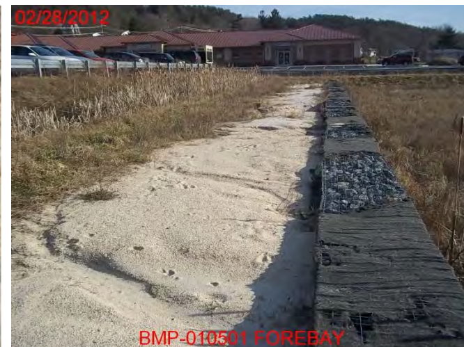
Major Sediment Accumulation in Forebay
