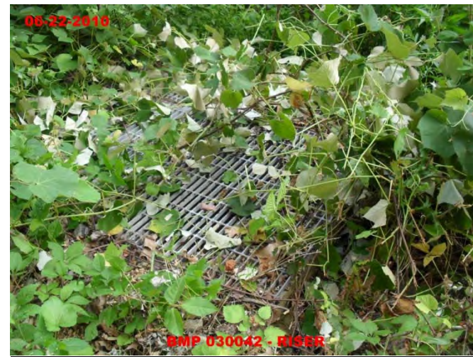
Vegetation Obstructing Outflow Point
