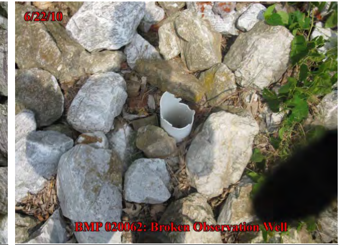
Broken Observation Well
