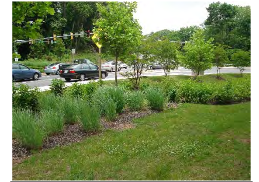
Example Filtration Facility
