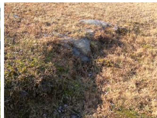
Frozen Seepage Through Embankment
