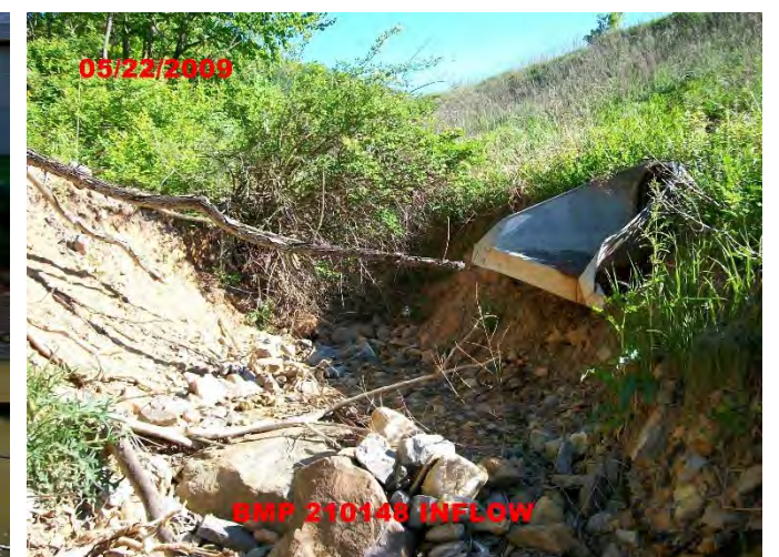
Major Erosion at Inflow Point
