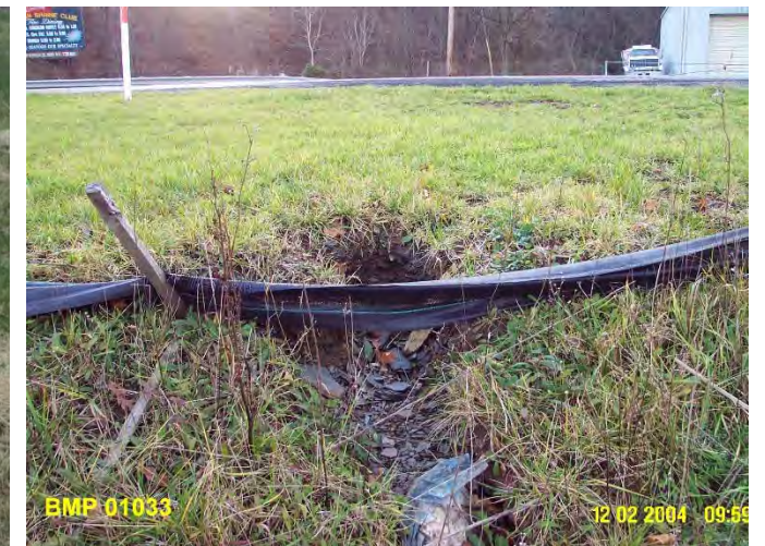
Minor Erosion Under Silt Fence
