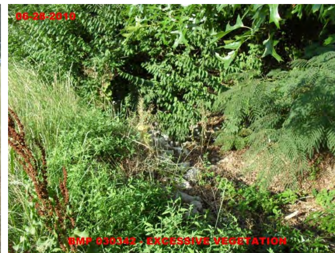
Excessive Vegetation in Infiltration Trench
