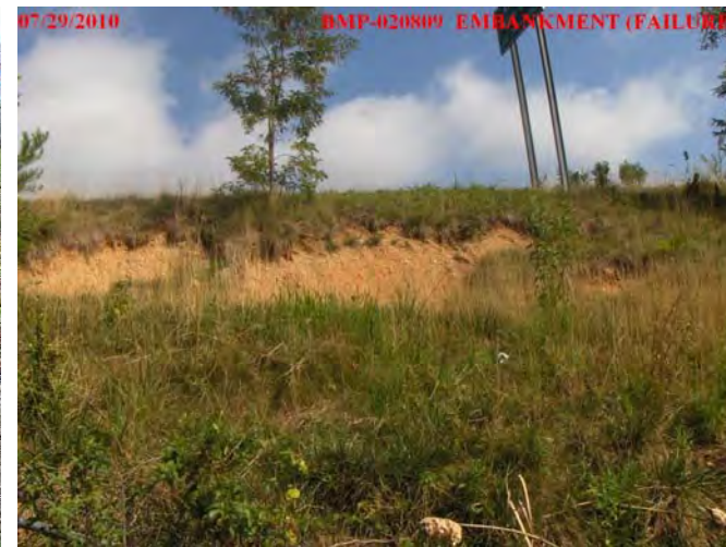
Eroded Embankment
