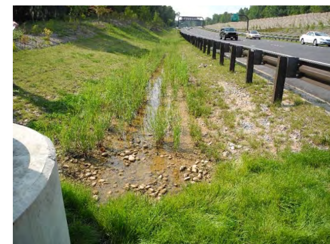
Ponding Water in Bio-Swale
