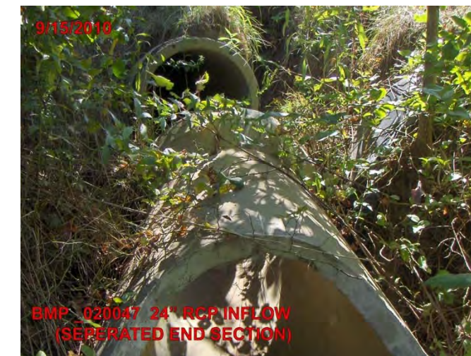
Pipe Separated From End Structure
