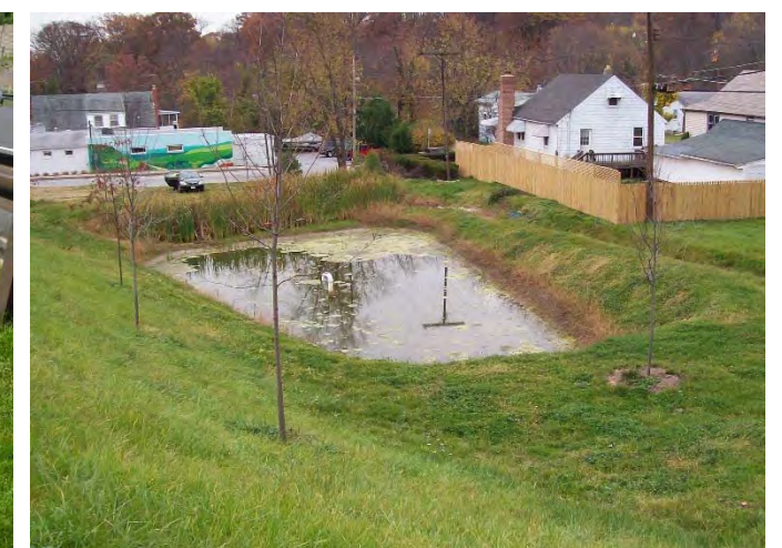
Surface Sand Filter Not Draining
