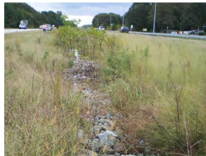
Excessive Vegetation in Infiltration Trench
