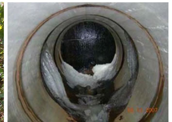
Water Leaking into Pipe
