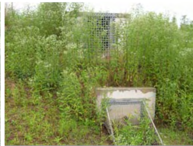
Vegetation Obstructing Riser Structure
