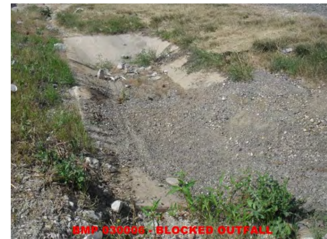
Accumulated Sediment Blocking Outflow Point
