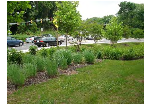
Example Filtration Facility
