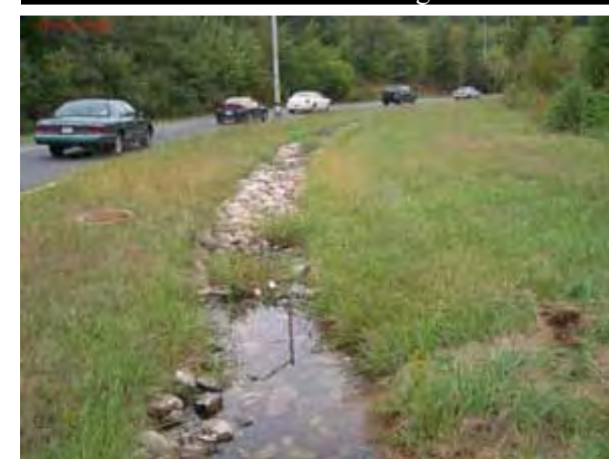
Saturated Infiltration Trench
