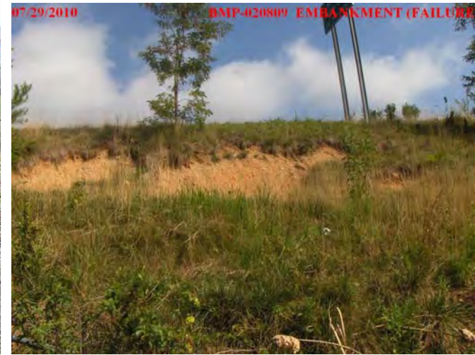
Eroded Embankment
