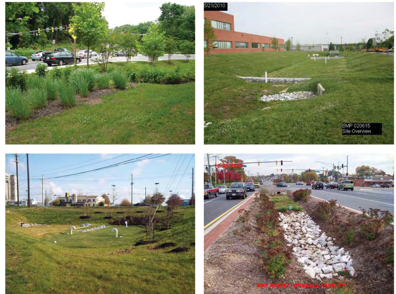
SAMPLE FILTRATION FACILITY PHOTOS
