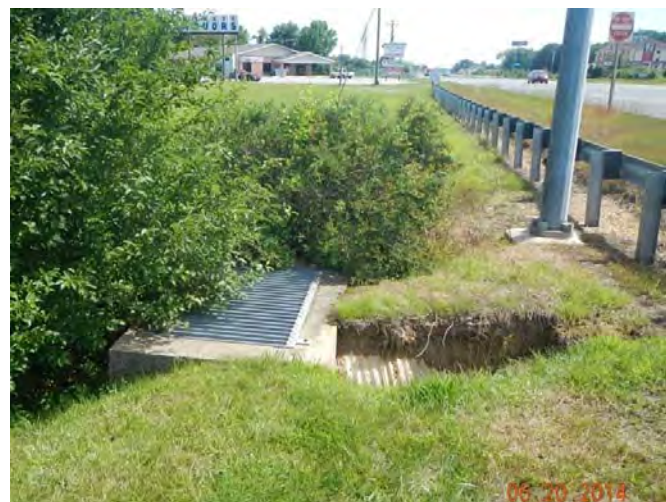
Eroded Embankment Exposing Pipe
