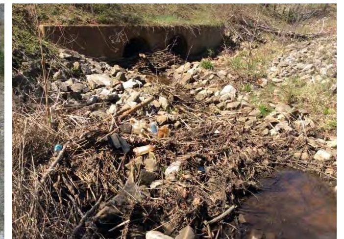
Accumulated Debris Blocking Outflow Point
