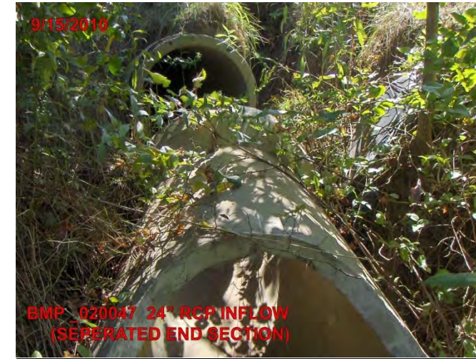
End Structure Separated From Pipe
