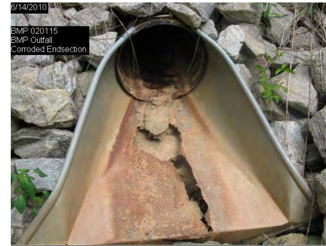
Deteriorated CMP End Structure
