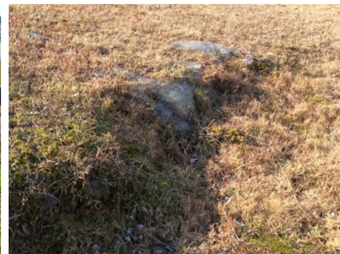
Frozen Seepage Through Embankment
