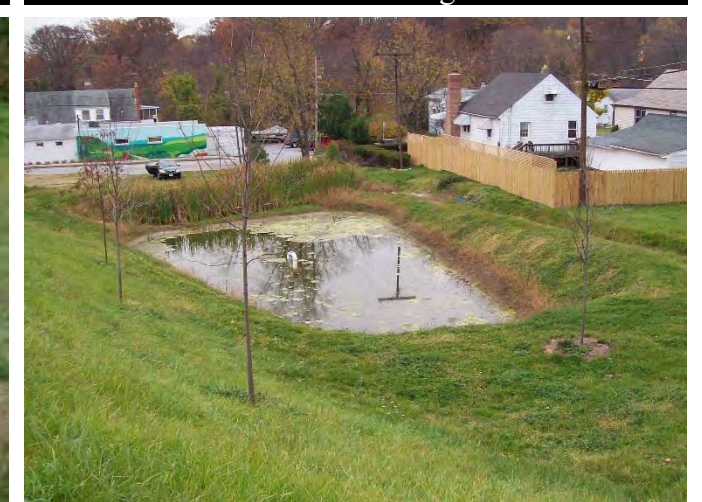
Surface Sand Filter Not Draining
