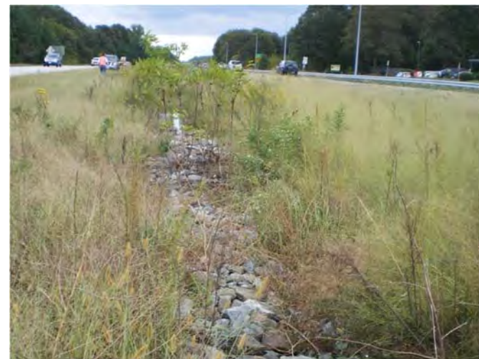
Excessive Vegetation in Infiltration Trench
